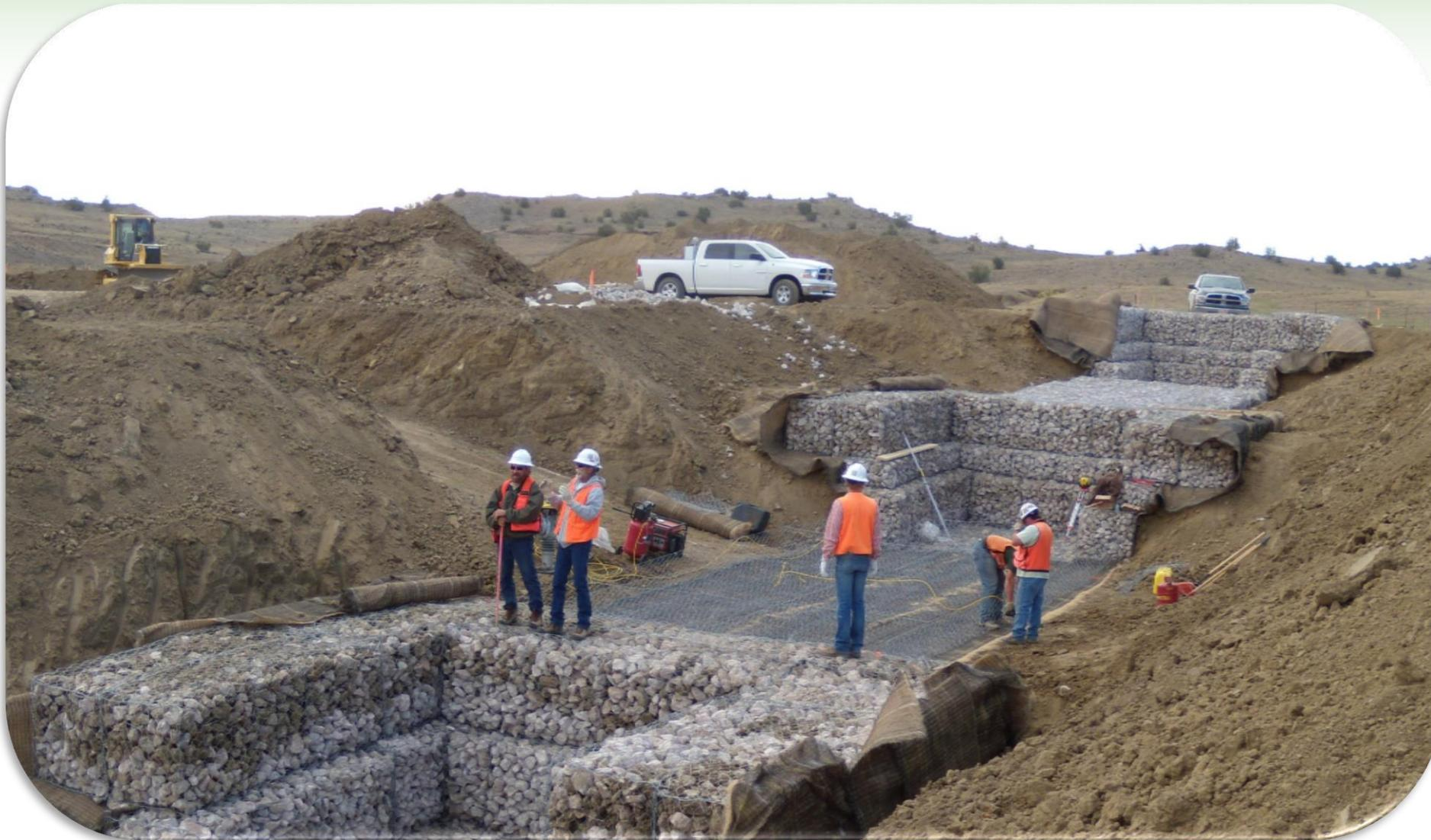
Installation of Rock Erosion Barriers at L-Bar, New Mexico
