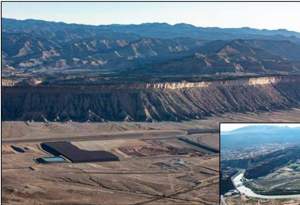
Crescent Junction, Utah, Disposal Cell Site (2018).
