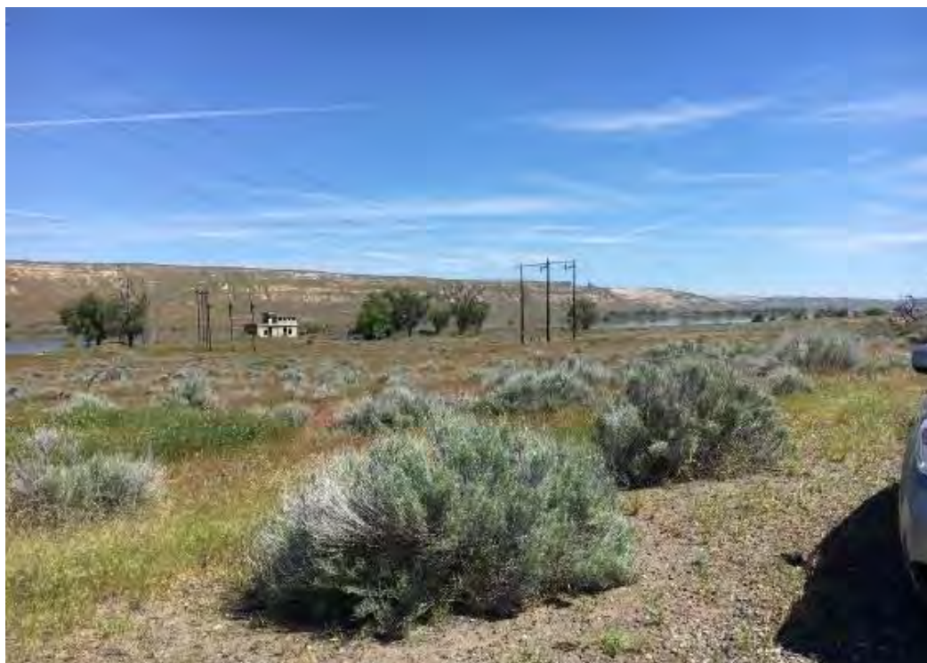
Figure 3-16. View from Gravel Road Near Solar-Powered Siren Facing Pole/Structures 24/1, 24/2, and 24/3
