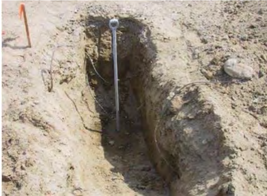
Figure 2-6. Plate Anchor Hole and Anchor Rod
