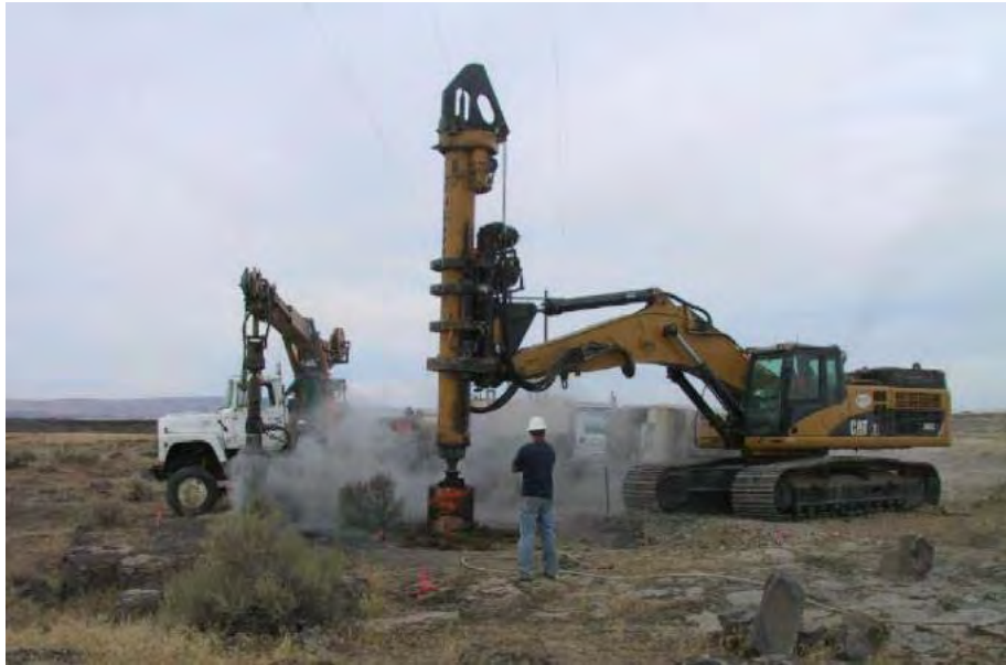
Figure 2-5. Pole Hole Excavation
