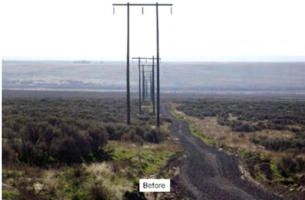
Figure 2-1. Transmission Line North of Project Limits (Before)
