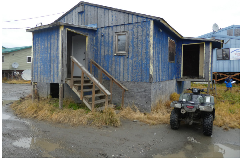
The TANF office could reduce energy costs by replacing supplementary electric heaters with another Toyotomi stove.
