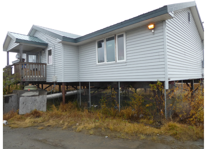
The daycare building frequently experienced overheating at the time of the building surveys.
