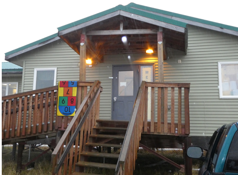
The head start building is relatively new but could benefit from lighting upgrade and setback thermostats.
