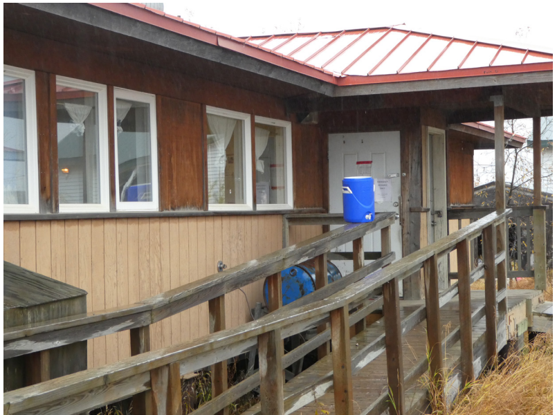
The top recommendation for the clinic, to repair and maintain zone valves in the heat distribution system, would save over $1,000 per year.
