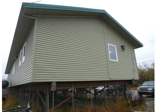
The monthly maintenance check should include a walk-around of the building exterior.
