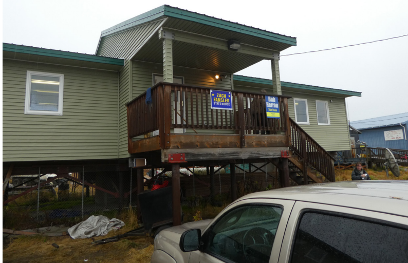
Energy retrofits for the Tribal I.R.A. building have a short payback, of approximately 2 years, if each recommendation is implemented.
