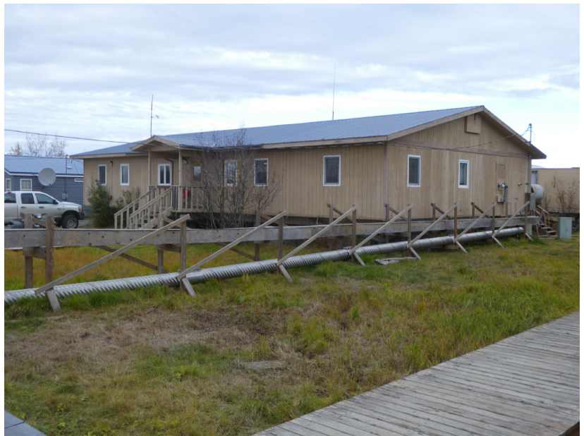
The number one retrofit for the school office is to implement a setback temperature.
