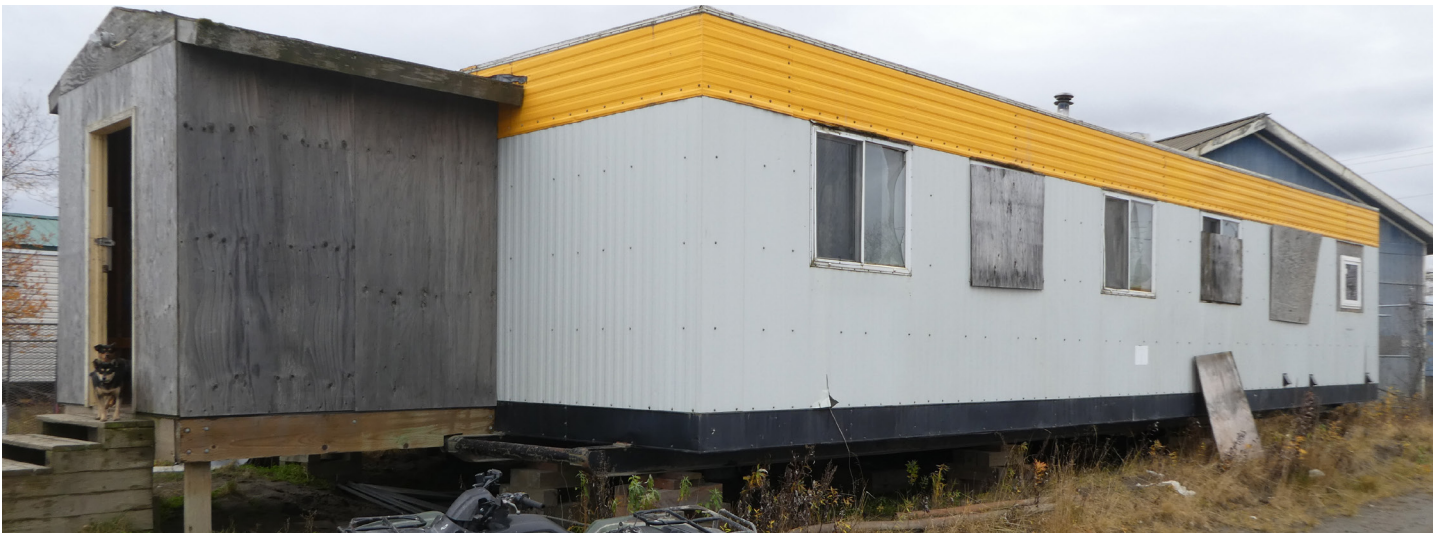
The laundry building is composed of three shipping containers from a former construction housing camp.
