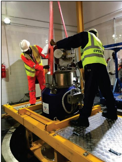
**Figure 1-3. Technical experts from Nigeria's Centre for Energy Research and Training stand over the miniature neutron source reactor and prepare to load the HEU reactor core into an interim cask.**
