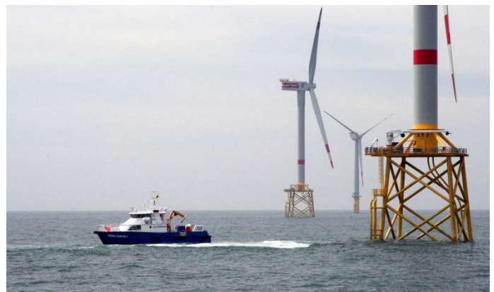
Alpha Ventus showing jacket structures in foreground, monopile in the background. Image by Gary Norton, NREL 27363
