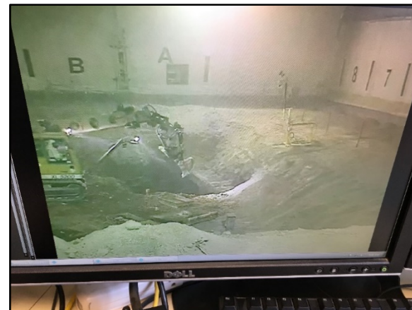
Exhuming targeted buried waste at ARP IX
