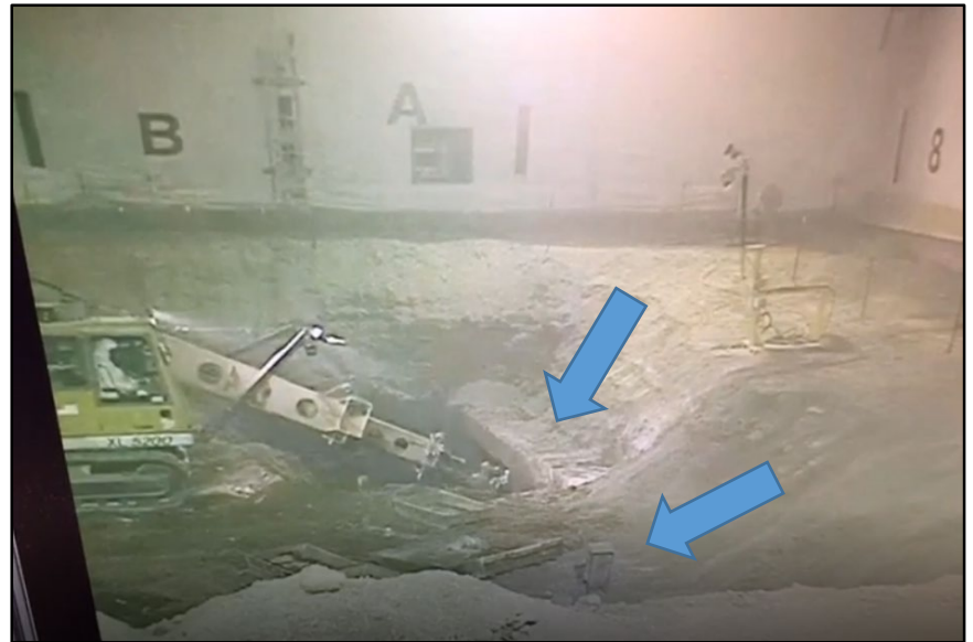
Looking south along west end of ARP IX. Arrows point to exhuming waste from under concrete duct bank and to capped H-pile.
