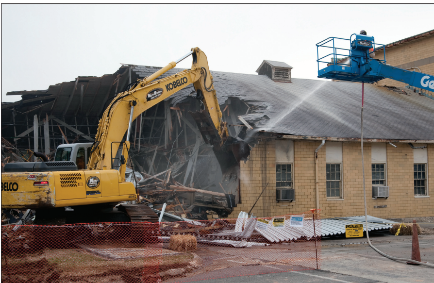
Building 9735 has been demolished
