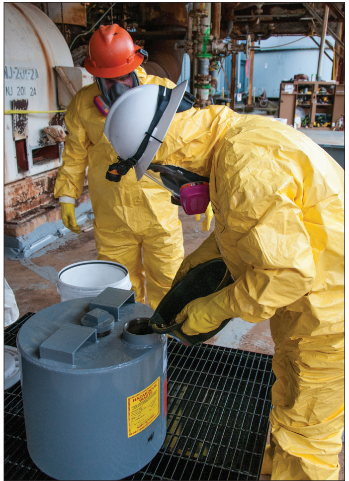
Mercury collected from the COLEX equipment is being poured into a container.
