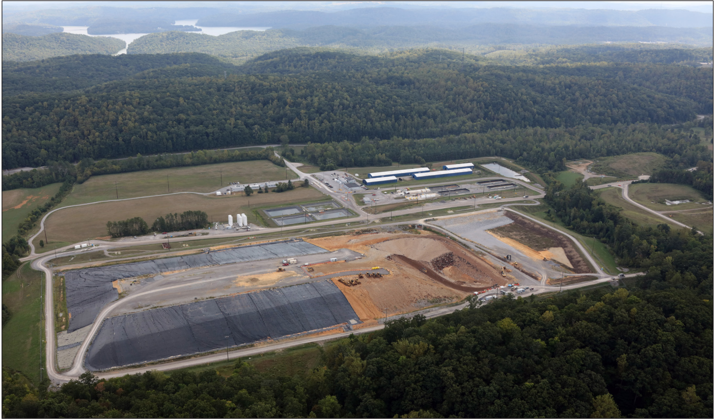
Environmental Management Waste Management Facility
