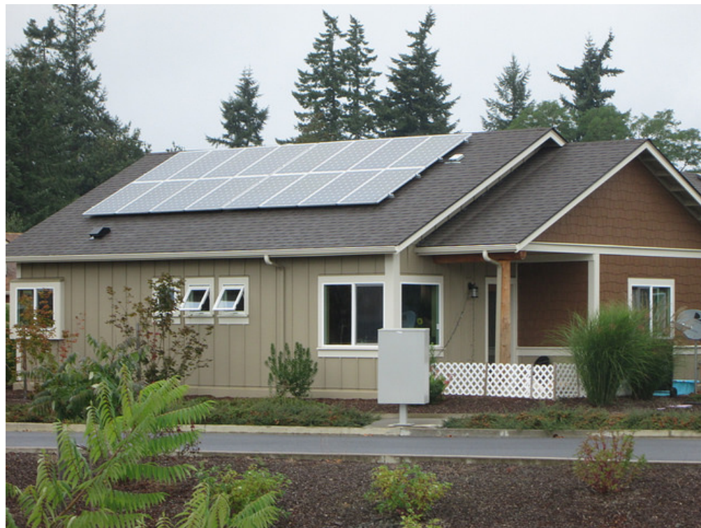
Solar PV arrays installed at a low-income housing complex for tribal elders in the Confederated Tribes of the Grand Ronde Community of Oregon. Photo from the Grand Ronde Tribal Housing Authority
