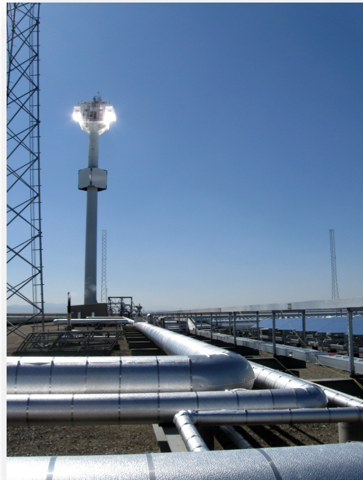
eSolar Sierra SunTower power tower plant in California. Photo by David Hicks, NREL 18397
