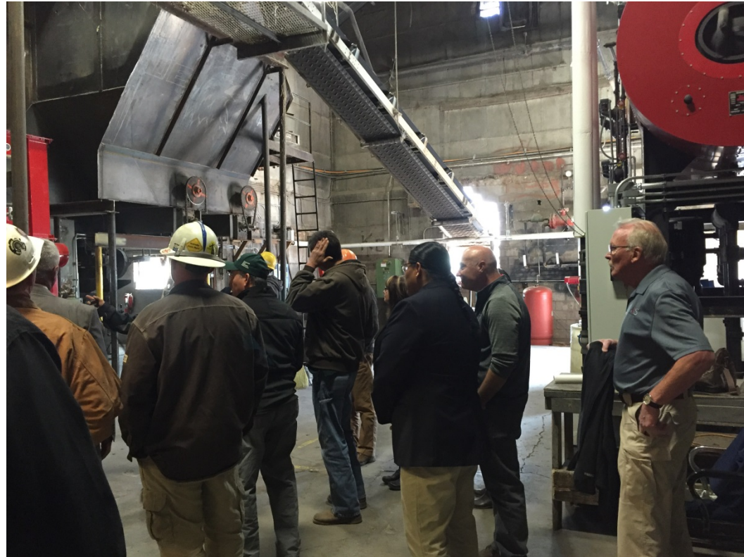
The Menominee Tribal Enterprises biomass combined heat and power district energy plant in Wisconsin. Photo from Menominee Tribal Enterprises.
