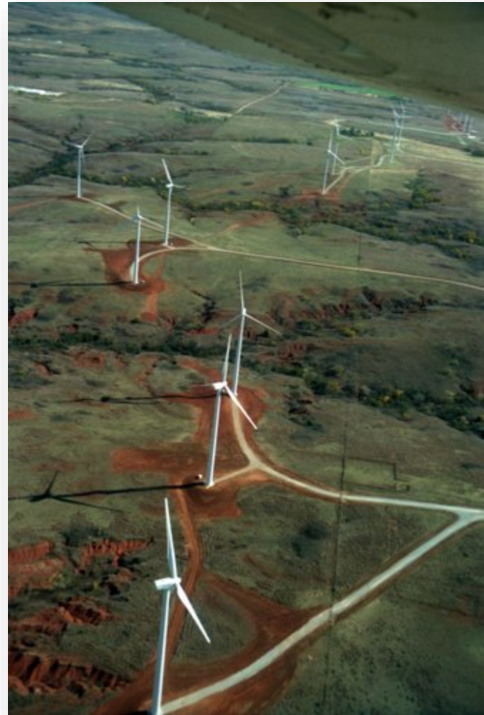
Red Hills Wind Farm in Oklahoma. Photo by Todd Spink, NREL 16509
