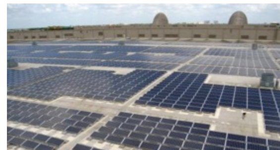
Orange County Convention Center, NREL 18077
