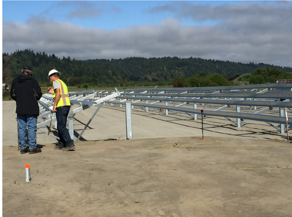
Workers installing the racking for the Blue Lake Rancheria's 500-kW solar system in California. Photo from Blue Lake Rancheria
