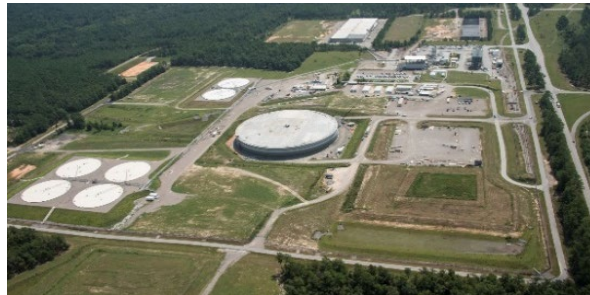
Savannah River Site
