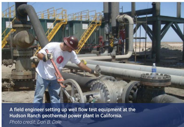
A field engineer setting up well flow test equipment at the Hudson Ranch geothermal power plant in California.
