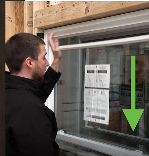
Sash sliding down under its own weight (balance not engaged)
