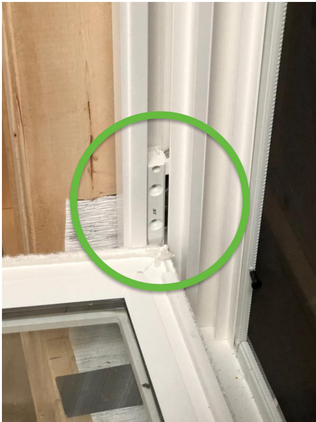
Normal—sash connected to window balance
