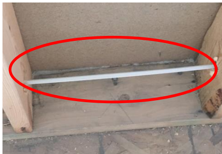
Bottom plate/sheathing gap
