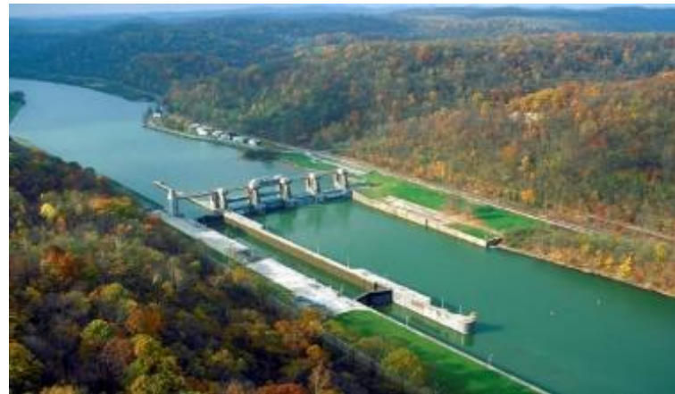
Non-Powered Dams and Conduits
