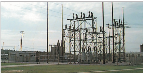
C. Primary Substation
