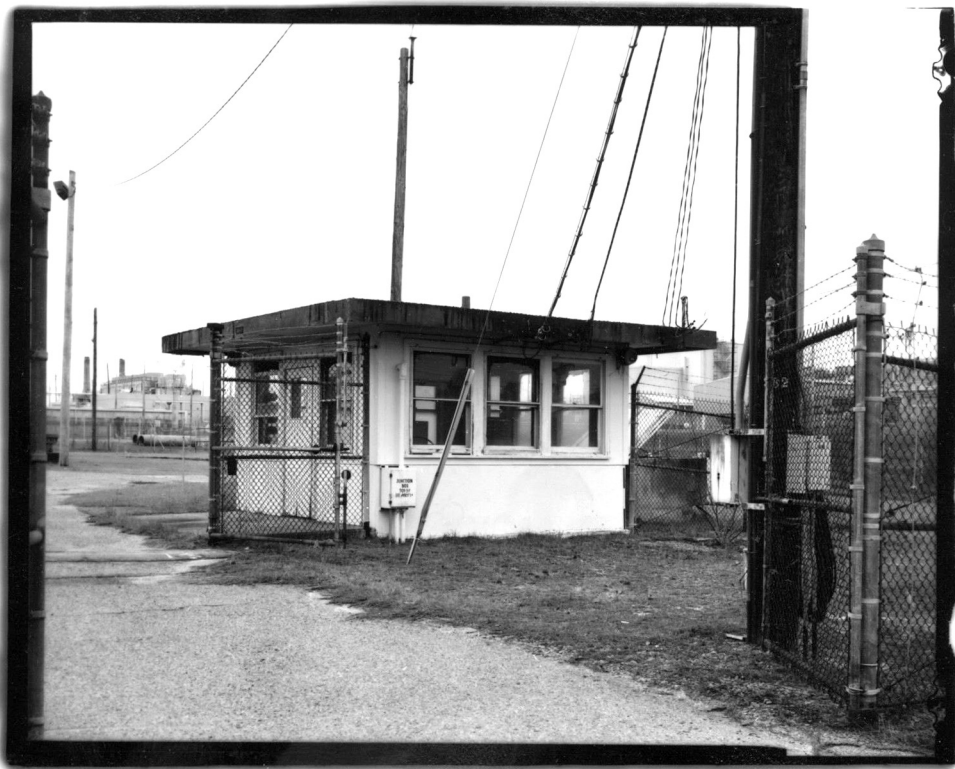
Figure 6 Example of HAER Photography, Building 701-5F, Guardhouse
