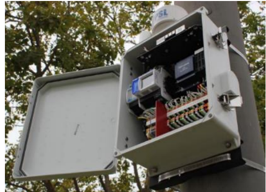
A \mu PMU installation on a utility distribution pole. There is a GPS antenna on top of box and a high resolution power quality monitor.
