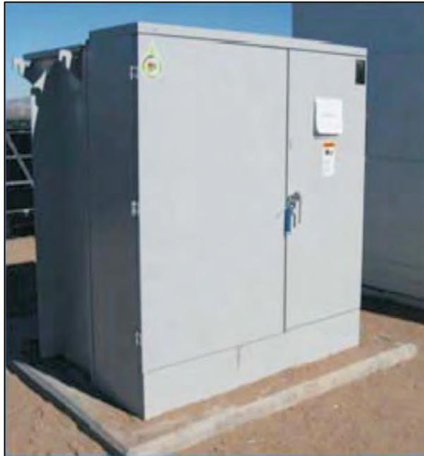
The PVCS would collect the power from between four and thirty arrays, depending upon the final site layout, for transmission to the Project substation. The switchgear cabinets, depicted below, would be approximately 12 feet high and would be situated on concrete pads dispersed among the arrays.
