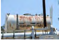
TCE (trichloroethylene) tank in Area I of SSFL – Photo by William Preston Bowling
