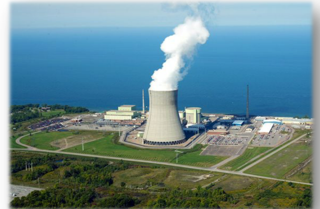
Nine Mile Point ~ Courtesy Exelon
