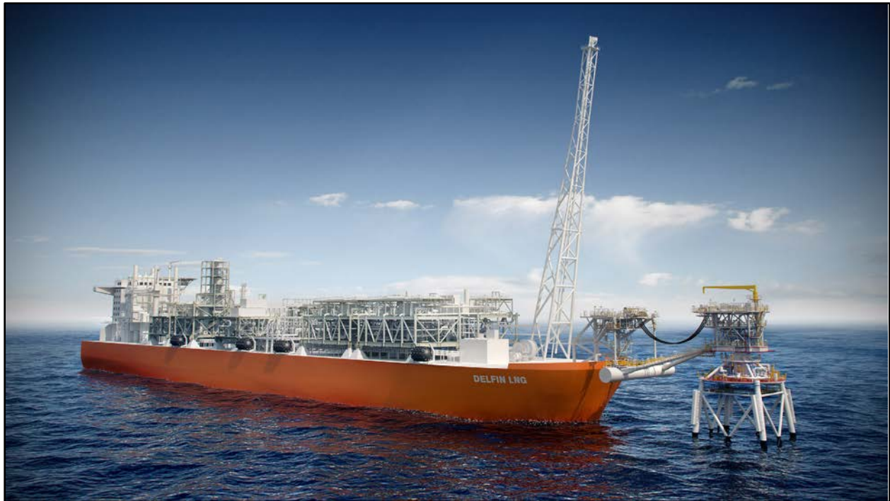
Figure 2.2-2. Floating Liquefied Natural Gas Vessel on a Tower Yoke Mooring System
