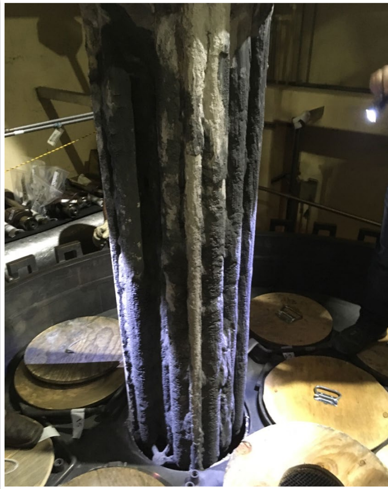
PGF Bundle being removed from housing
