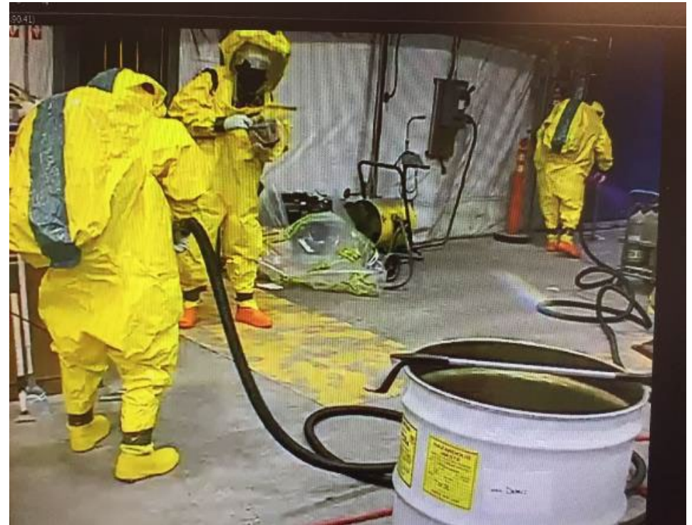
Crews used specialized vacuums early in the cleanup process to remove contaminants from the floor within ARP V
