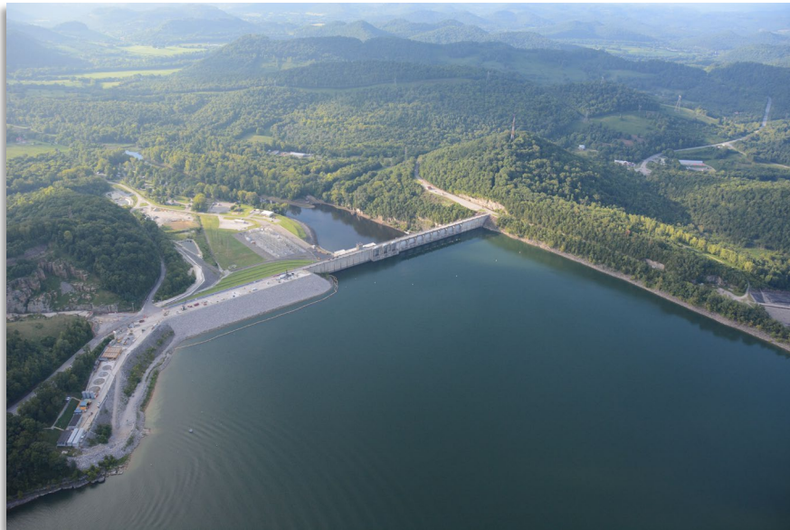
Center Hill Dam Safety - 26 Sep 2018
