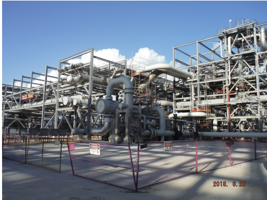
Train 5 – Feed Gas Heater turned over to Startup
