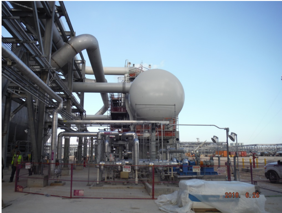
OSBL – Wet Gas Flare Knock Out Drum turned over to Startup
