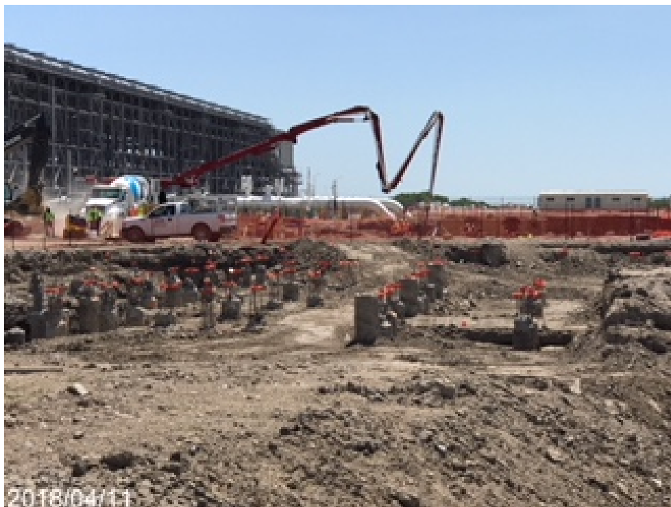
Third meter - Excavation at meter station
