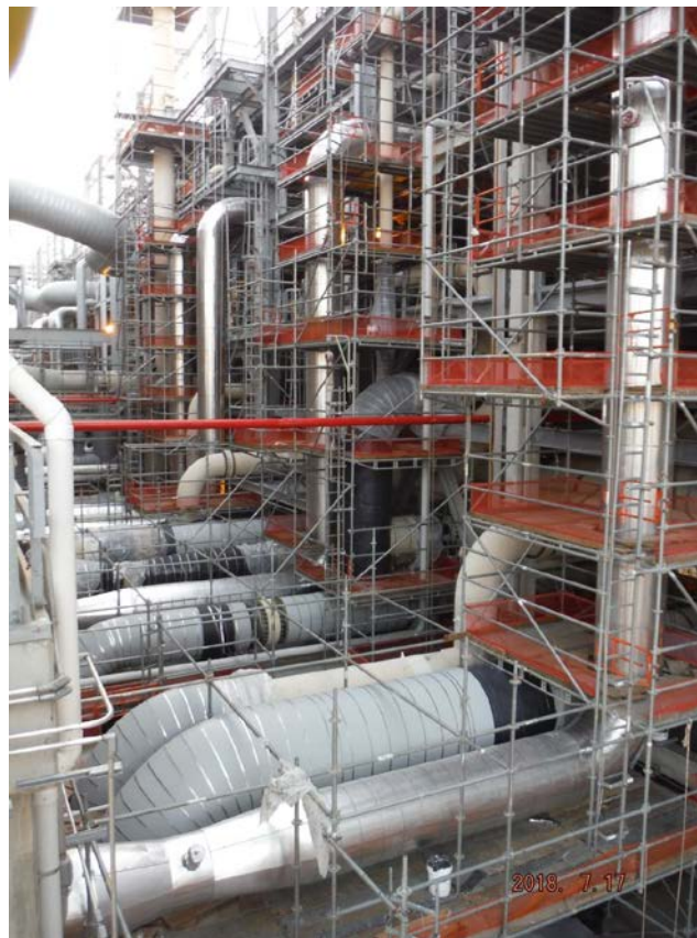
Train 5 – Alleyway Pipe Progress
