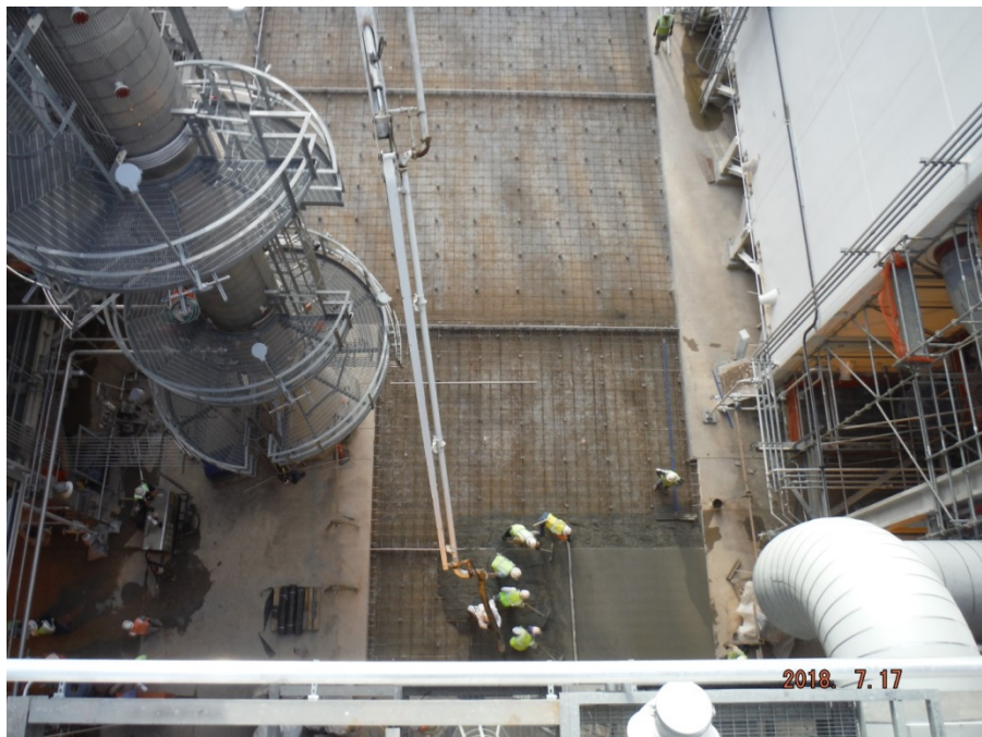
Train 5 – Paving works underway in Heavies Removal Area
