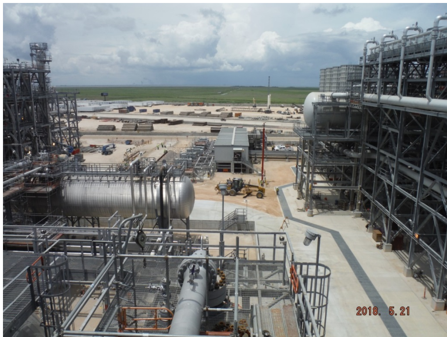
Train 5 – Area Paving Progress
