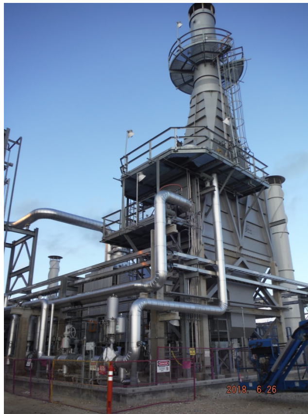
Train 5 – Thermal Oxidizer turned over to Startup
