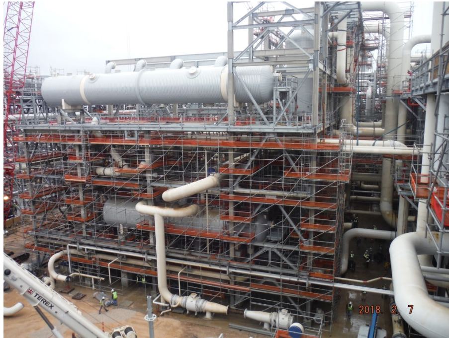
Train 5 – Piping Progress at Propane Refrigeration Area
