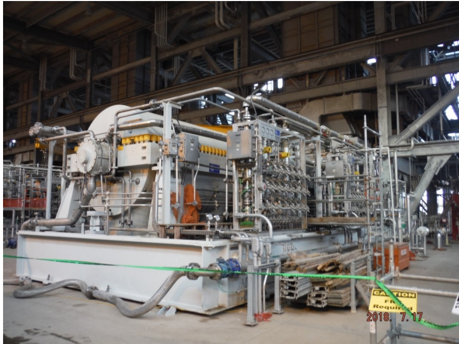
Train 5 – Compressor 1421 Post Mechanical Runs Complete
