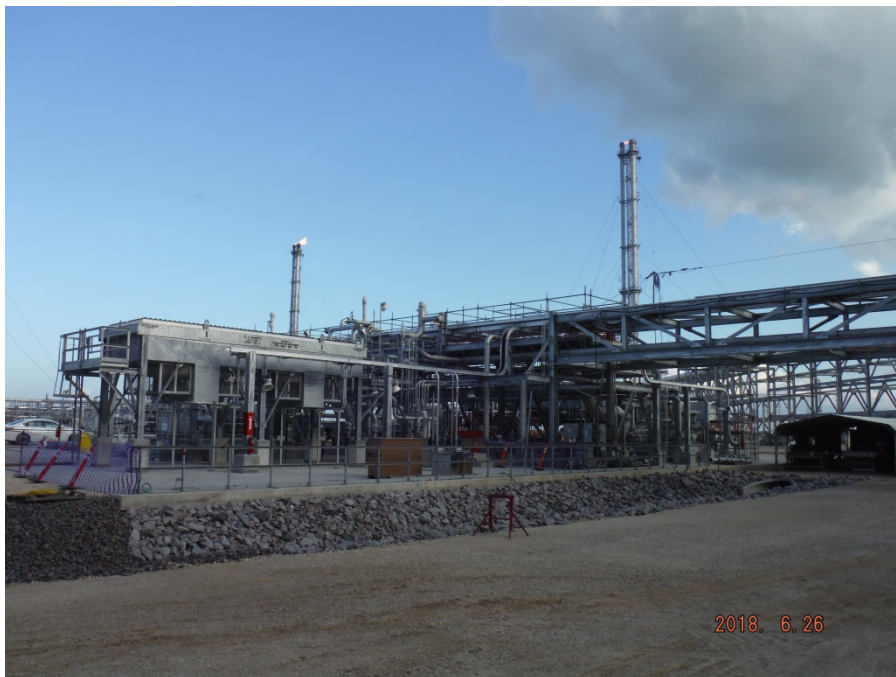
OSBL – Flare Air Assist Compressor Cooling Fans turned over to Startup
