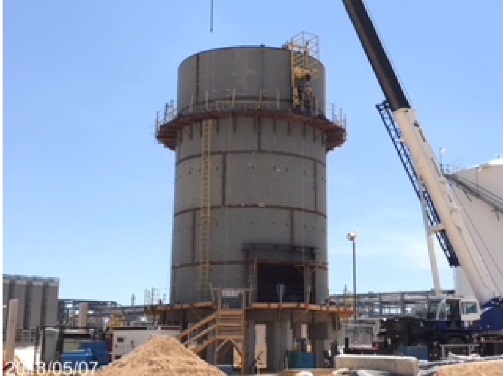
OSBL – Condensate Tank (CP13-2-000)
