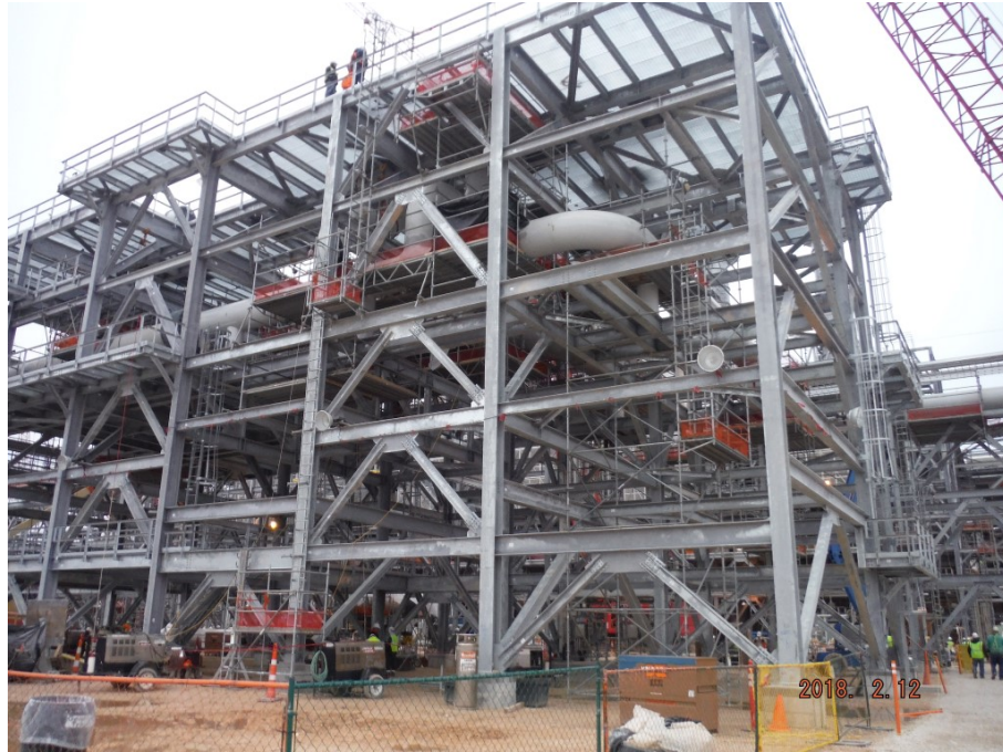
OSBL – Valve Platform Structure with Pipe Installation
