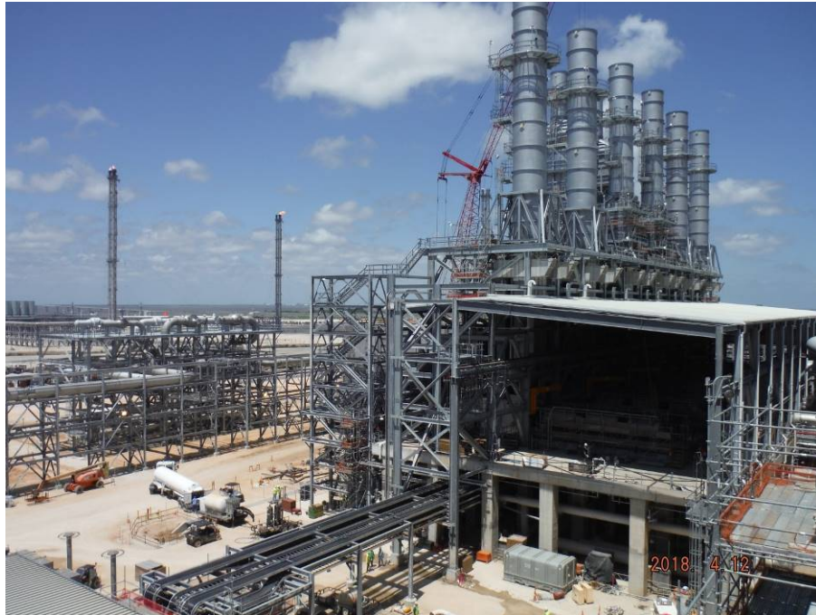
Train 5 – Construction of the Compressor Deck
