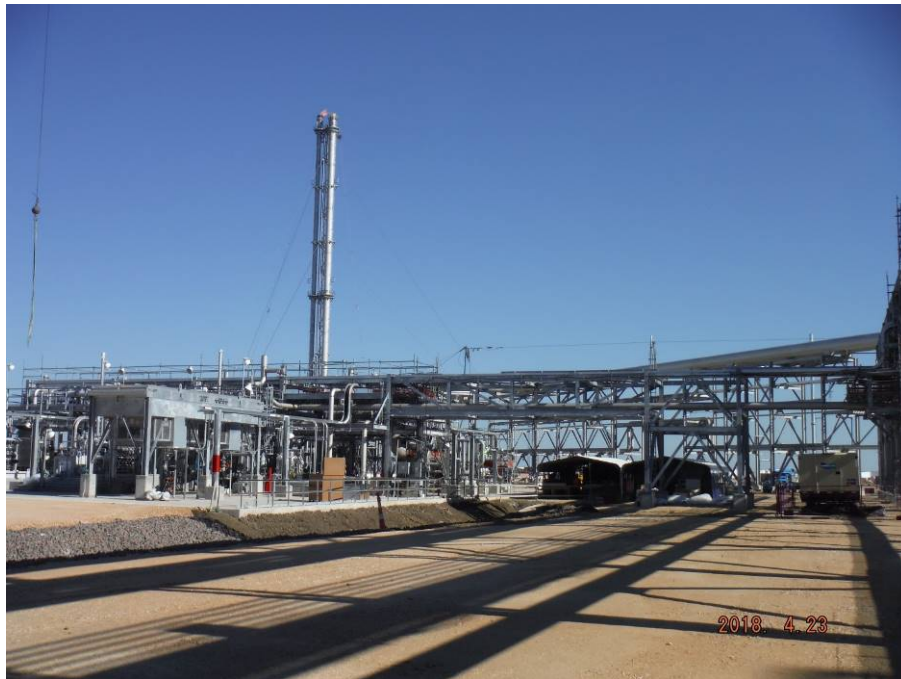
OSBL – Flare Air Compressor Area
