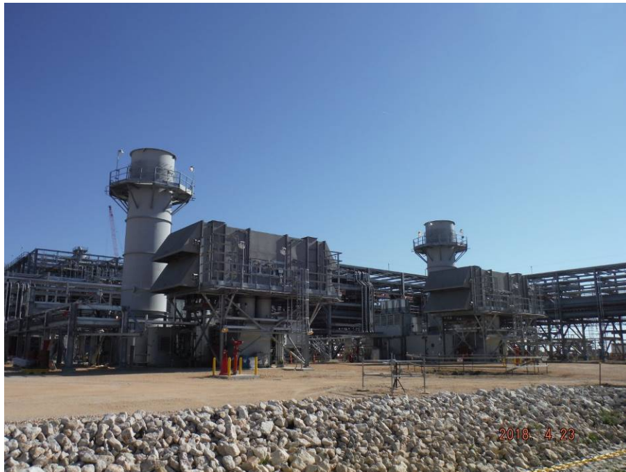
OSBL – Gas Turbine Generator Area
