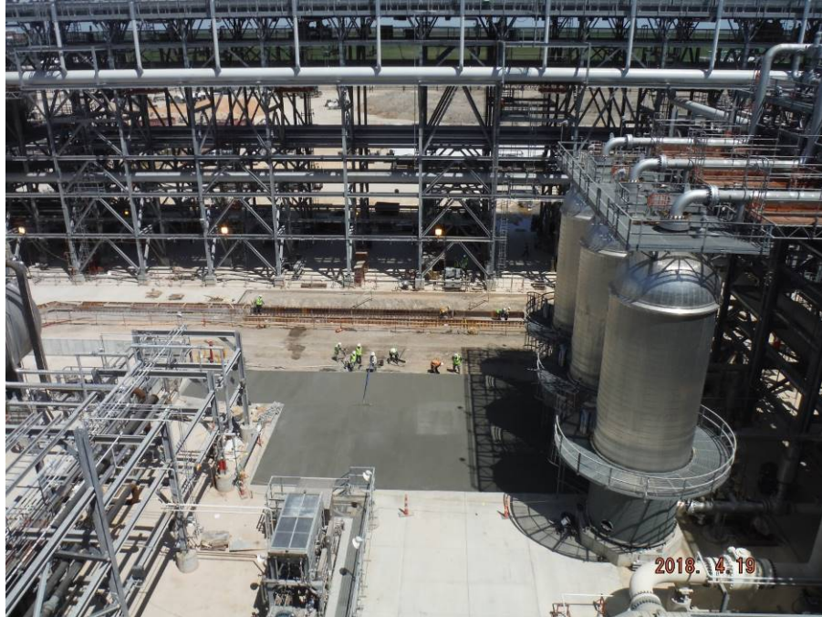
Train 5 – Area Paving
