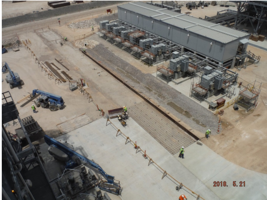
Train 5 – Area Paving and A02 Progress
