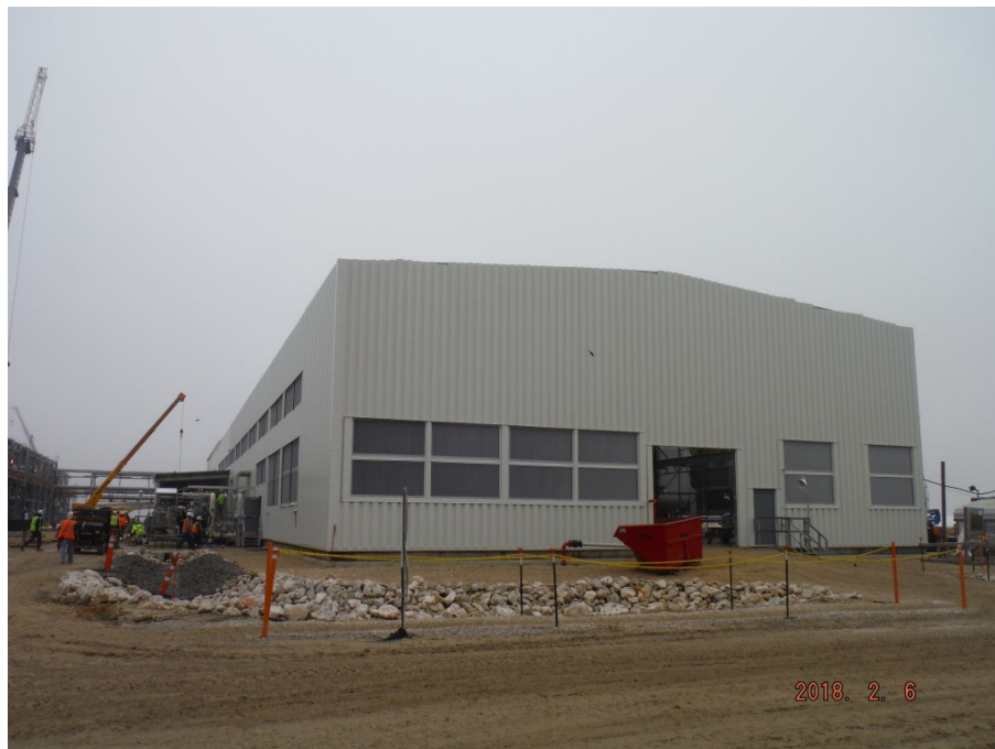
OSBL – Water Treatment Building Progress
