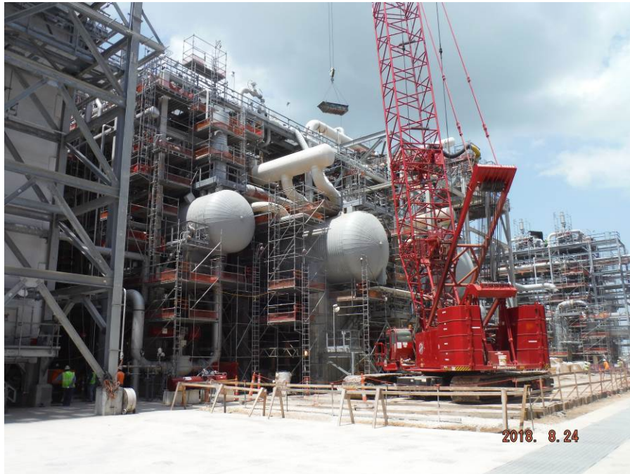
Train 5 – Propane Refrigeration Area Progress
