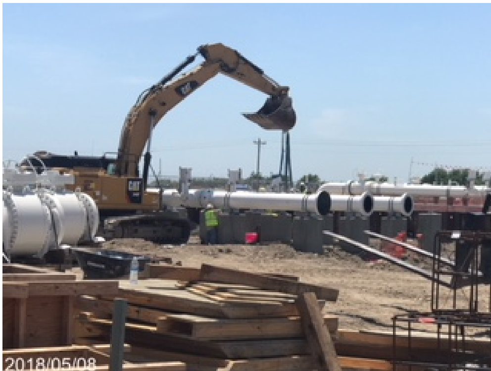
Meter station construction (CP13-2-000)
