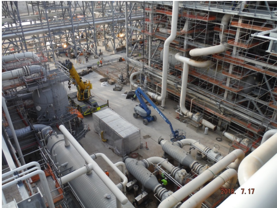
Train 5 – Construction Progress in Dehydration & Mercury Removal Area
