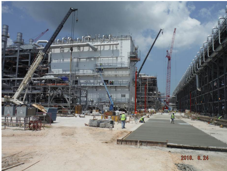
Train 5 – Area Paving Progress
