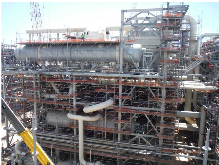
Train 5 – Construction progress for the J01 Structure
