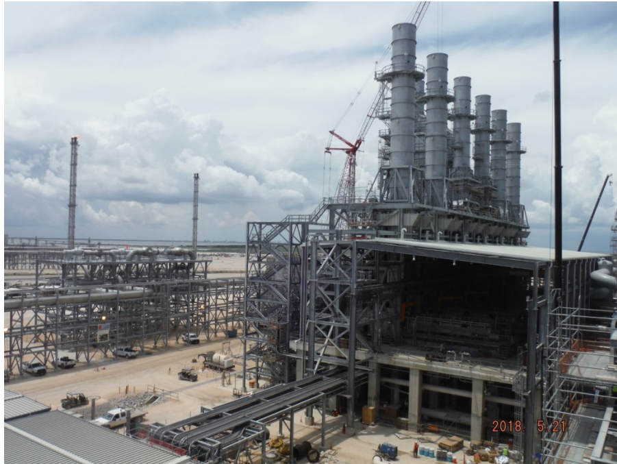
Train 5 – Construction Progress for the Compressor Deck
