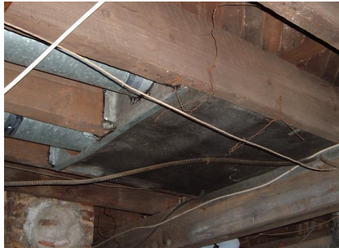
Using building cavities
