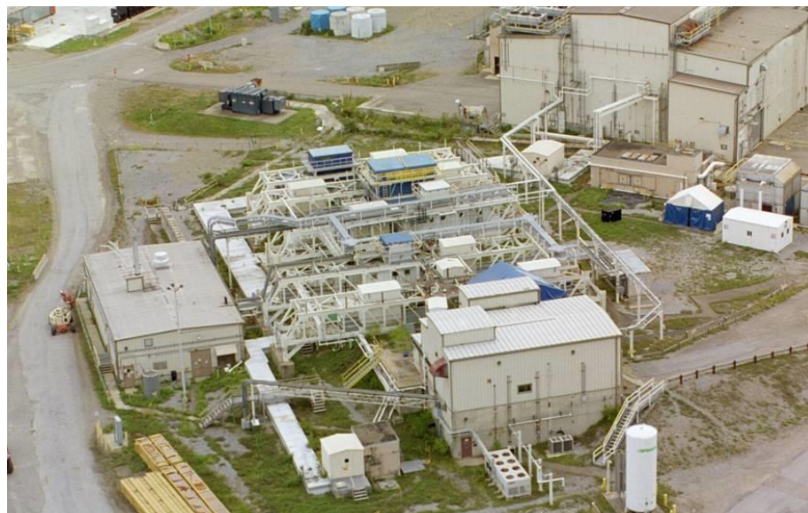
WVDP Waste Tank Farm
