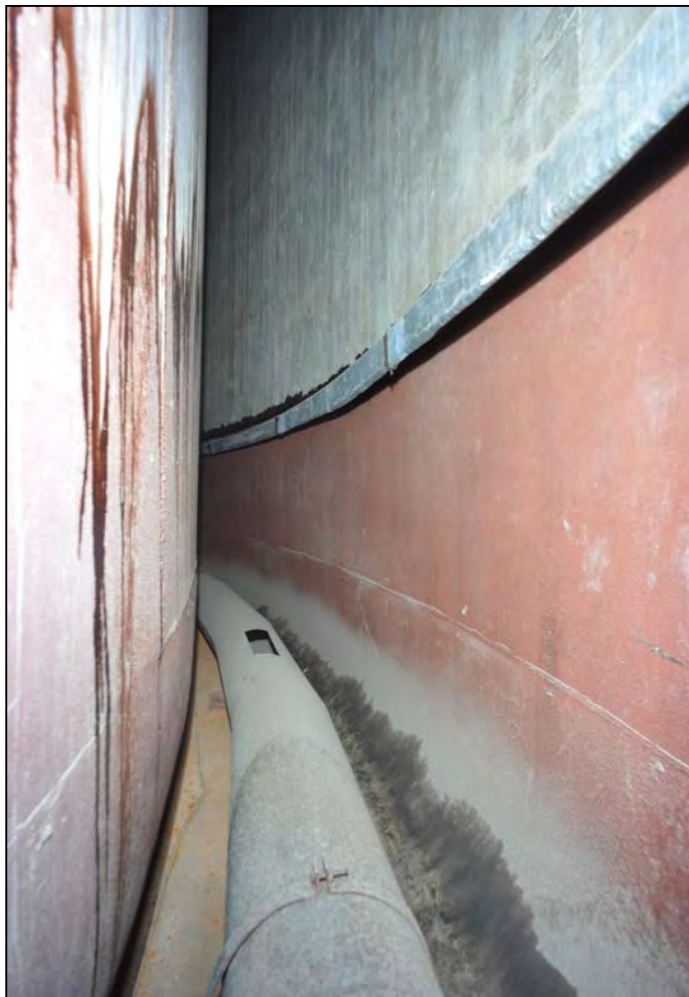
Tank 12H Annulus and Horizontal Ventilation Duct (West Riser)
