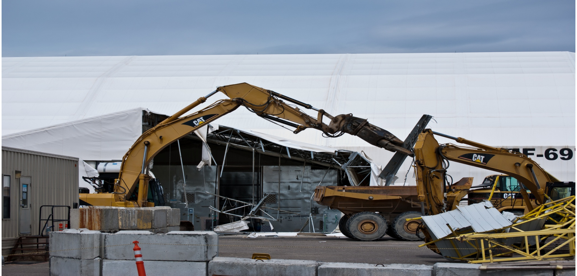
ARP airlock demolition
