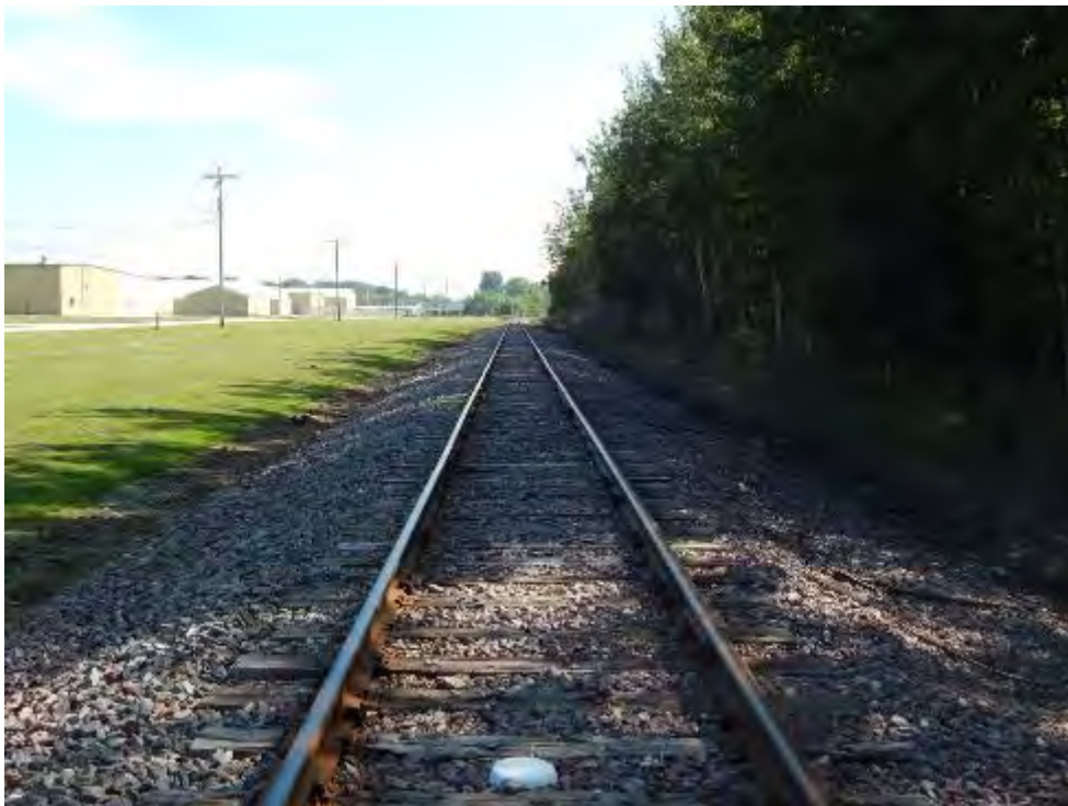
Figure 2-240. Potential Rockwood Spur at the Manitowoc Airport Transload Location (Looking South) (2014)
