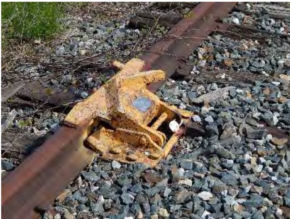
Figure 2-322. Derailer on Vermont Yankee Rail Spur (2016)
