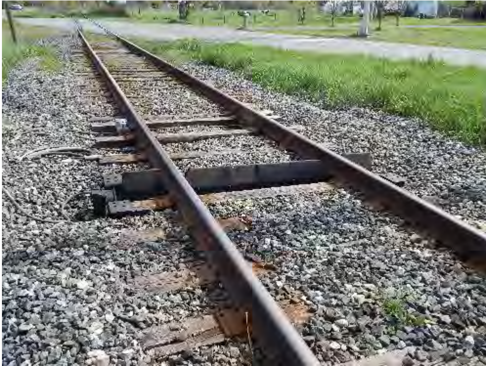
Figure 2-323. Dragging Equipment Detector and Hot Bearing Detector on New England Central Railroad Mainline (2016)
