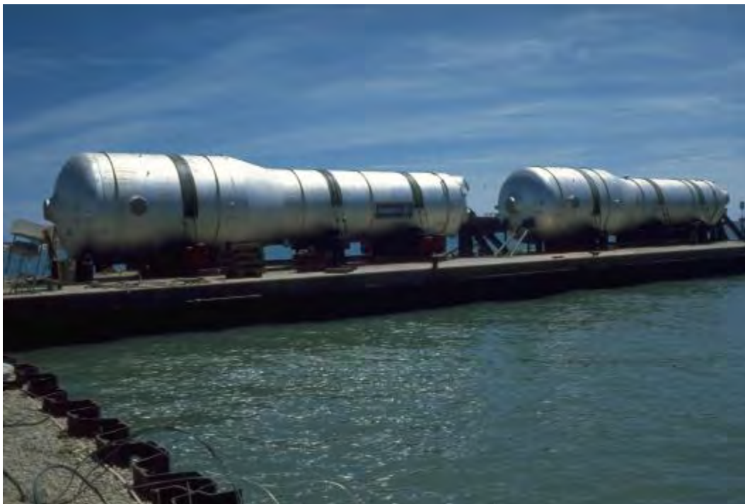
Figure 2-143. Steam Generators Being Delivered to Zion Site by Barge during Construction
