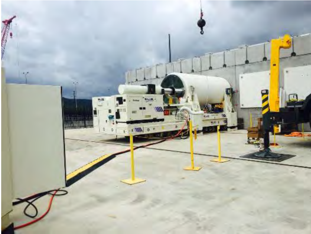
Photo courtesy of AREVA TN
