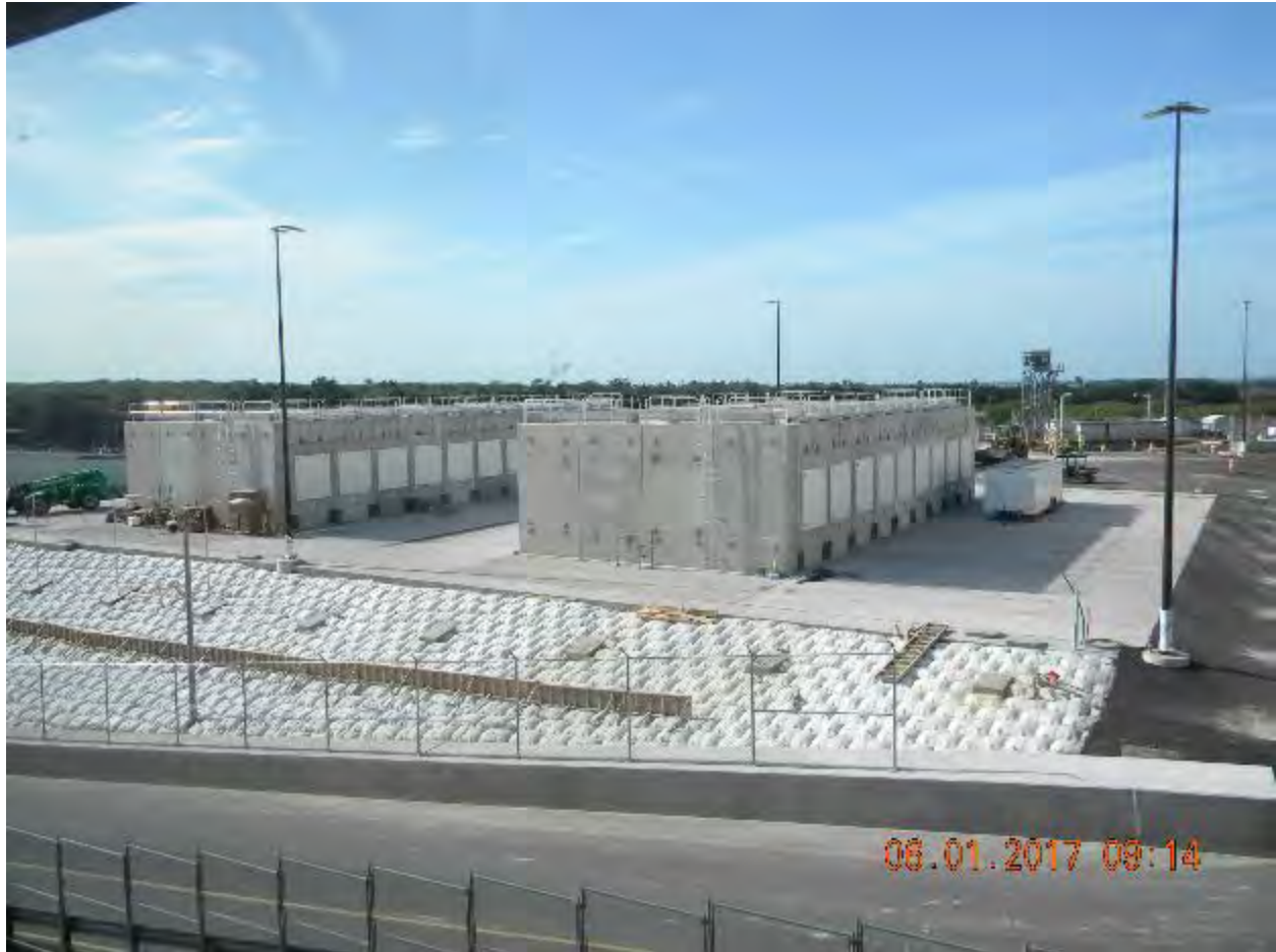
Figure 2-156. Crystal River Independent Spent Fuel Storage Installation with Horizontal Storage Modules Installed (2017)
