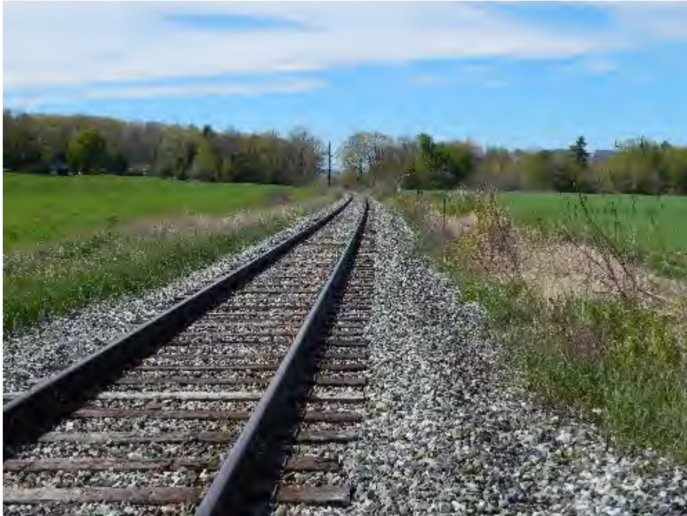
Figure 2-321. Junction of Vermont Yankee Rail Spur and New England Central Railroad Mainline Looking North (2016)
