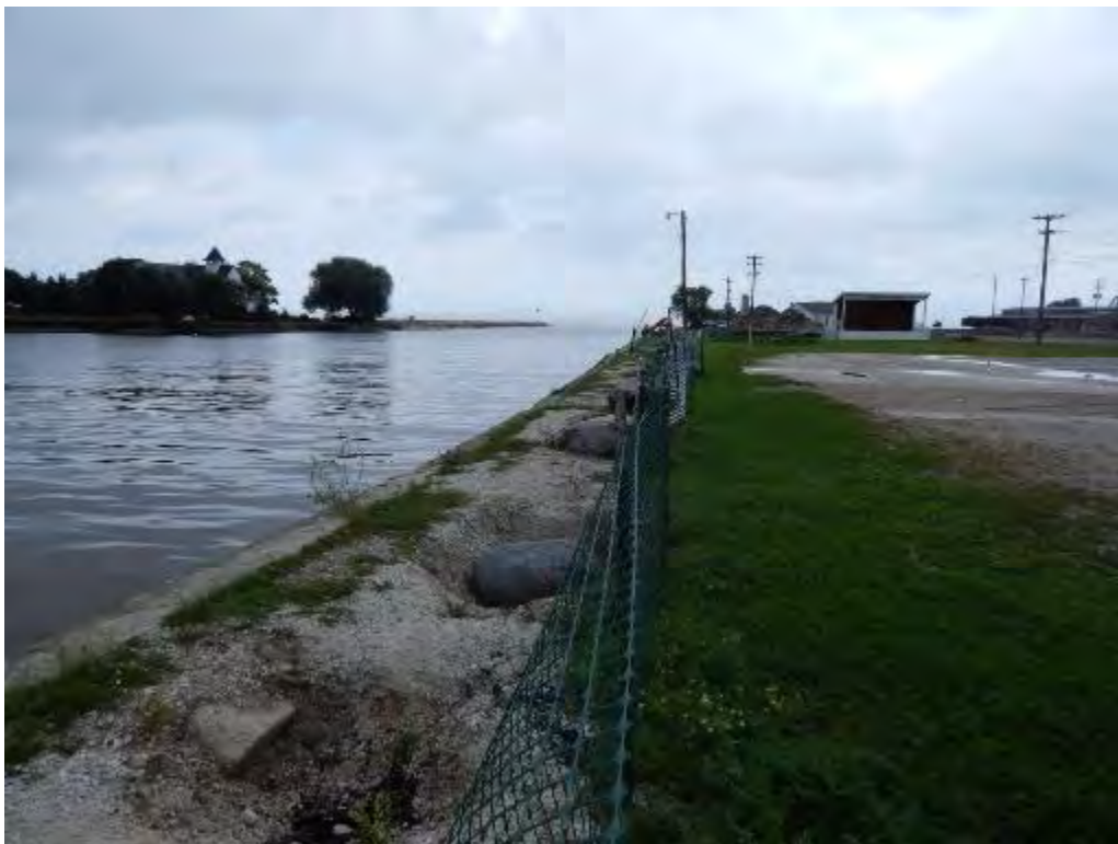
Figure 2-250. Potential Kewaunee Barge Transload Location Water Front (2014)
