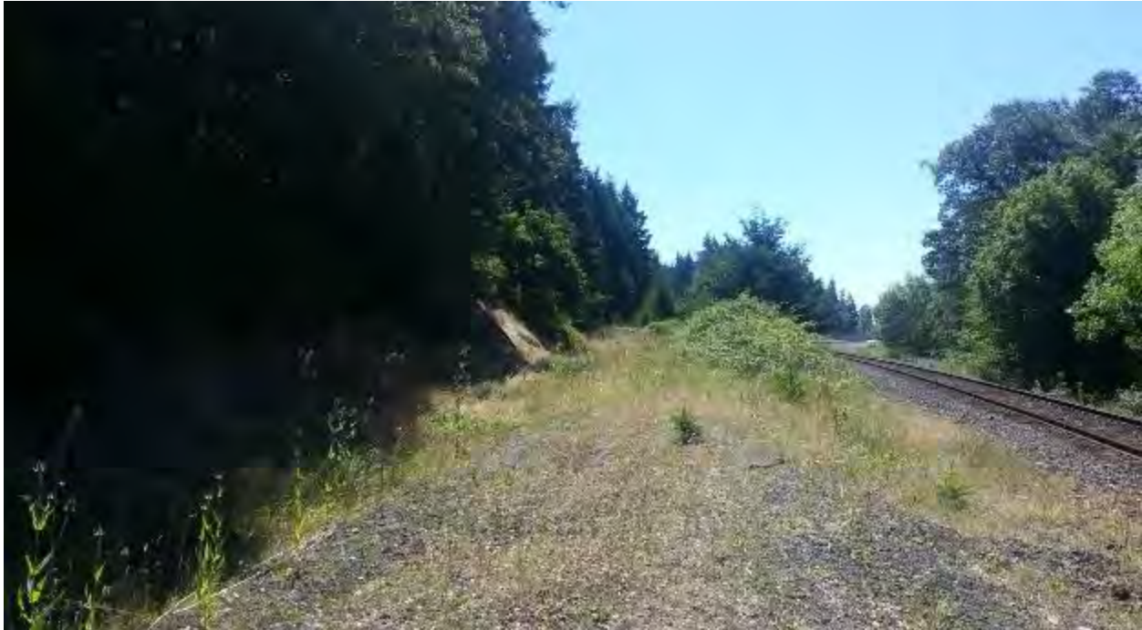
Figure 2-110. Former Trojan Rail Spur Railbed (2013)
