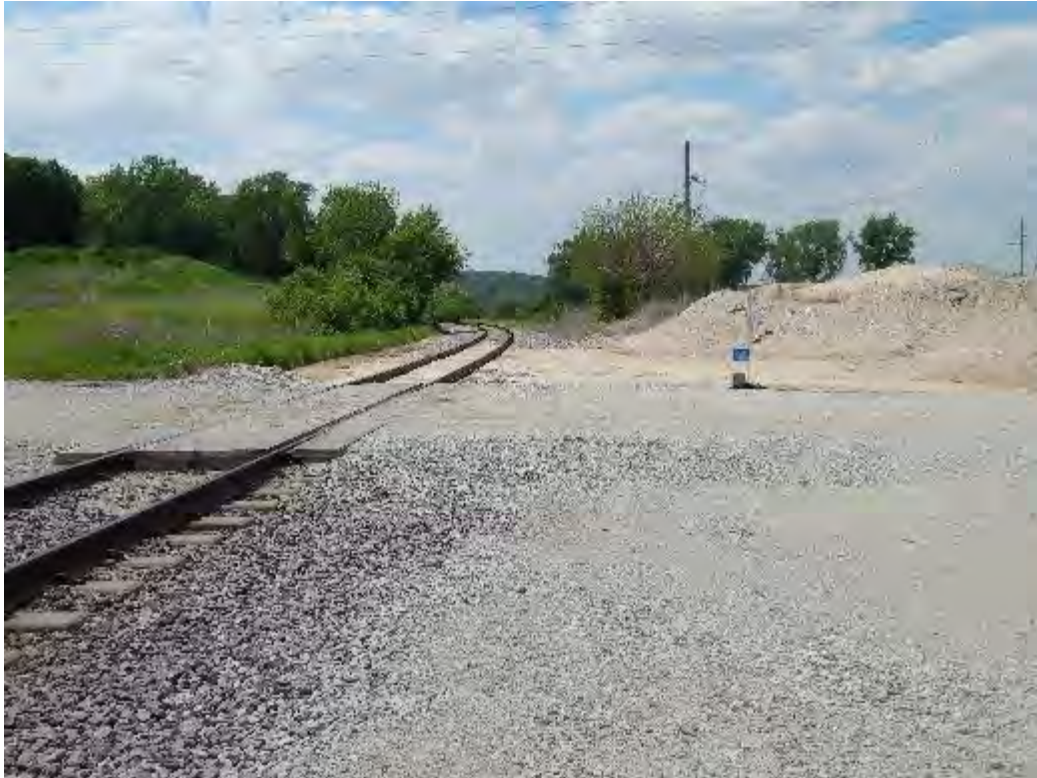
Figure 2-361. Current Condition of Transload Location (2017)
