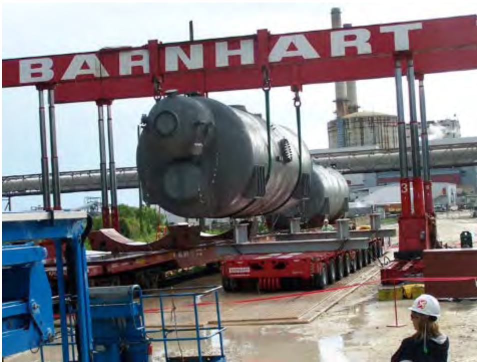
Figure 2-181. Moisture Separator Reheaters Being Unloaded at the Crystal River Site (2009)
