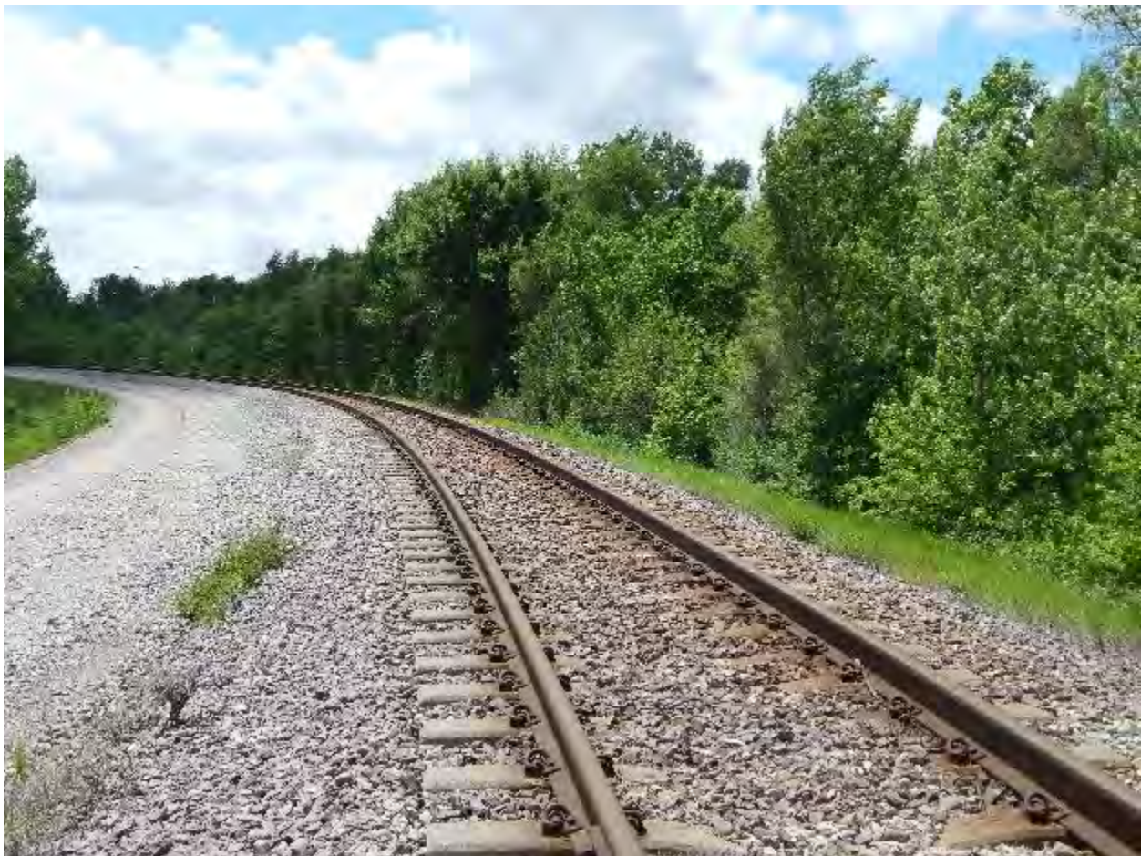
Figure 2-346. Track at Entrance to Cargill Industrial Spur (Looking South) (2017)
