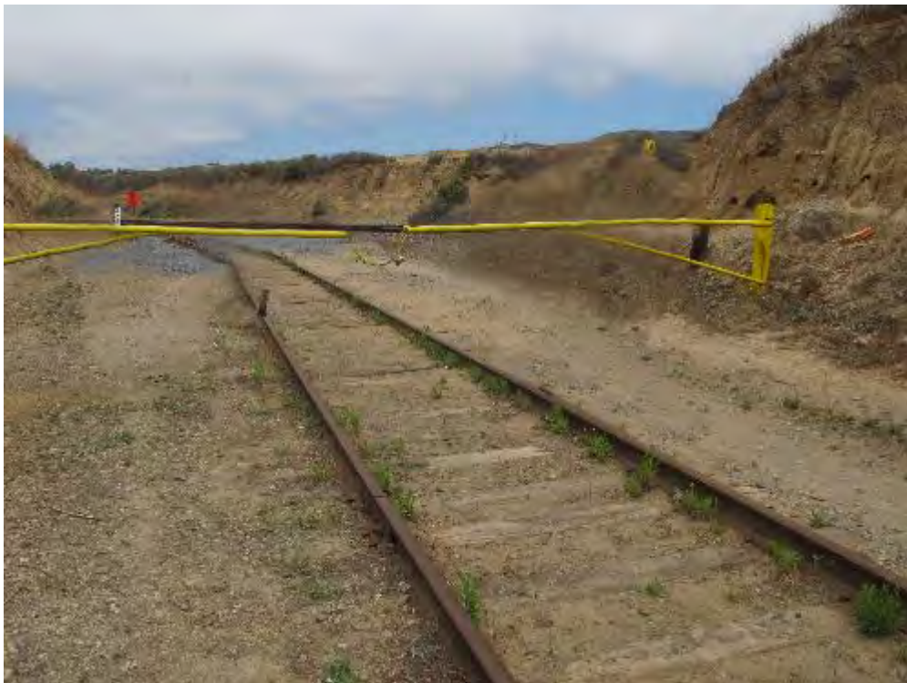
Figure B-58. Locked Facility Gate (2015)
