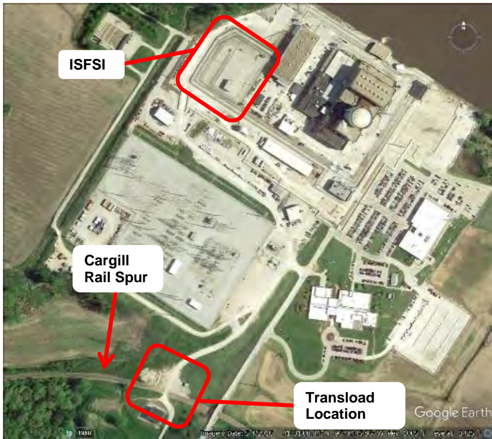
Figure 2-356. Aerial View of Transload Location (2017)
