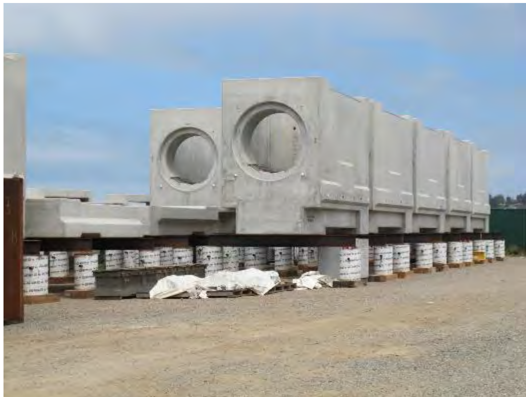
Figure 2-267. Horizontal Storage Modules (2015)
