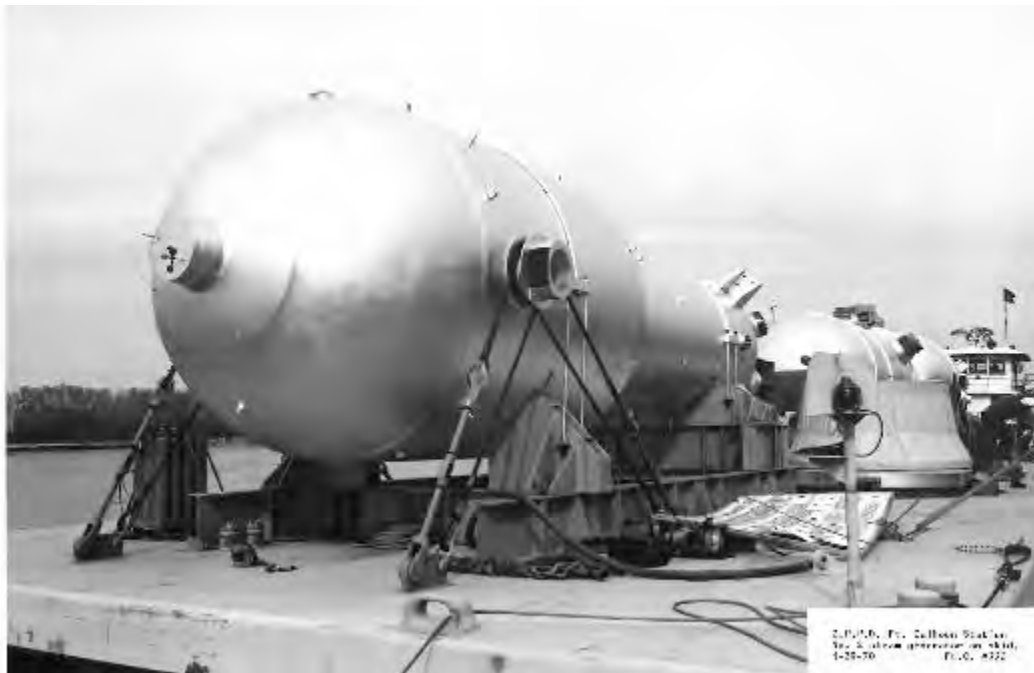
Photo courtesy of Fort Calhoun
