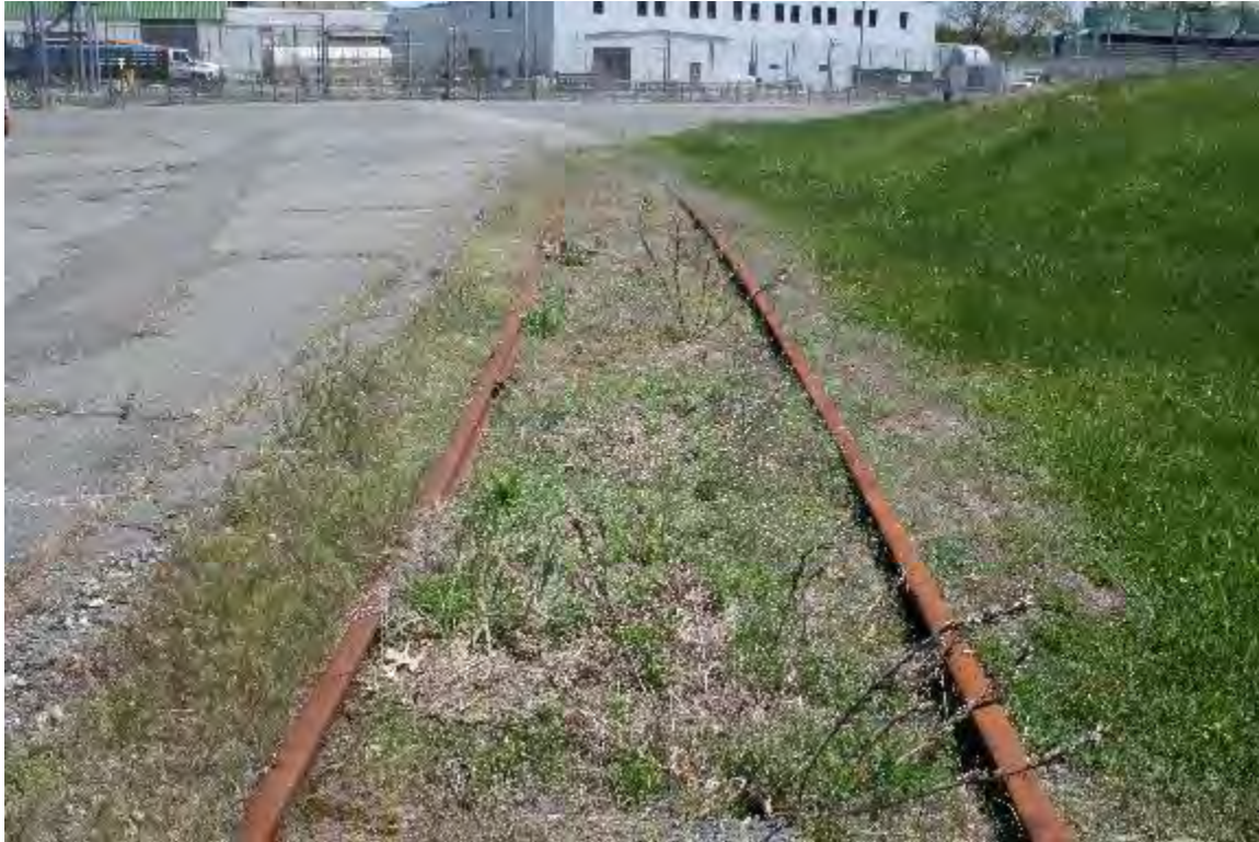
Photo courtesy of Vermont Yankee
