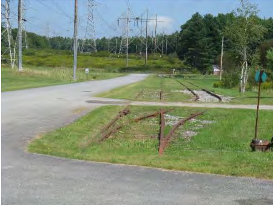
Figure 2-14. Paved-over Railroad Tracks at the Maine Yankee Site (2012)
