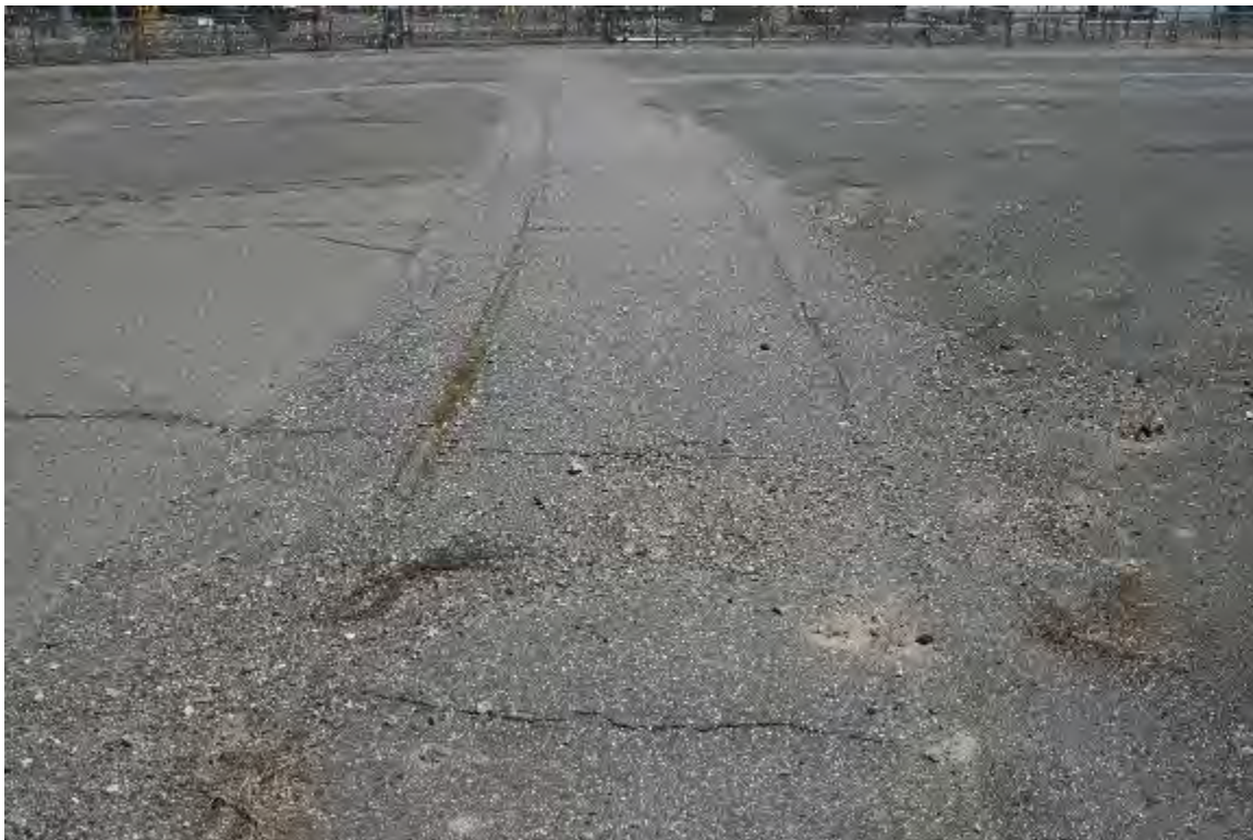
Photo courtesy of Vermont Yankee
