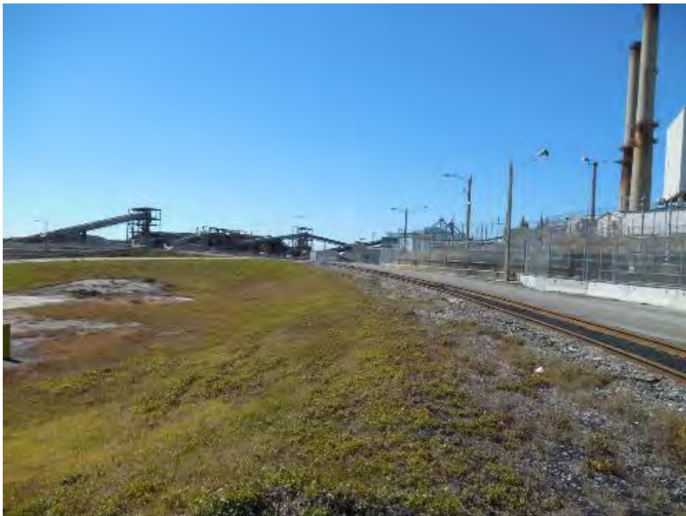
Figure 2-162. Onsite Industrial Rail Spur in Front of the Independent Spent Fuel Storage Installation Site (Looking West) (2015)
