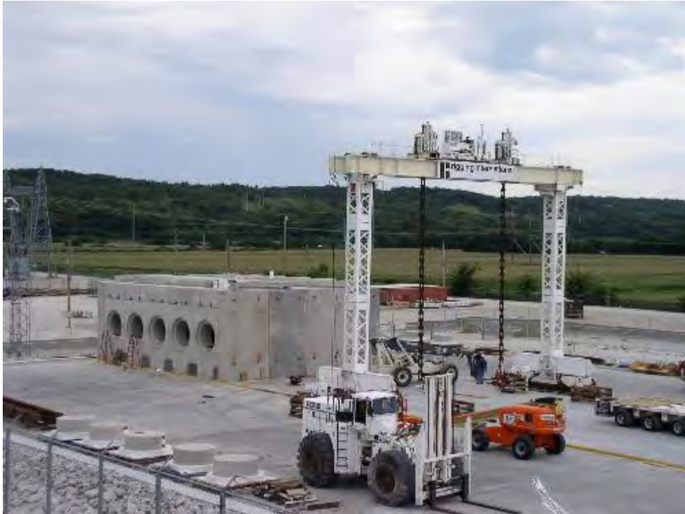
Photo courtesy of Fort Calhoun
