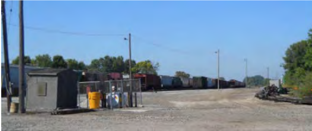
Figure B-39. Calumet Yard in Manitowoc, Wisconsin (2014)
