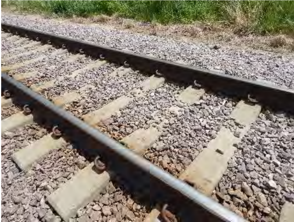
Figure 2-343. Rail, Concrete Ties, and Pandrol Clips on Cargill Industrial Spur (2017)
