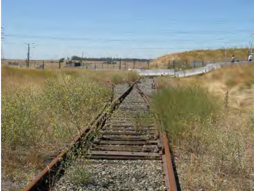
Figure 2-92. Junction of the On-site Track Spur Running Adjacent to the Independent Spent Fuel Storage Installation (Right) and the Longer Track Running into the Rancho Seco Site (Left) (2013)
