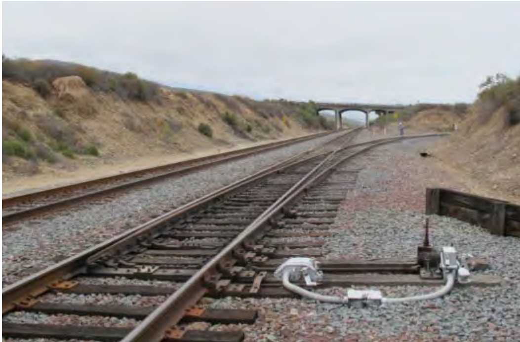
Figure B-56. Manually Operated, Timed Switch (2015)
