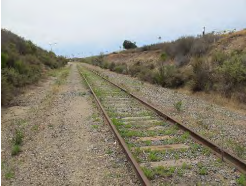
Figure 2-284. Onsite Rail Spur at San Onofre Site (2015)
