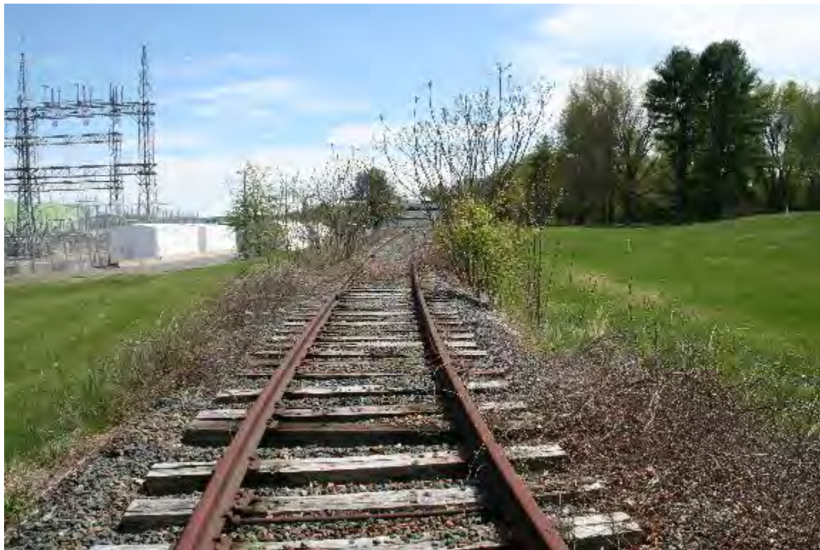
Photo courtesy of Vermont Yankee
