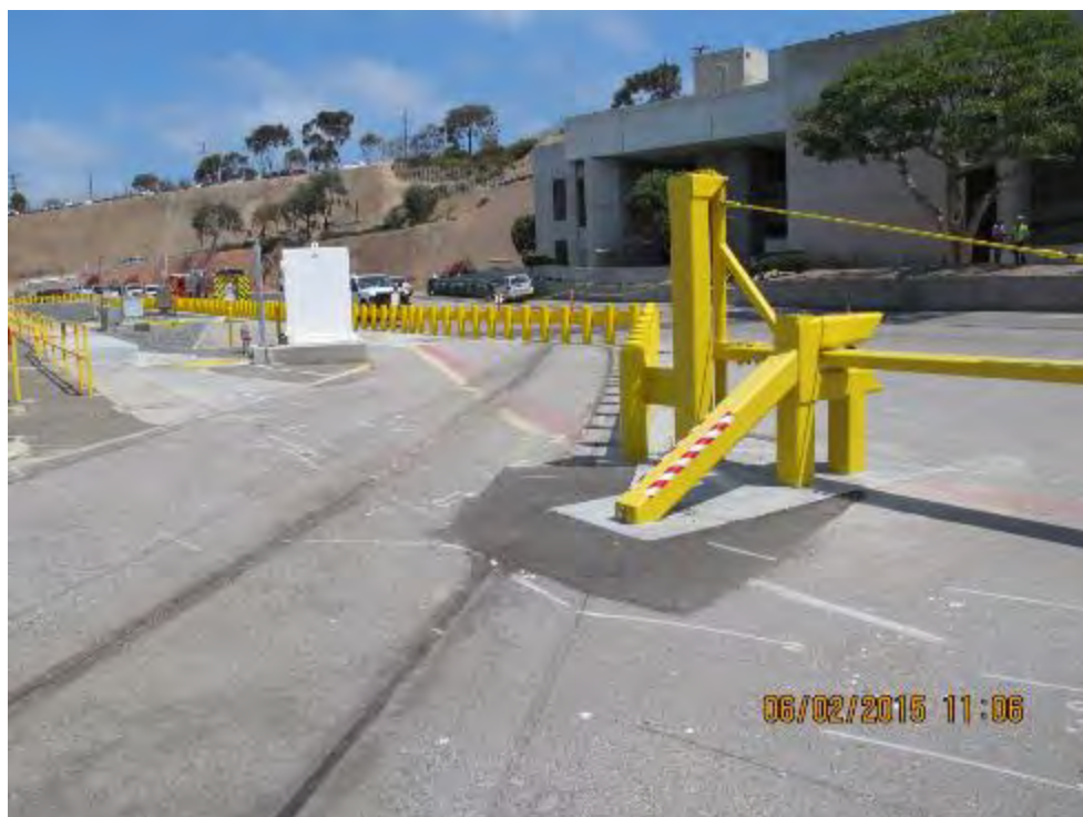
Figure 2-283. Onsite Rail System and Vehicle Barrier near Independent Spent Fuel Storage Installation at San Onofre Site (Looking Northeast) (2015)
