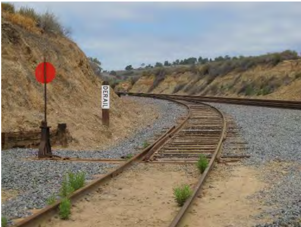
Figure 2-285. Junction of Onsite Rail Spur with Mainline at San Onofre Site (2015)
