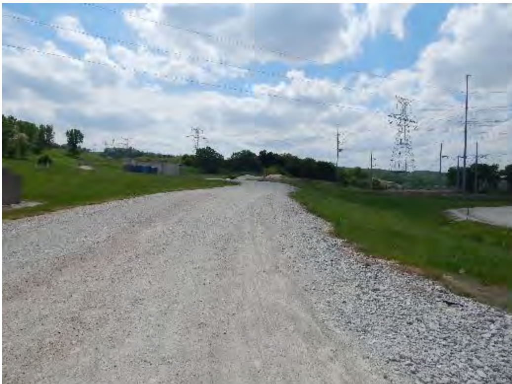
Figure 2-362. Current Condition of Haul Road (2017)
