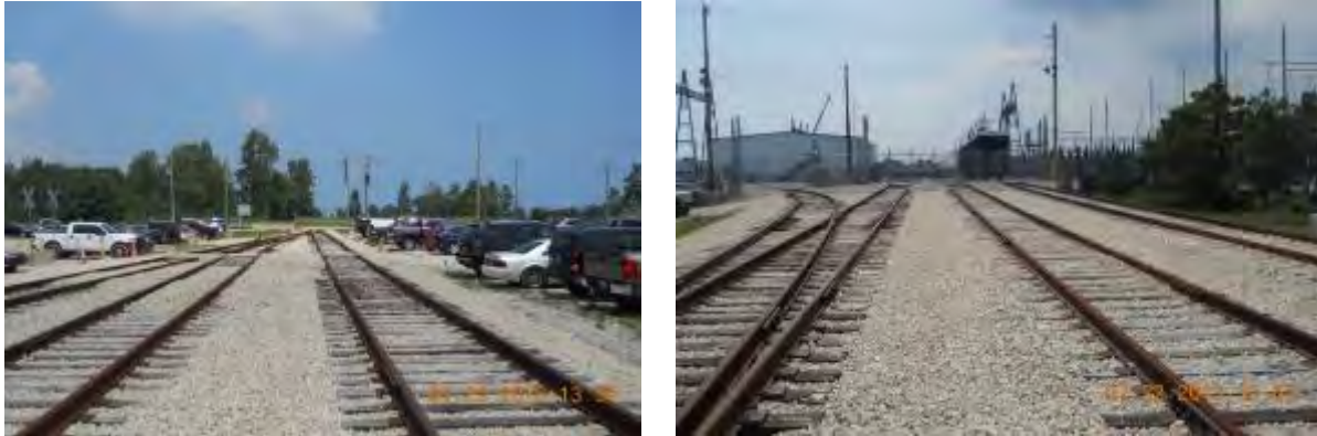
Figure B-19. Zion Site Plant Lead (2013)
