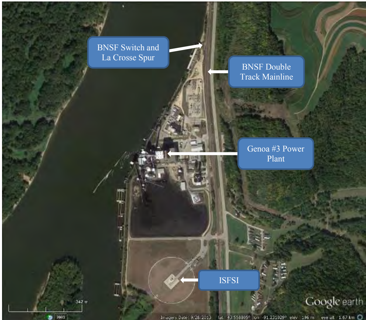
Figure B-13. Satellite View of the La Crosse Site with Switch, Spur, Mainline, and Independent Spent Fuel Storage Installation (Google 2017)
