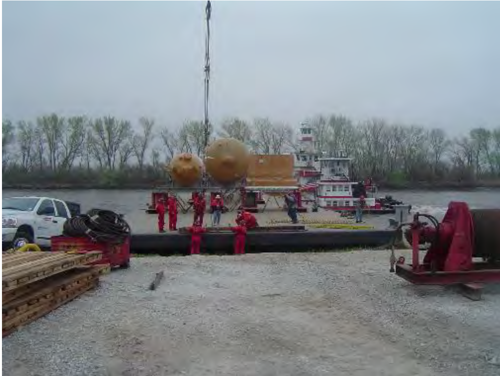
Photo courtesy of Fort Calhoun
