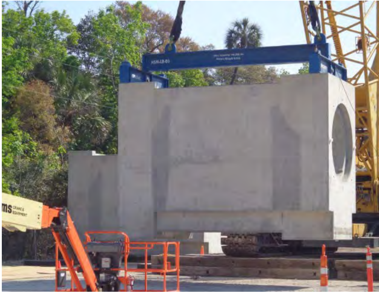
Figure 2-188. Horizontal Storage Module Being Unloaded from Railcar (2015)
