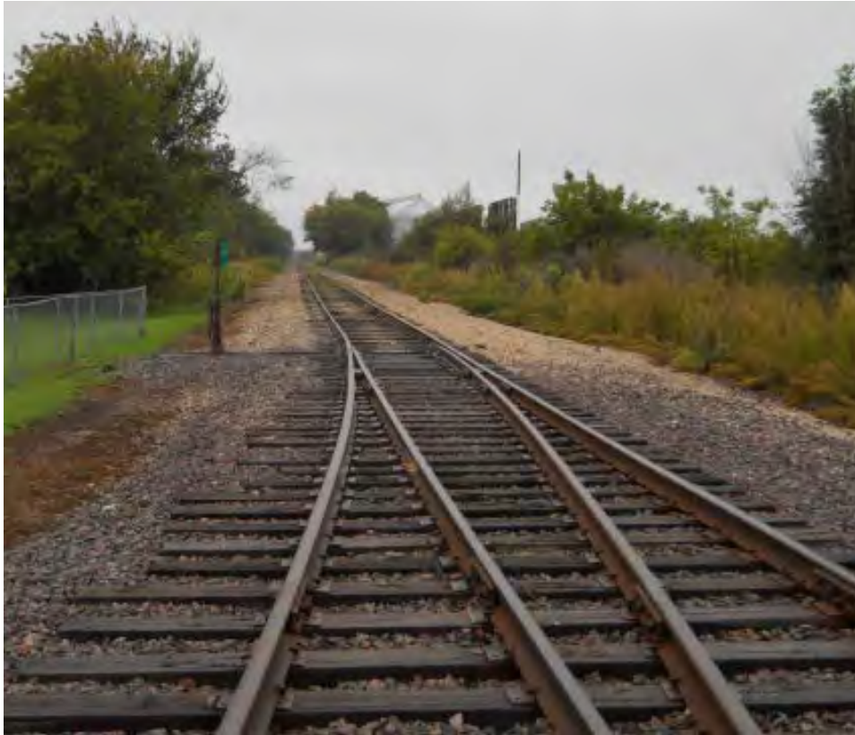
Figure B-43. Switch at Luxemburg (2014)
