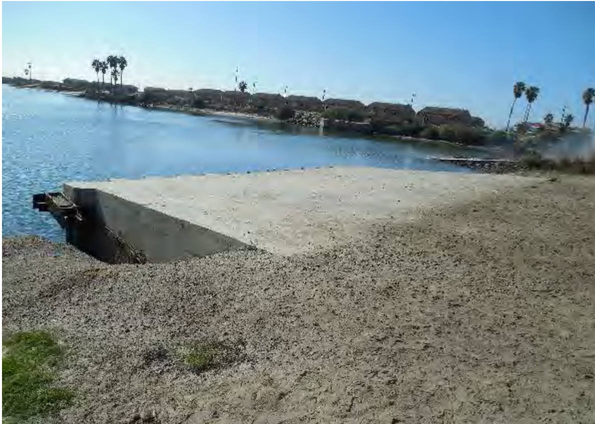
Figure 2-299. Del Mar Boat Basin Bulkhead (2016)
