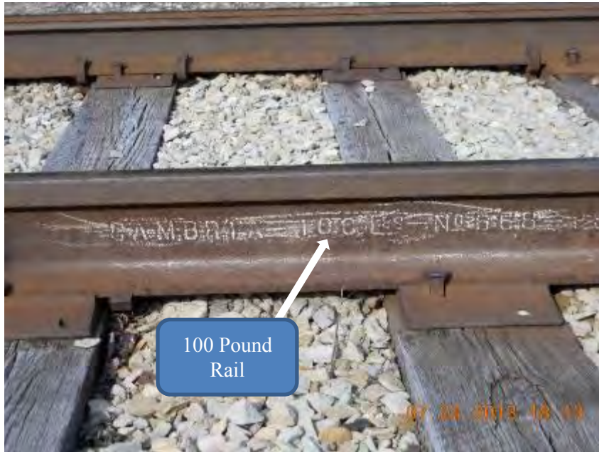
Figure B-5. Railroad Track Located Near Petoskey, Michigan Transload Location (2013)
