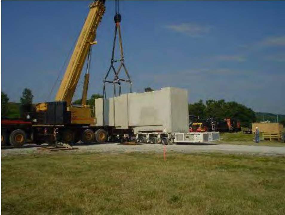
Figure 2-357. Horizontal Storage Module Being Transloaded from Railcar to Self-Propelled Modular Transporter
