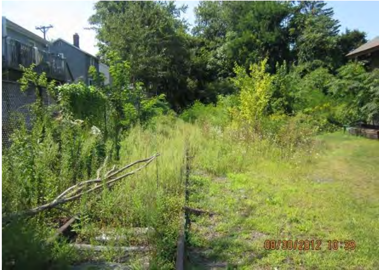
Figure 2-42. Conditions at the End of the Portland Rail Spur (2012)
