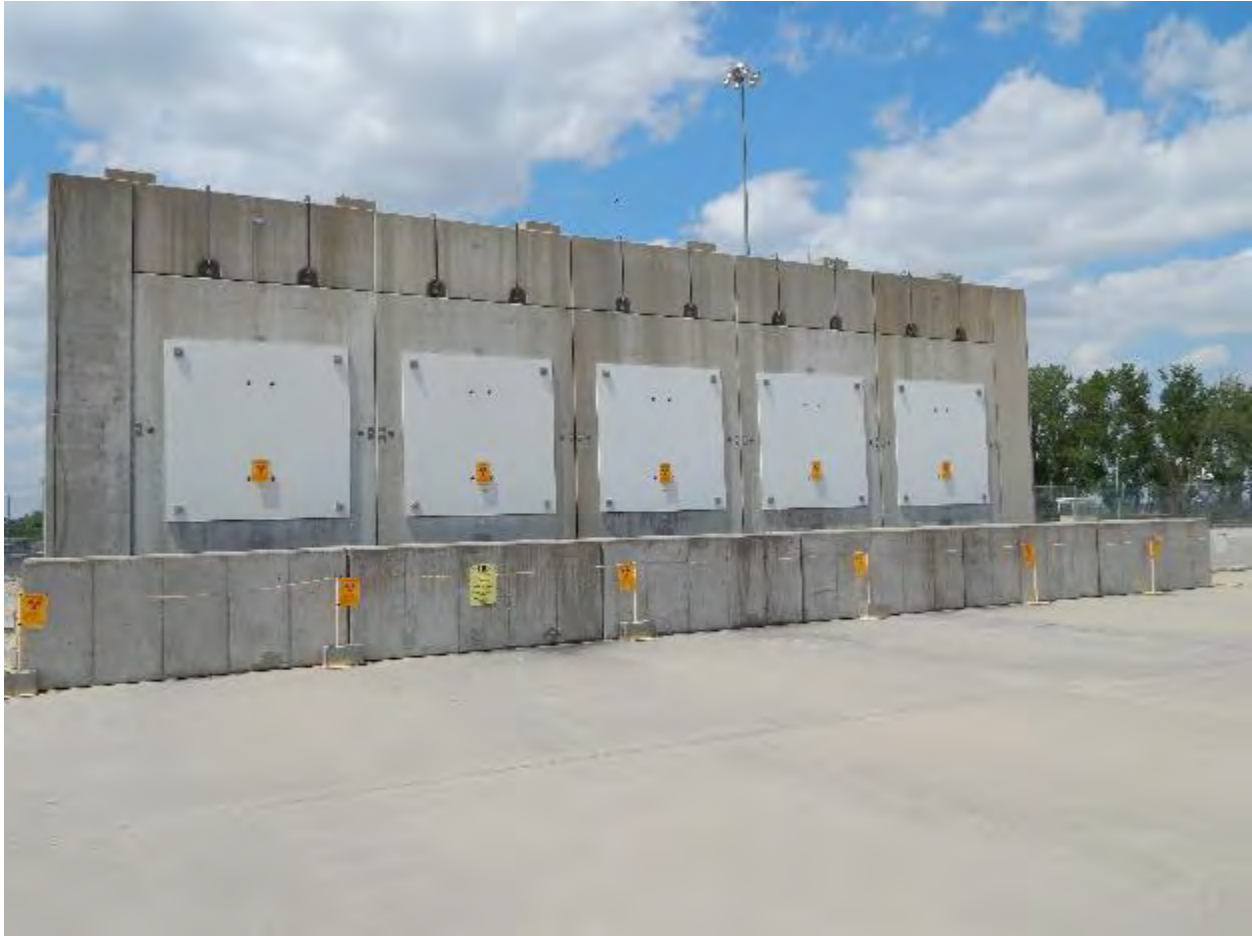
Figure 2-338. Fort Calhoun Independent Spent Fuel Storage Installation (2017)
