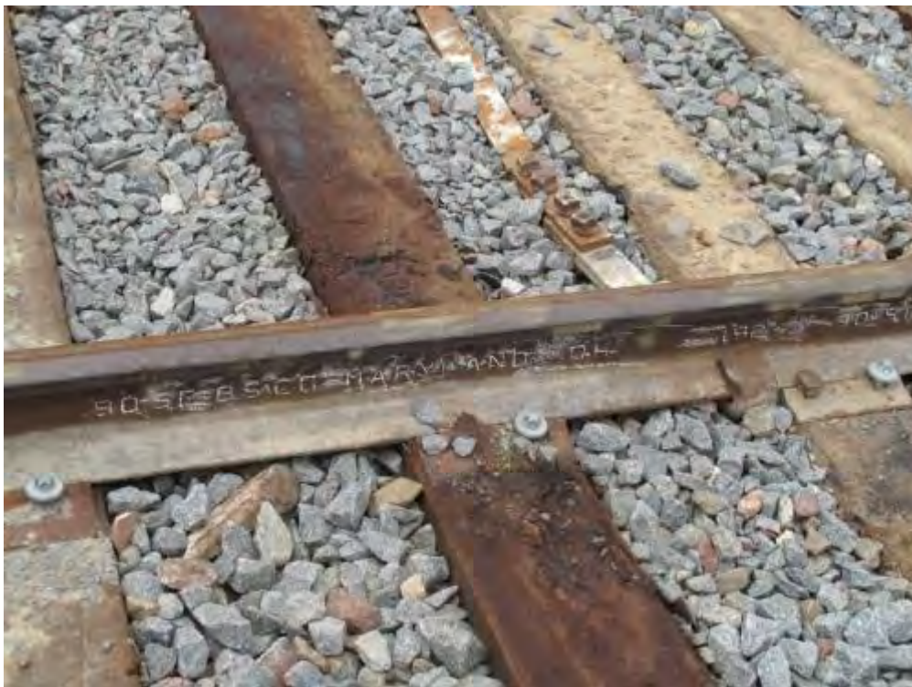
Figure B-60. Site Lead 90-lb. Rail (2015)
