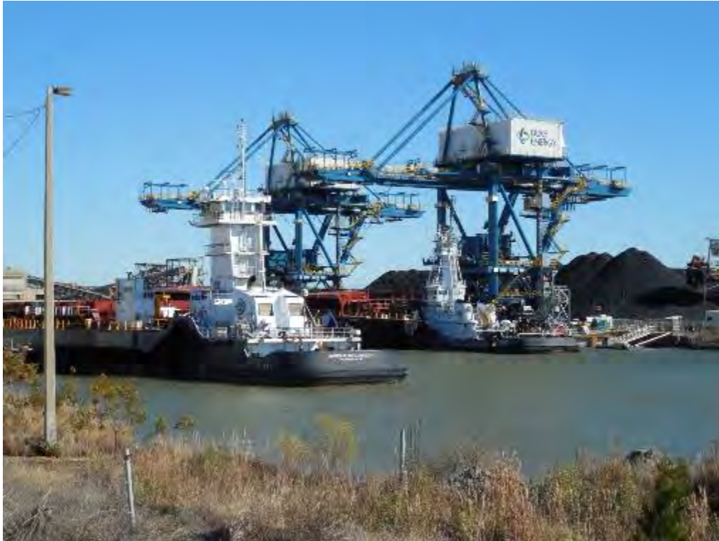
Figure 2-166. Current Barge Area Used for Unloading Coal Barges (2015)
