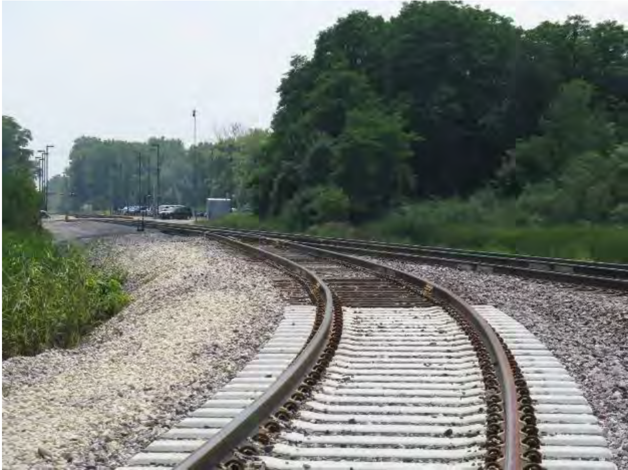
Figure 2-148. Junction of Zion On-site Rail Spur with Union Pacific Railroad Showing Concrete Rail Ties (2013)
