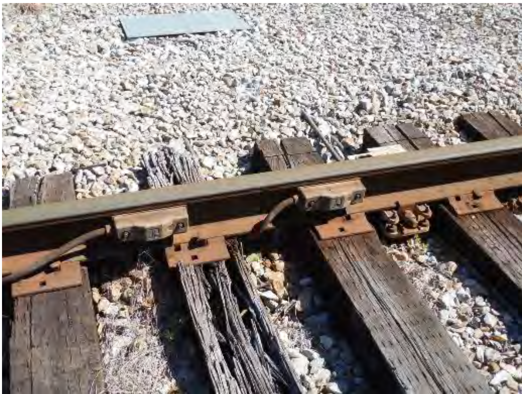
Figure 2-175. Wheel Detectors on Florida Northern Railroad (2015)
