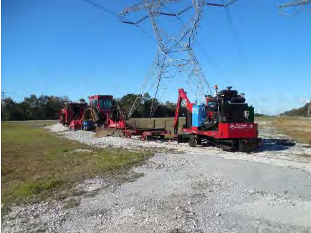
Figure 2-178. Track Maintenance Equipment Staged at the Mine Spur (2015)
