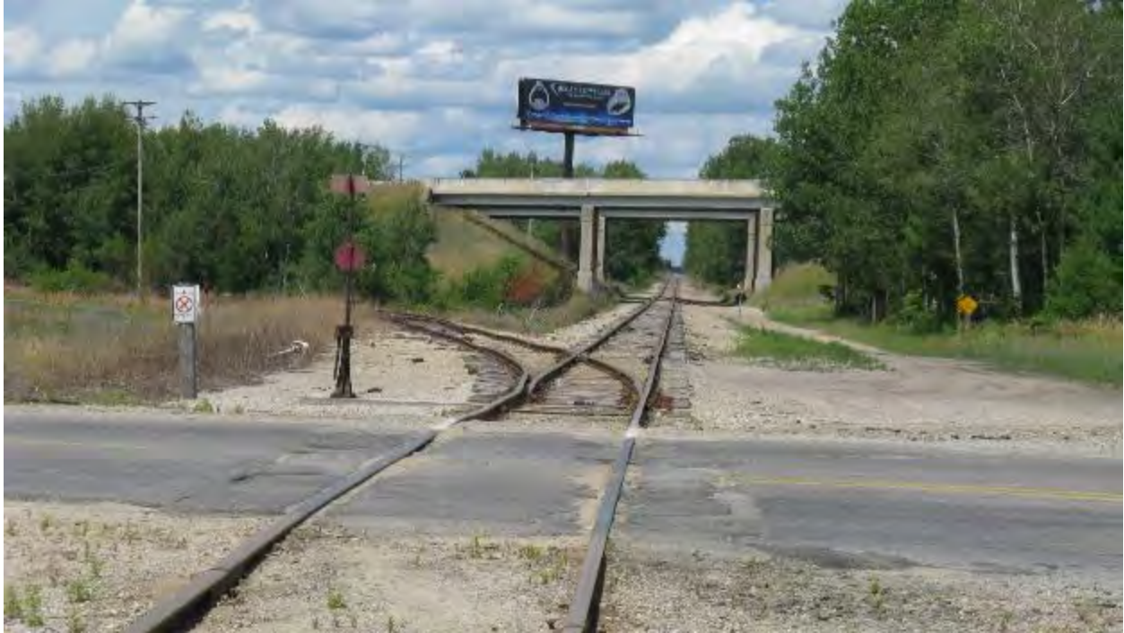
Figure 2-78. Condition of Rail Crossing Used for Big Rock Point Reactor Pressure Vessel Transload (Looking North) (2013)
