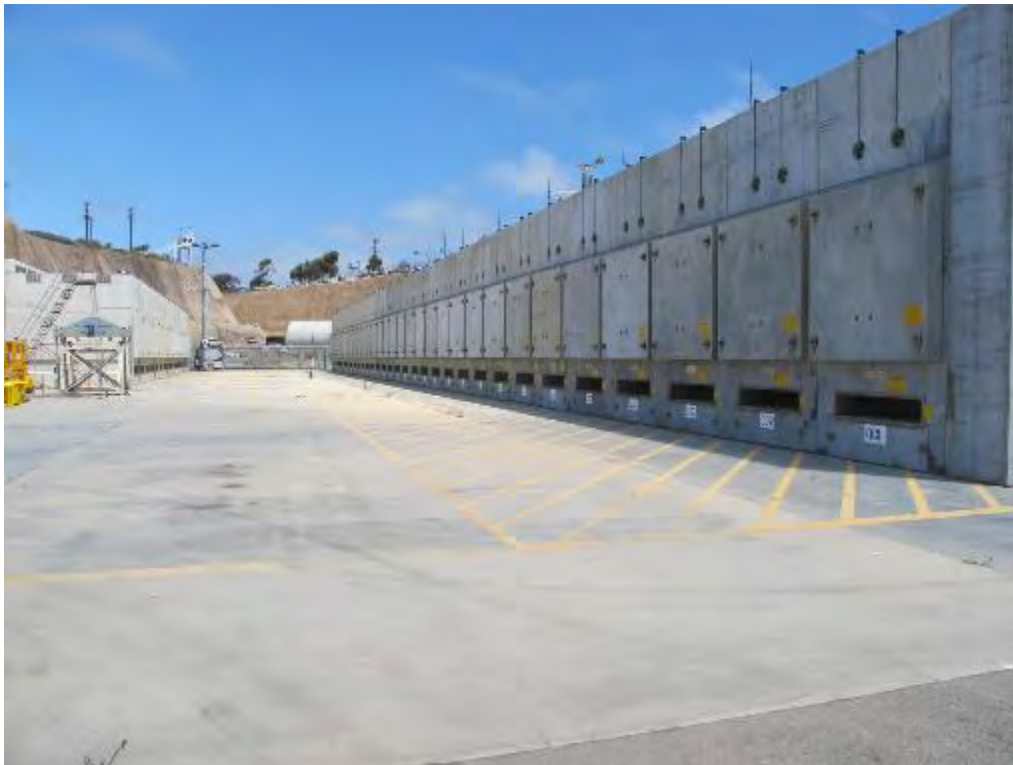
Figure 2-277. Close-up View of San Onofre Independent Spent Fuel Storage Installation (2015)
