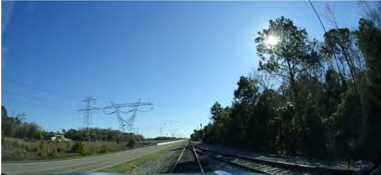
Figure 2-163. Onsite Industrial Rail Spur at the Coal Loop Junction (2015)
