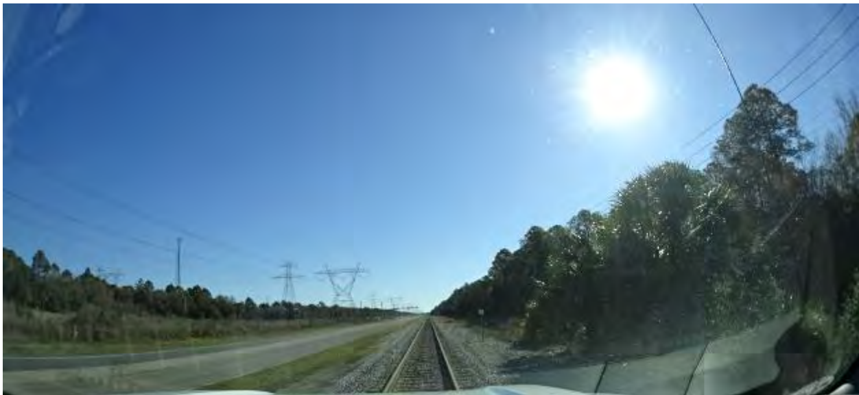
Figure 2-164. Onsite Industrial Rail Spur Approaching U.S. Highway 19 from the West (2015)
