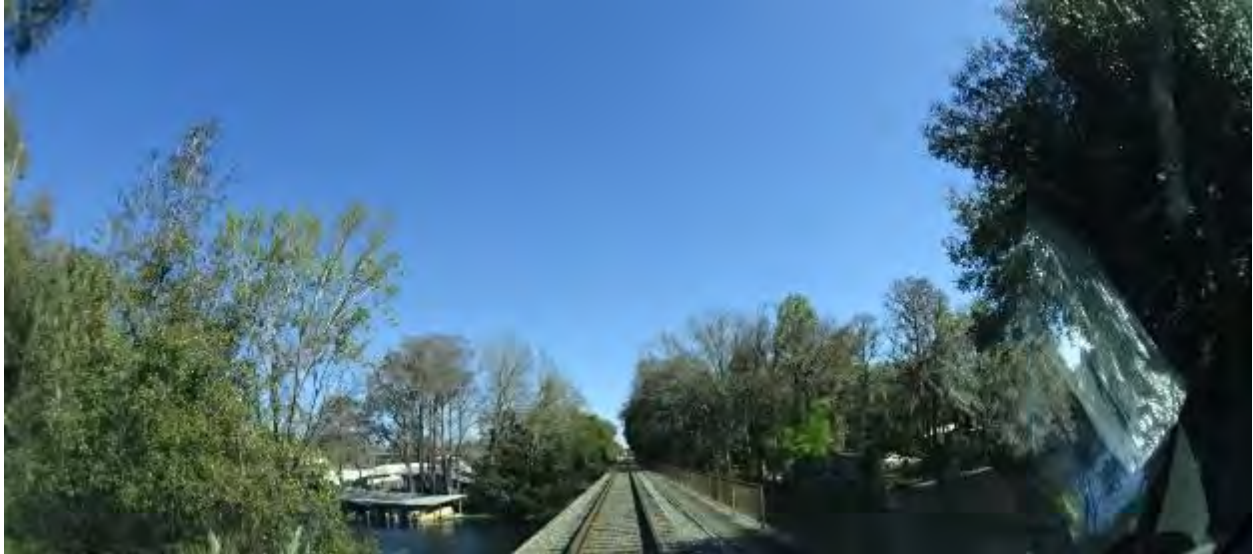
Figure 2-174. Florida Northern Railroad Bridge (2015)
