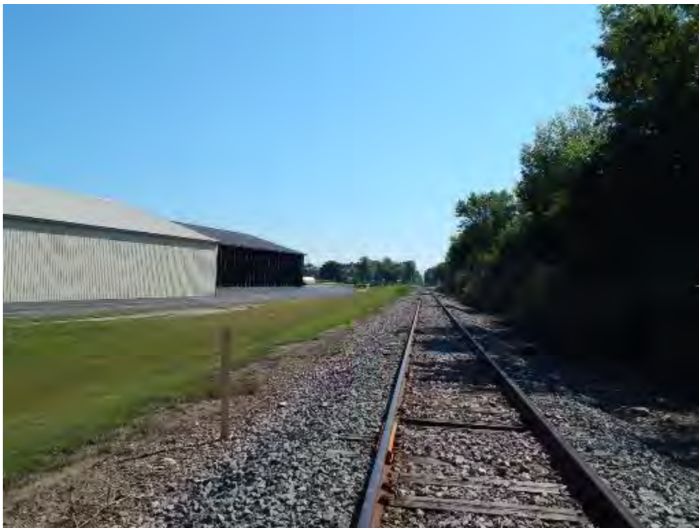
Figure 2-233. Potential Rockwood Spur at WI-310 Transload Location (Looking South) (2014)
