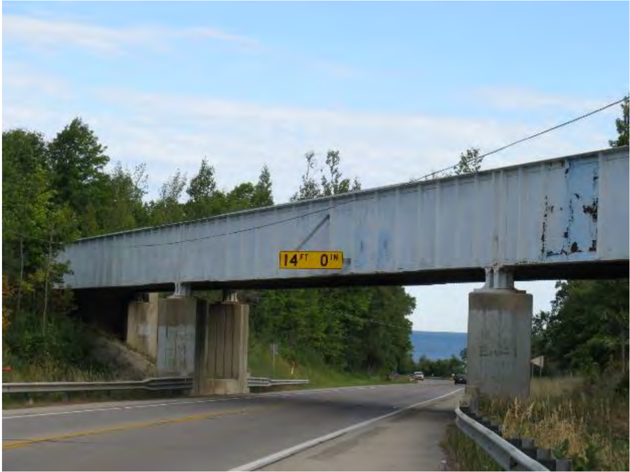
Figure 2-76. Low Overhead Clearance Abandoned Railroad Bridge on U.S. 31 (2013)
