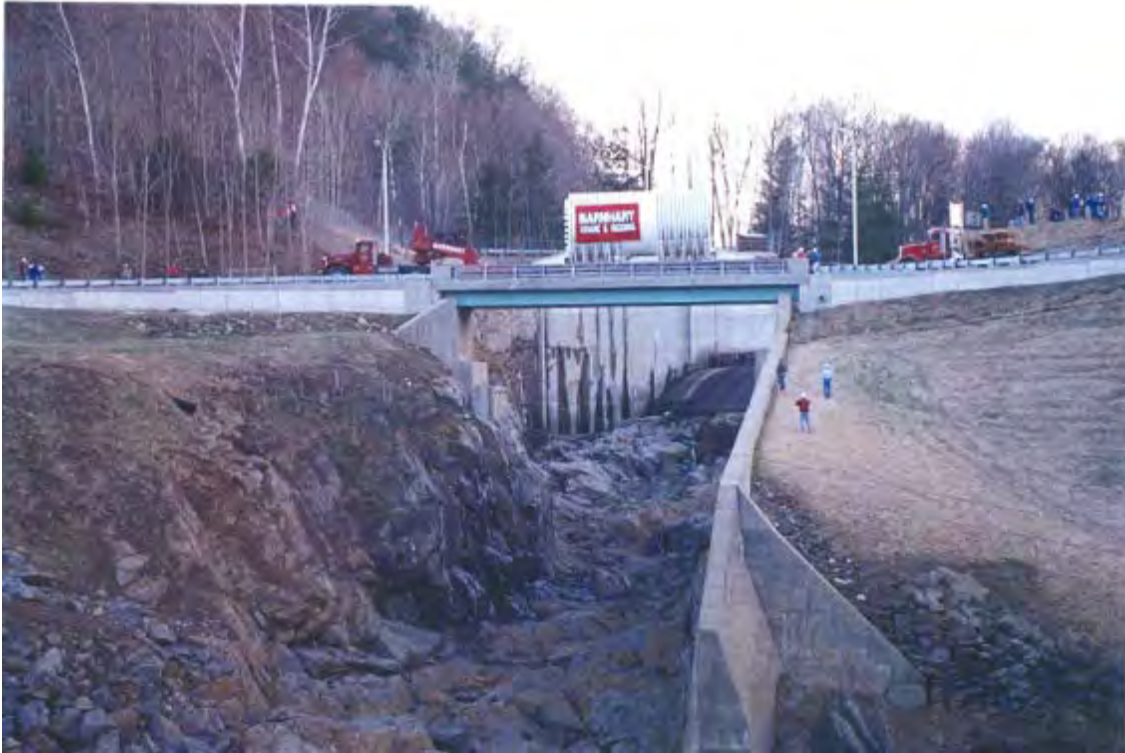
Photo courtesy of AREVA
