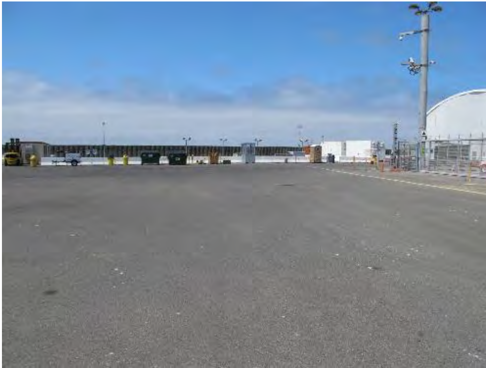
Figure 2-280. Expanded San Onofre Independent Spent Fuel Storage Installation Location (2015)
