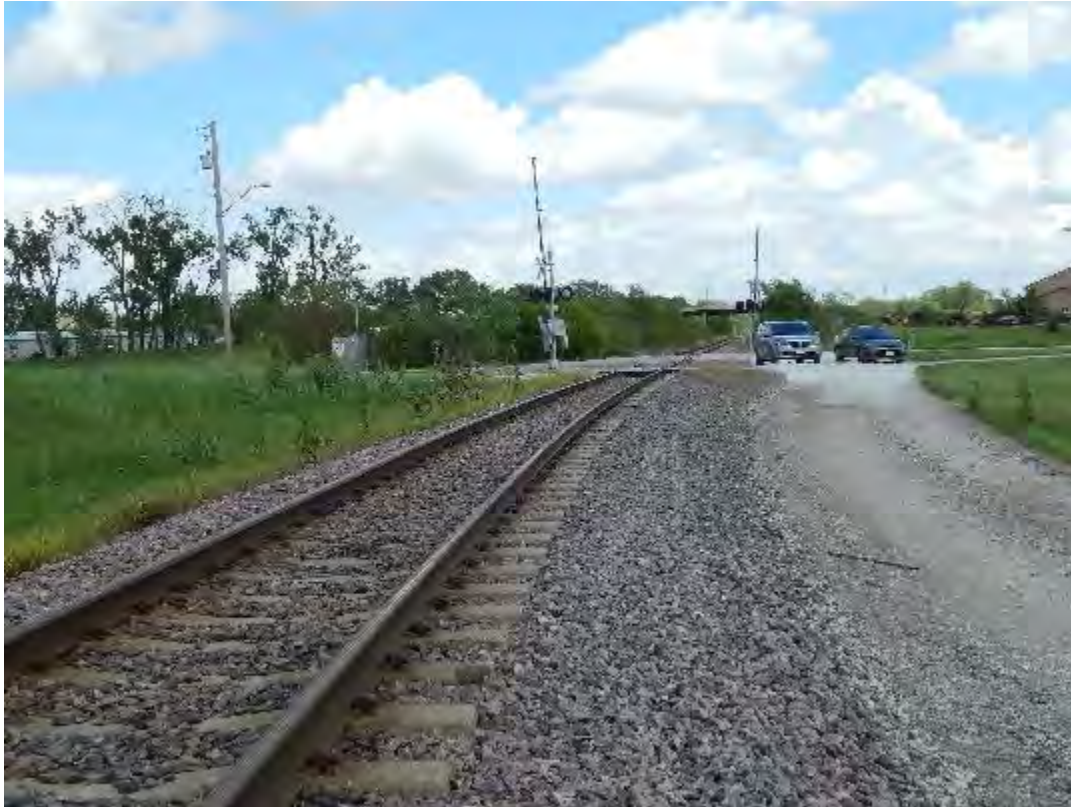
Figure 2-347. Track at Entrance to Cargill Industrial Spur (Looking North) (2017)
