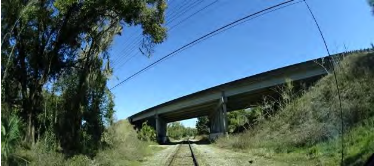
Figure 2-172. Highway Bridge over Florida Northern Railroad (2015)
