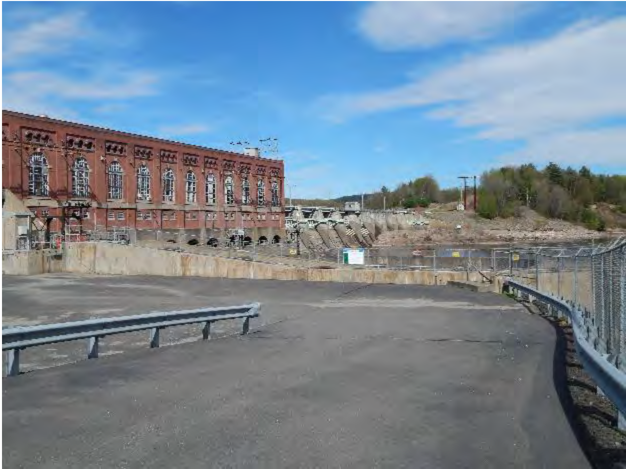
Figure 2-308. Vernon Dam and Hydroelectric Station (2016)
