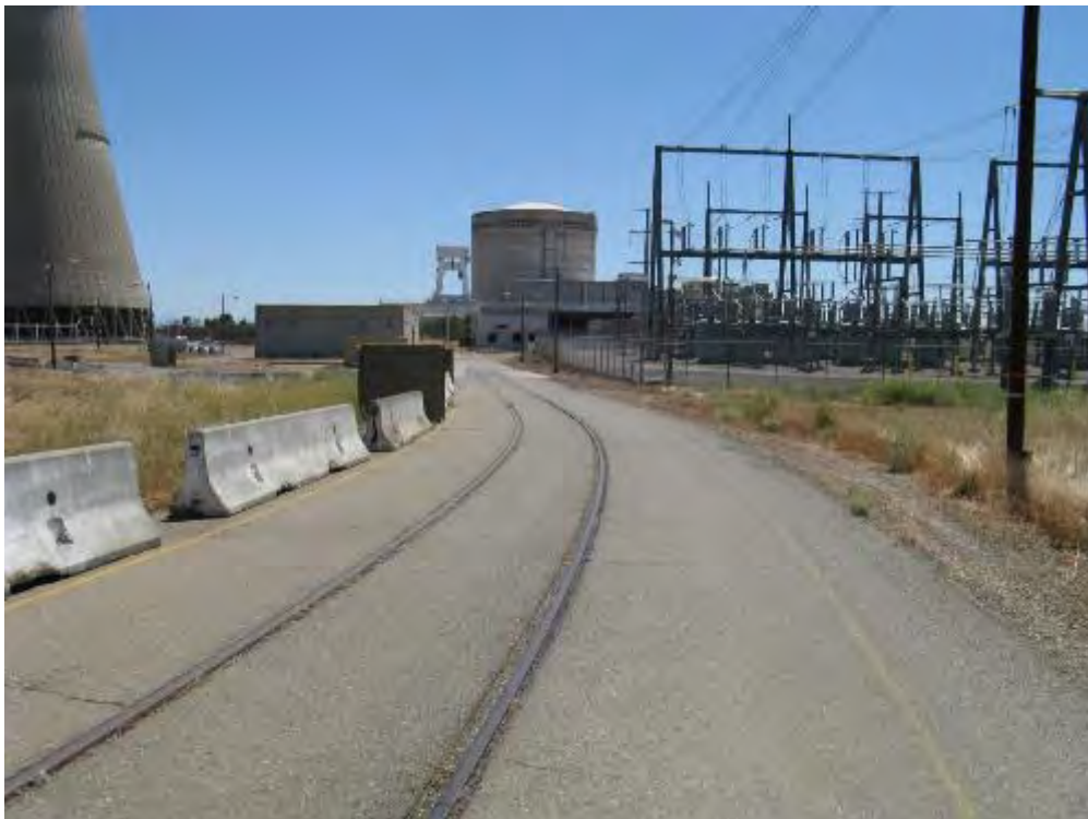
Figure 2-93. On-site Rail Spur Running into Rancho Seco Site (2013)
