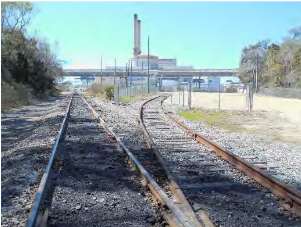
Figure 2-160. Junction of Onsite Industrial Spur (Left) and Nuclear Spur (Right) (2015)
