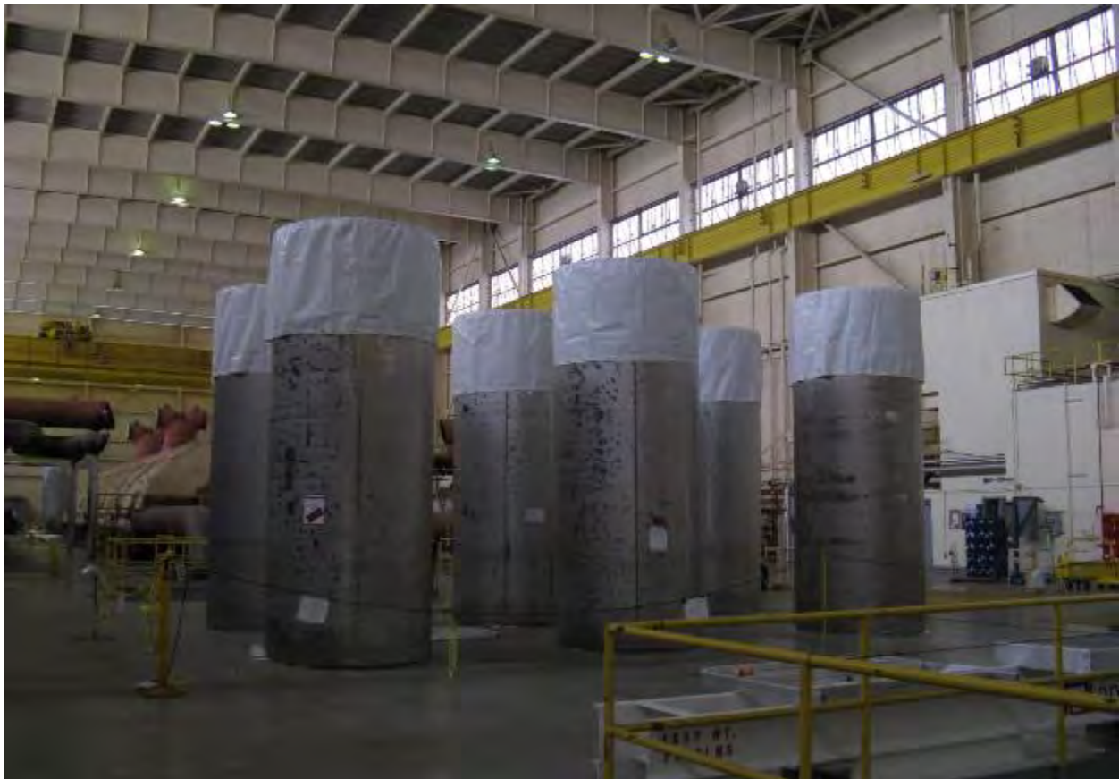
Figure 2-141. Used Nuclear Fuel Transportable Storage Canisters Staged at Zion (2013)
