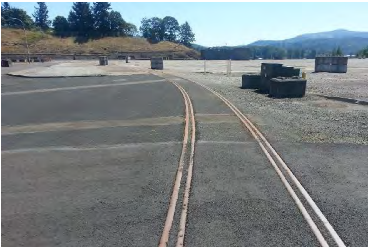
Figure 2-111. Remnants of On-site Rail Spur at Trojan (2013)
