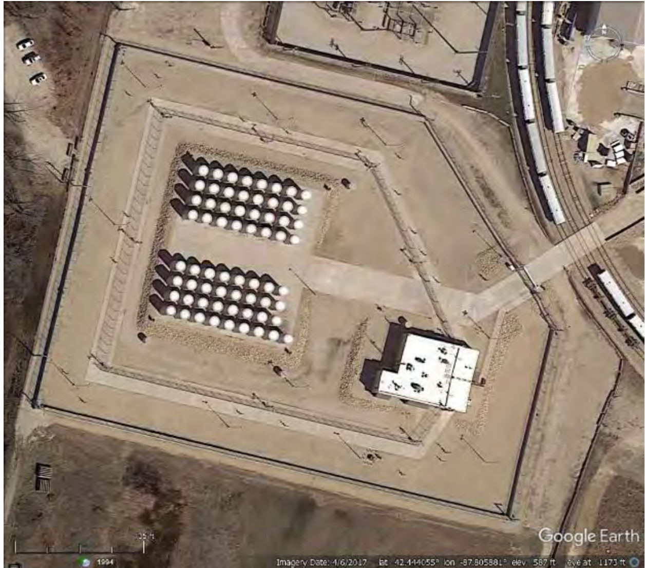
Figure 2-139. Aerial View of Zion Independent Spent Fuel Storage Installation (Google 2017)
