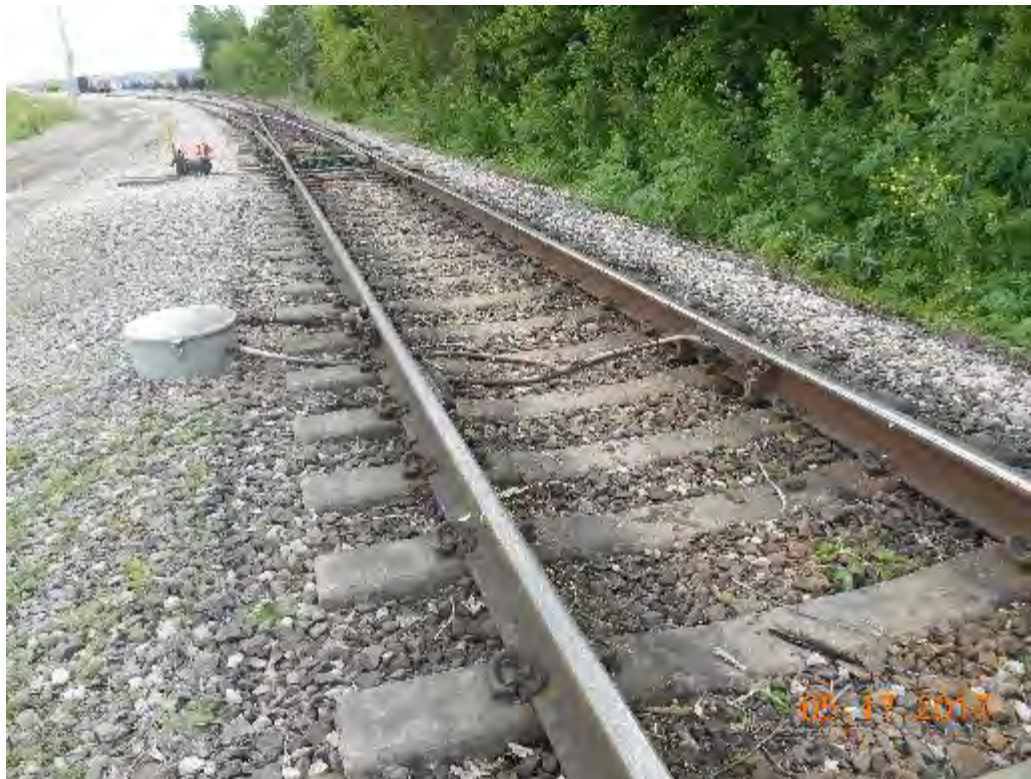
Figure 2-350. Derailer and Greaser on Cargill Industrial Spur (2017)
