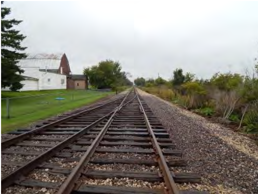
Figure 2-212. Potential Luxemburg Transload Location Further Down Track (Looking West) (2014)
