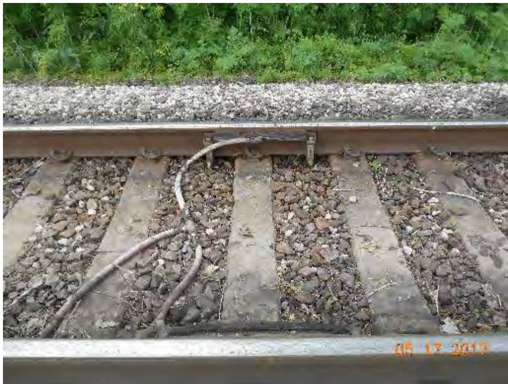
Figure 2-351. Close-up of Greaser Activators on Cargill Industrial Spur (2017)
