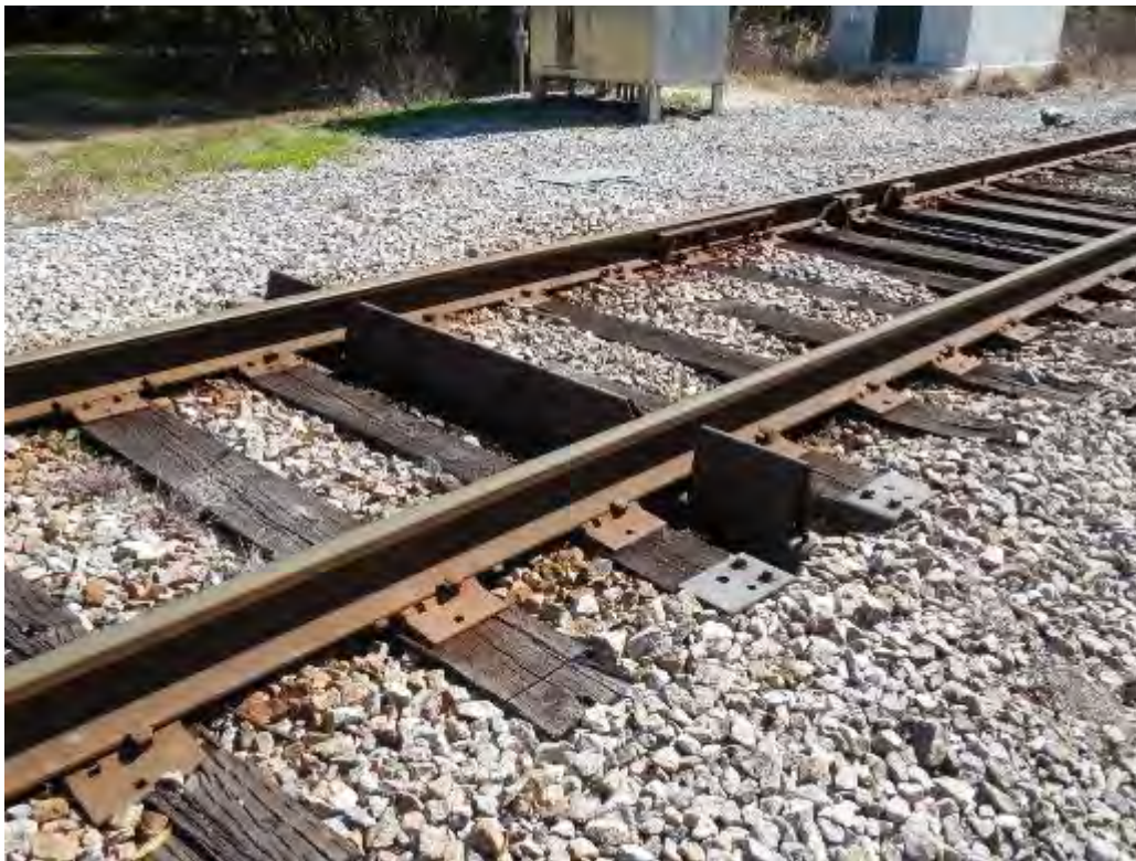
Figure 2-177. Dragging Equipment Detector on Florida Northern Railroad (2015)
