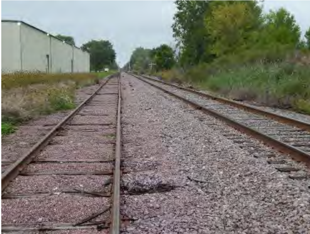
Figure 2-218. Potential Bellevue Transload Location (Looking North) (2014)
