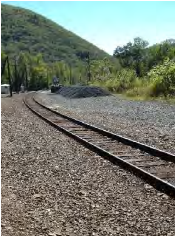
Figure 2-28. Rail Line at East Portal of the Hoosac Tunnel (2012)
