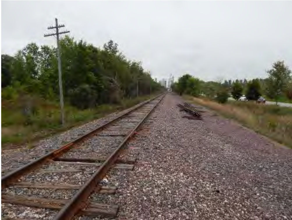
Figure 2-226. Potential Denmark Transload Location (Looking South) (2014)
