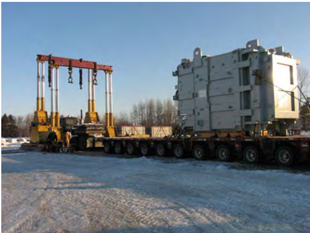
Figure 2-214. Gantry System Used to Transfer Transformers from Railcars to Goldhofer Trailers (2008)
