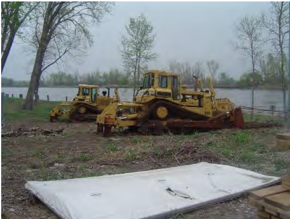
Photo courtesy of Fort Calhoun
