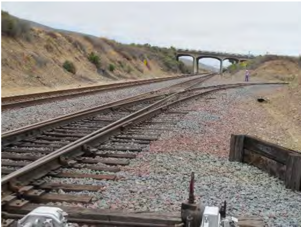
Figure 2-290. Mainline at San Onofre Site (Looking South) (2015)
