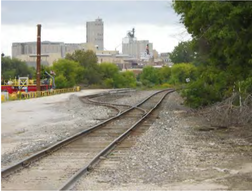
Figure B-37. Red Arrow Siding (2014)
