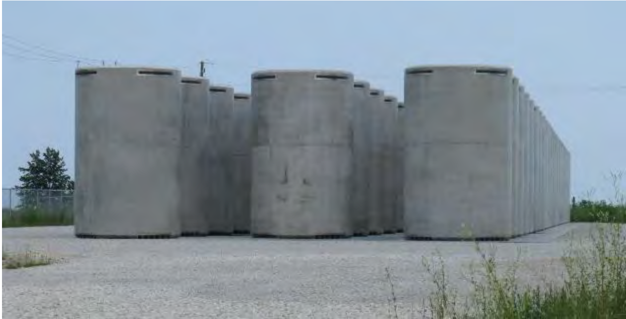
Figure 2-140. Vertical Concrete Storage Casks Staged at Zion (2013)
