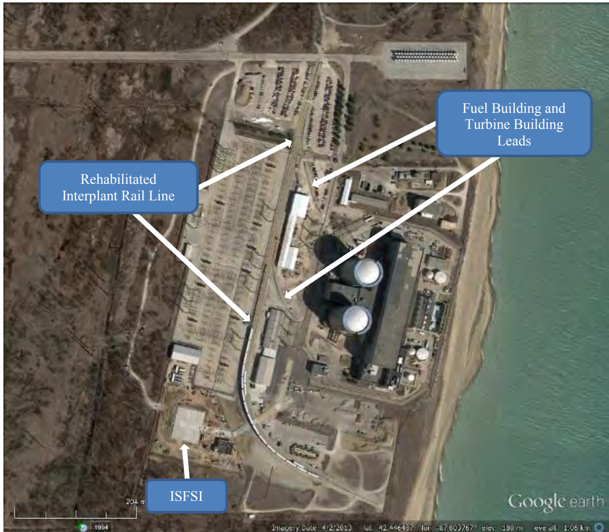
Figure B-21. Satellite view of Zion Site Showing Independent Spent Fuel Storage Installation Pad, the Rehabilitated Interplant Rail Line, and the Leads to the Reactor Containment Building (Google 2017)
