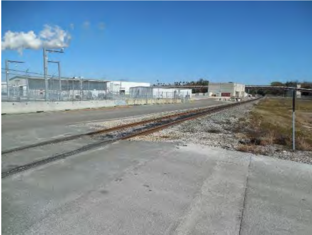
Figure 2-161. Onsite Industrial Rail Spur in Front of the Independent Spent Fuel Storage Installation Site (Looking East) (2015)
