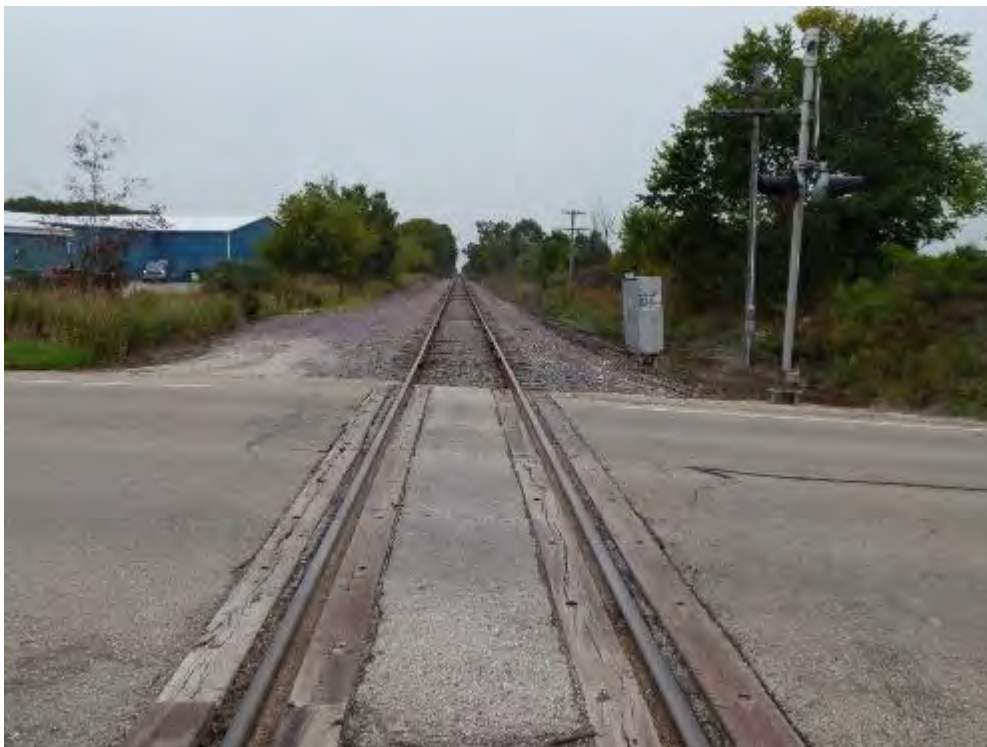
Figure 2-227. Potential Denmark Transload Location (Looking North) (2014)
