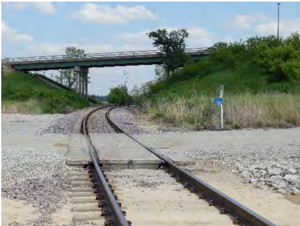
Figure 2-342. Cargill Industrial Spur (Looking Southeast) (2017)
