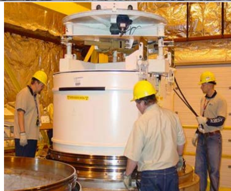
Right: Waste in a Ten Drum Over-pack being loaded into a TRU Pact II.
