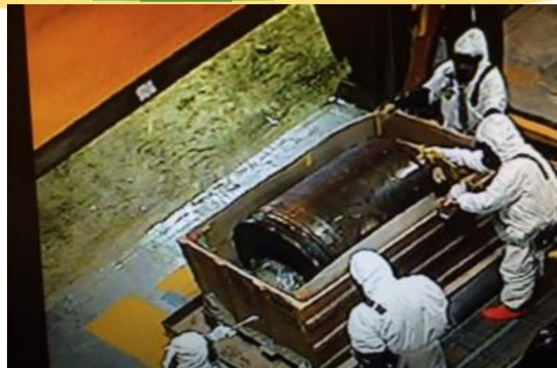
Above: Crews decontaminate the back-up roller for disposal as M/LLW.
