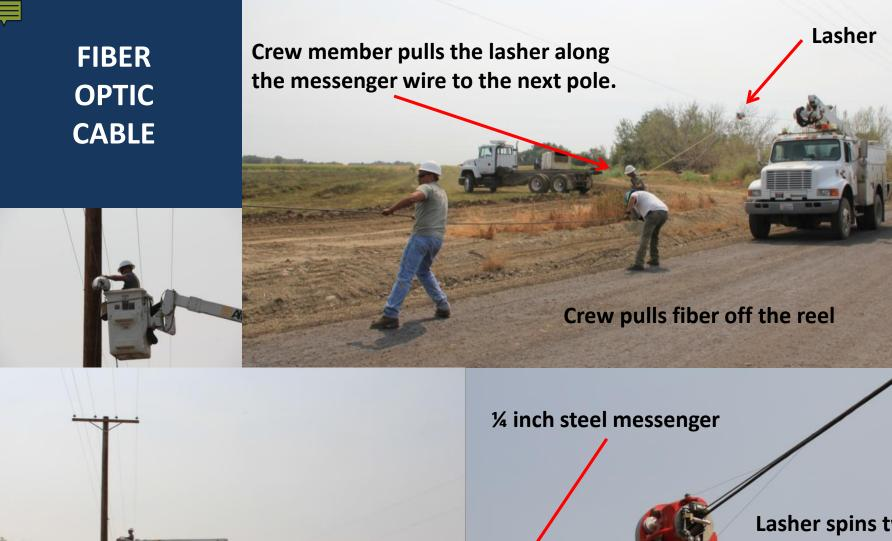
Lasher spins two steel wires around the fiber and messenger wire, which provides the strongest solution.
