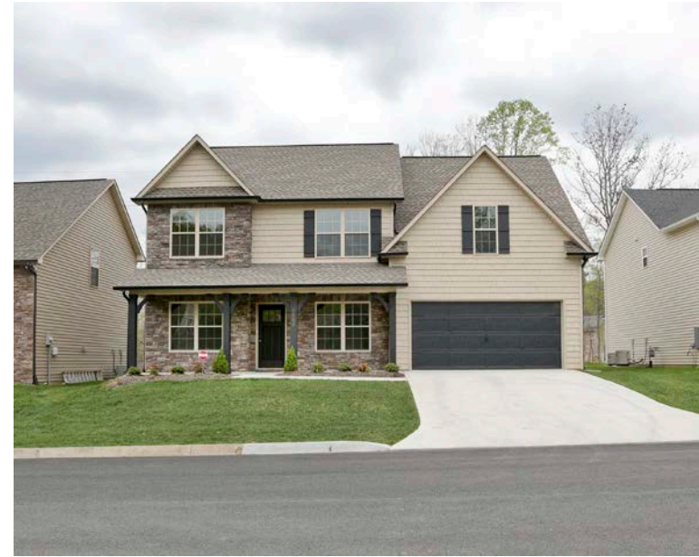
Yarnell Station house, A 2,400 ft 2 house located in Knoxville, TN
