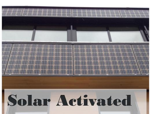
Facades: Cladding systems that capture and store solar energy within the building to create a thermal buffer
