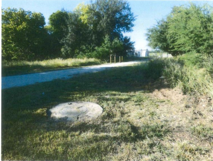
7. View from Avenue F Access Road, at southwest corner of facility site, showing concrete block structure and Quonset hut in background, facing southwest.
