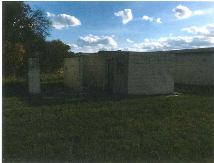
4. View of concrete block structure, facing south.
