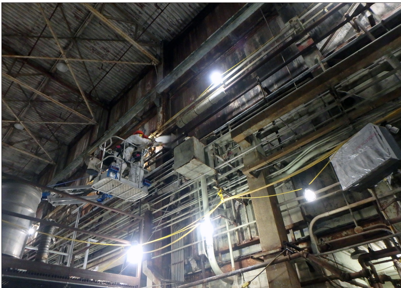
Asbestos abatement in Building 7500
