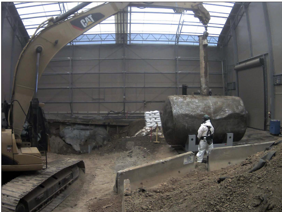
Tank W-1A being removed from the ground
