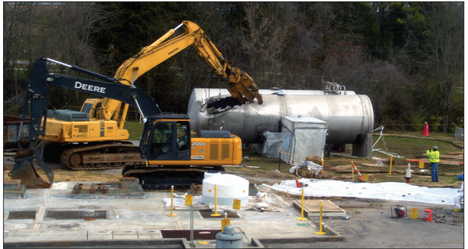
The 3085 tanks were among the non-reactor facilities that were demolished
