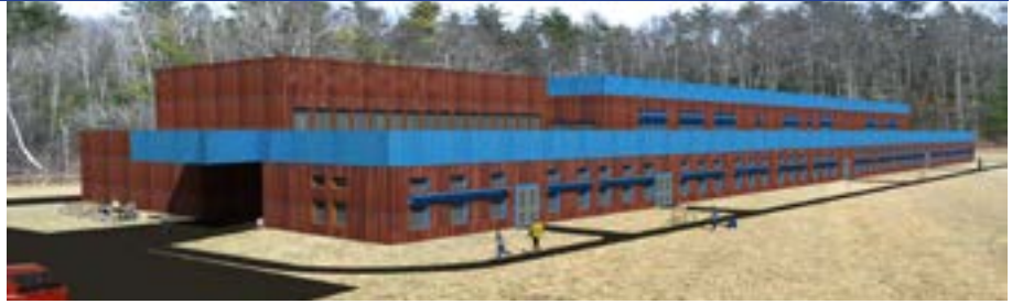
Figure 1. View of the main entrance and southern facade.
