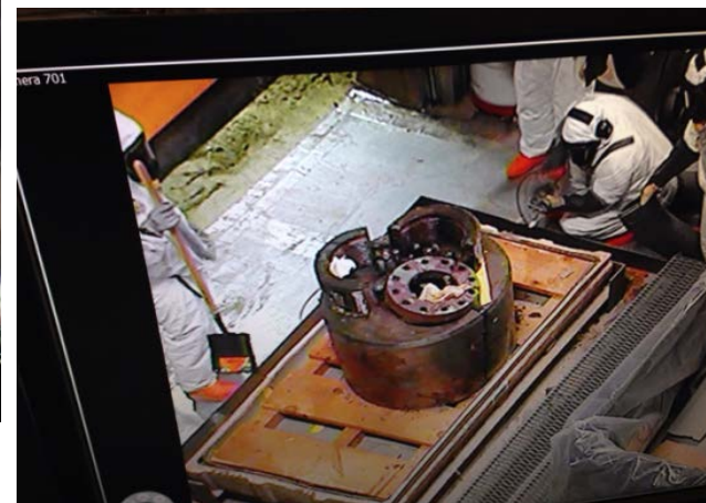
Crews decontaminate the large items for disposal as M/LLW.
