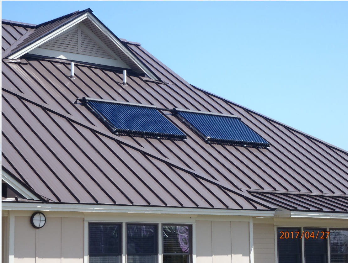
Picture: Passive solar hot water heaters units on south facing roof slope
