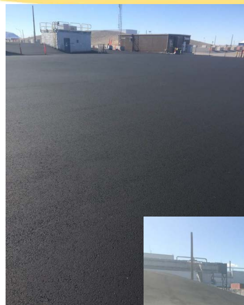
New asphalt and sealcoat over north Tank Farm area
