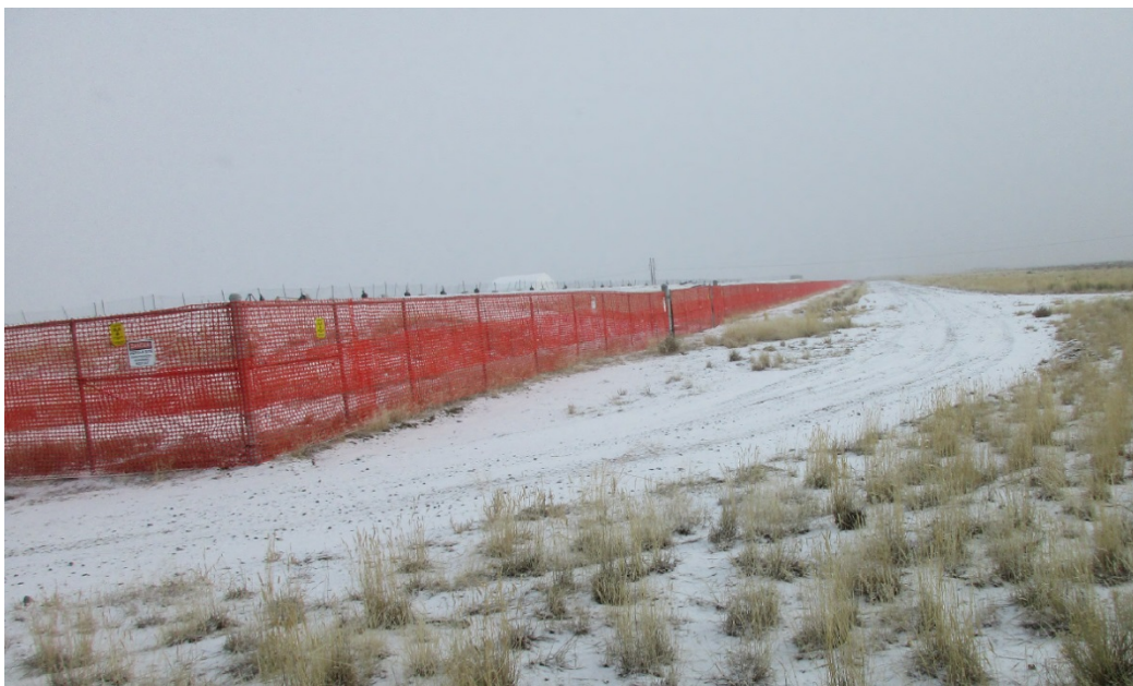
Snow fence installed around ICDF disposal cell to reduce the amount of leachate from melting snow
