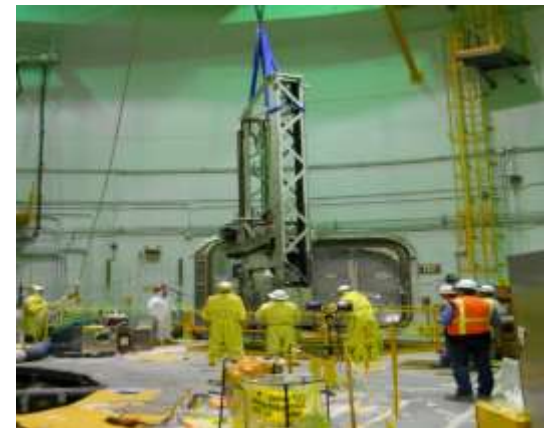
Preparatory actions to grout EBR-II Reactor Basement. View looking into the basement and removal of ancillary equipment
