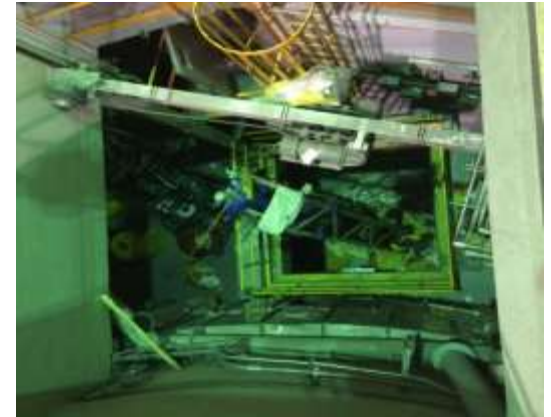
Preparatory actions to grout EBR-II Reactor Basement. View looking into the basement and removal of ancillary equipment
