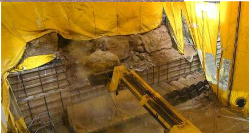
Removal of Soil Fire Break Between Cells 1 & 2
