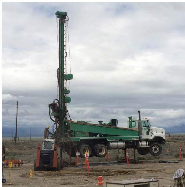
Setting up drill rig for TAN well drilling - May 2015
