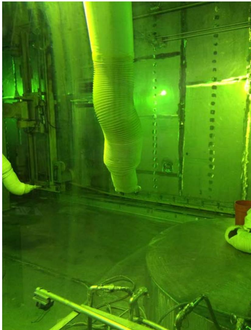
Removing the cell port cover (above the cell) significantly increased ventilation flow through Decontamination Cell 308 and reduced the vacuum in the cell, which maintains contamination confinement
