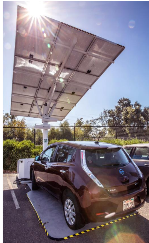
Mobile Solar Level 2 Charger DOE/NNSA Livermore, CA
