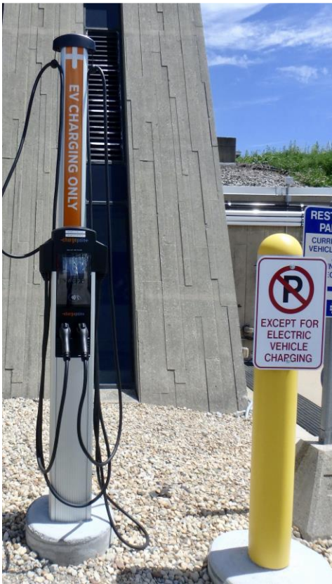
Level 2 Charger DOE/SC Fermilab, IL
