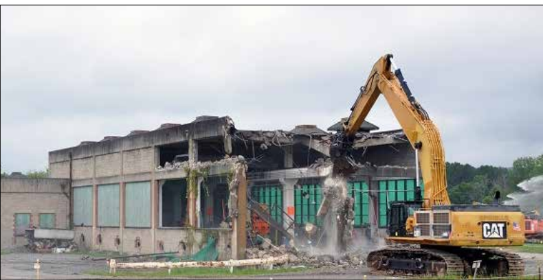
Workers tear down the K-832 Cooling Water Pumphouse.
