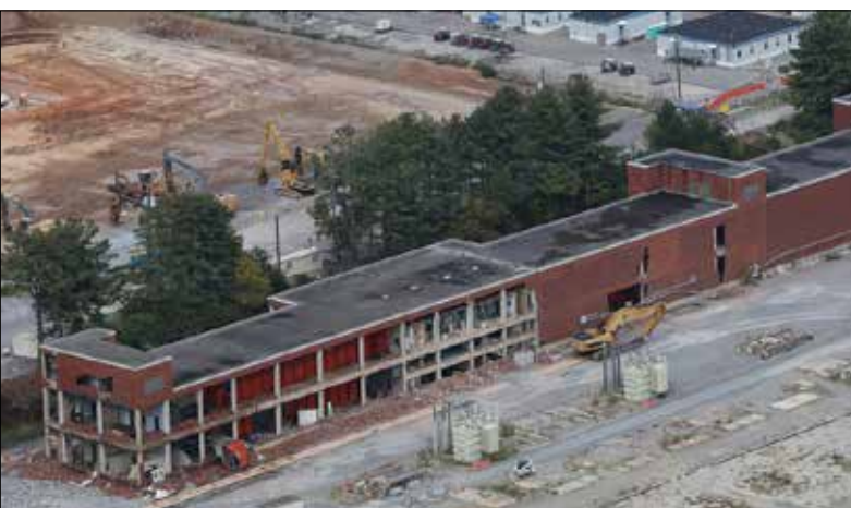
Building K-731 during demolition.
