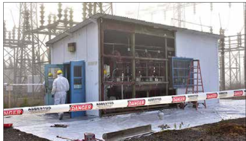
CTI workers clean up the K-732 switchyard
