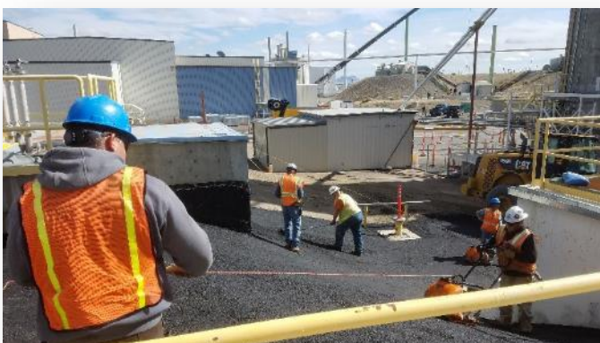
Workers paved a large section of the tank farm at the Idaho Nuclear Technology and Engineering Center to protect the underlying Snake River Plain Aquifer
