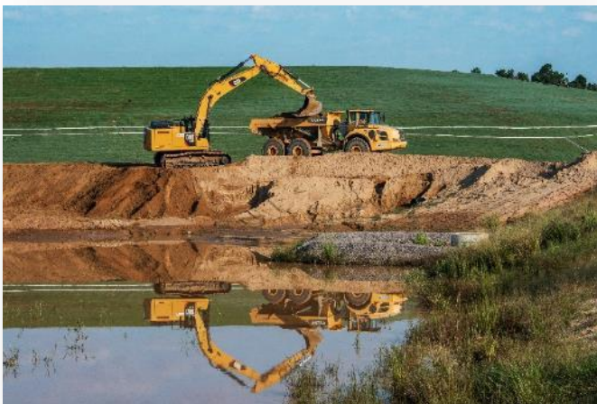
The D Ash Remediation project is 68 percent complete.
