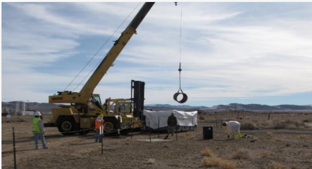
Contaminated debris removed from an Area 3 Plutonium Dispersion Site is placed in a waste package for disposal at the Area 5 Radioactive Waste Management Complex
