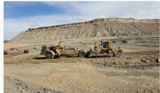
Above: The new water wagon sprays water for dust suppression at the Moab site. Below: A scraper and a bulldozer work in tandem to excavate Phase 3b of the Crescent Junction disposal cell.
