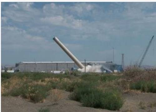
Demolition of the ventilation stack at the Plutonium Finishing Plant.
