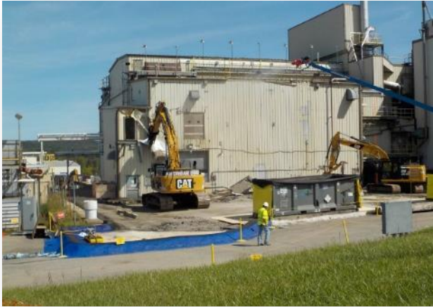
"First Bite" in Vit Facility demolition. Sept 11, 2017
