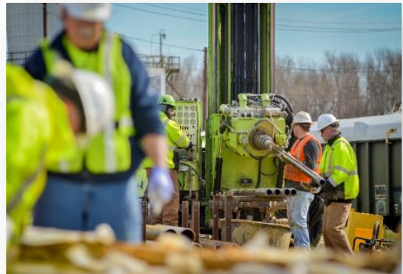
Drill operators attach a section of pipe to continue drilling wells for Paducah’s Northeast pump-and-treat system optimization.
