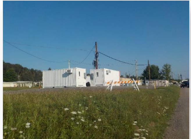
New data center installed to house telephone and computer server equipment being removed from the vacant Administration Building
