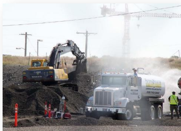
Workers place soil in the area of the partial collapse on PUREX Tunnel 1, immediately after the breach is discovered.
