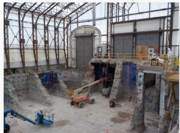
With tanks removed, the building is ready for open air demolition
