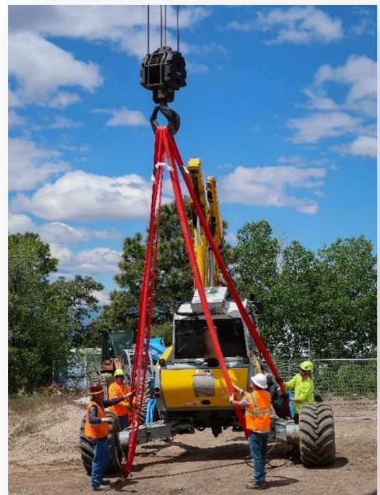
After carefully securing a spider excavator to a crane, the excavator was lowered to the cleanup site on the side of a canyon
