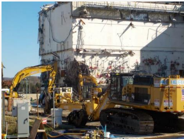
First piece of Vit Cell demolished. Nov 8, 2017
