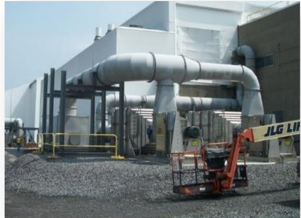
G2 building enclosure
