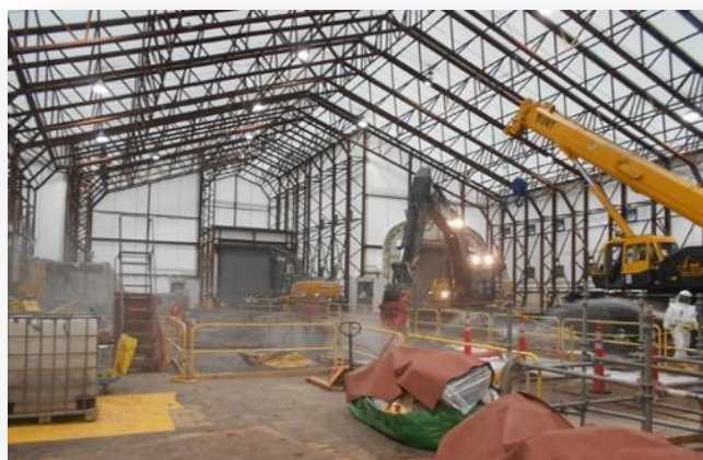
Building H2 beneath the tent enclosure at the Separations Process Research Unit
