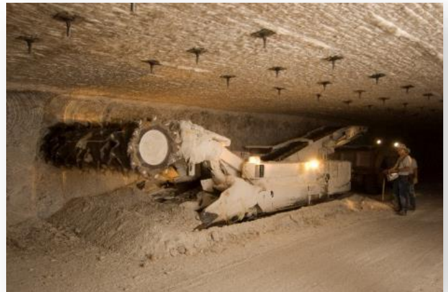
This continuous miner, located in the underground at WIPP, cuts the salt and creates space for the emplacement of transuranic waste. WIPP was mined into a 2,000-ft. salt bed which is more than 25-million years old.
