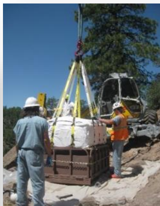
Workers sealed bags of contaminated soil prior to transportation and shipment to an offsite disposal facility.
