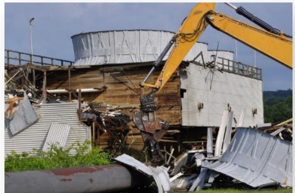
Workers tear down the K-832 Cooling Water Pumphouse.
