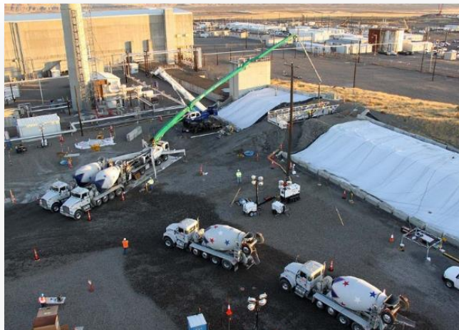
An aerial view of workers placing grout in PUREX Tunnel 1.
