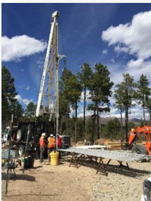
A groundwater sampling system was installed at the monitoring well R-68.
