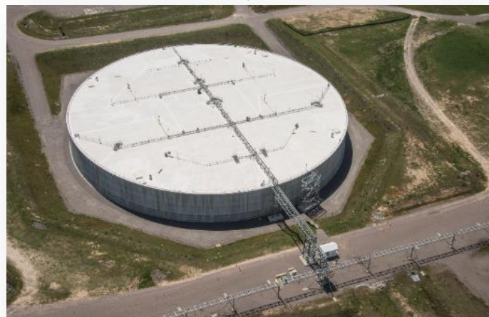
The Savannah River Site's first mega-volume Saltstone Disposal Unit sits on 2-1/2 acres and will hold about 33 million gallons of saltstone. Construction was completed in 2017 under budget and ahead of schedule.
