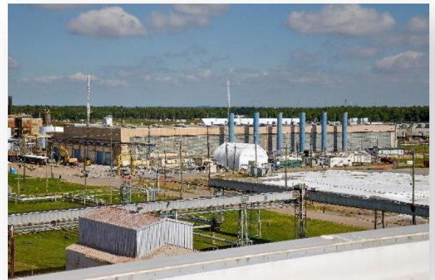
Northwest view of the Paducah C-400 Cleaning Building
