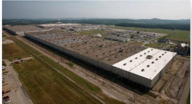
Extensive characterization occurred in Portsmouth X-326 Process Building in 2017, work that is instrumental in achieving Cold & Dark status.
