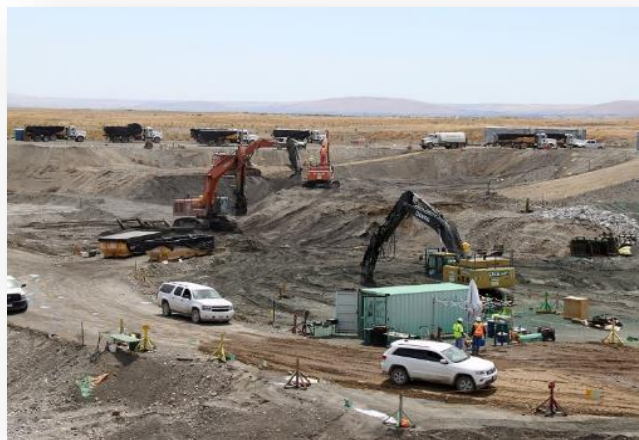
Workers remove contaminated soil and debris from the 618-10 Burial Ground.
