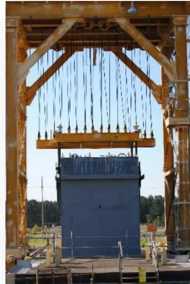
Melter 2, inside its storage box, was lowered by crane into an underground storage facility for safe, interim storage
