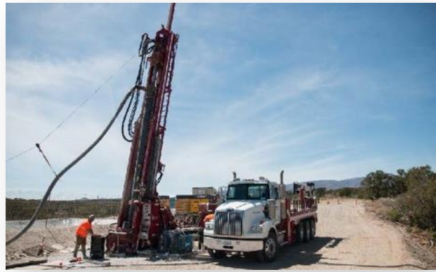
Angled drilling, at wells such as at the CrIN-4, enabled the project team to reach objectives and avoid culturally sensitive sites.
