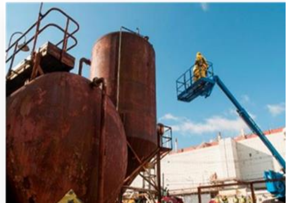
Crews work to clean and remove the old column exchange (COLEX) equipment at Alpha 4
