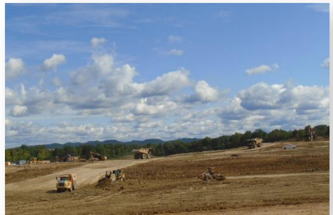
Progress continued on the construction of Portsmouth's On-Site Waste Disposal Facility in 2017.
