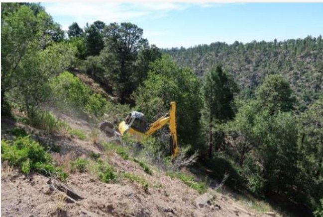
A spider excavator crawled along the side of the canyon to the second cleanup site.
