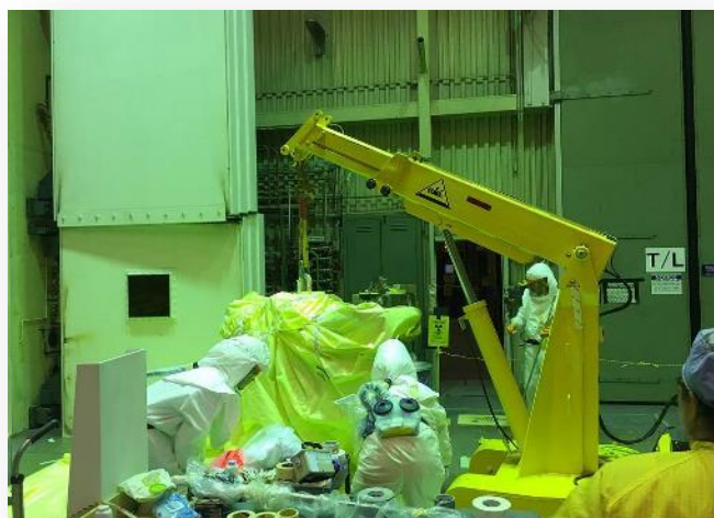
Workers remove a large hose reel from an airlock in the 324 Building.
