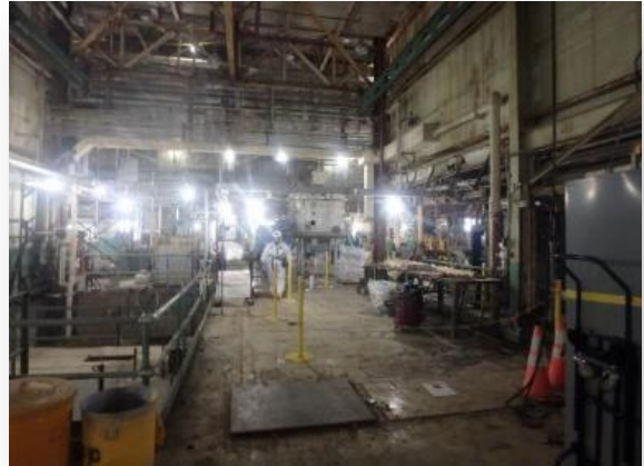
Workers remove asbestos from Oak Ridge National Laboratory Building 7500
