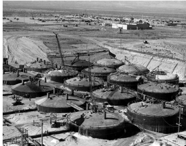
*The Hanford Site's single-shell underground storage tank system was built from 1943–1964. The Draft EIS analyzes the potential environmental impacts of closure of Hanford's 149 single-shell tanks.*
