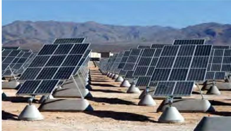
*This 14-megawatt single axis, flat panel photovoltaic cell system is located at Nellis Air Force Base, Nevada. More than 72,000 solar panels occupy 140 acres – the largest solar photovoltaic system in North America.*
