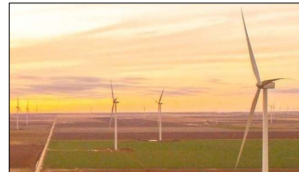
Fort Hood, Texas: 65 MW AC Hybrid Wind & Solar Projects; Expected to provide $100 million in cost avoidance over the term of the 30-year contract
