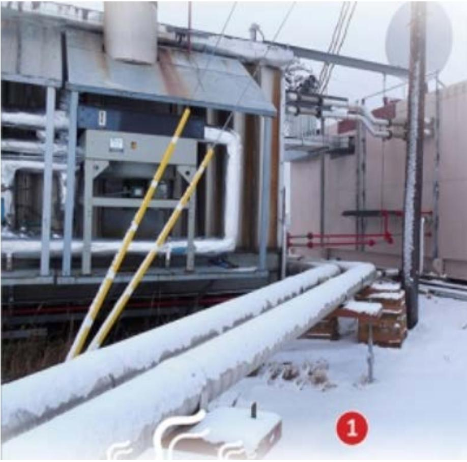
1 AVEC Radiator manifold and heat recovery pipelines
