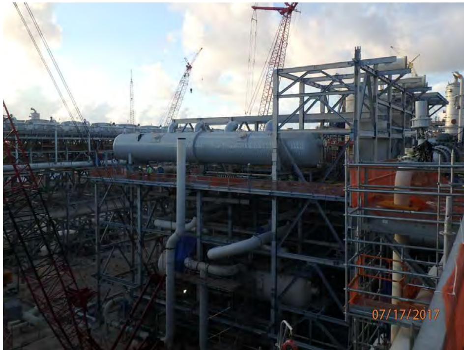
Train 1 – Setting Propane-Methane / Ethylene Feed chiller
