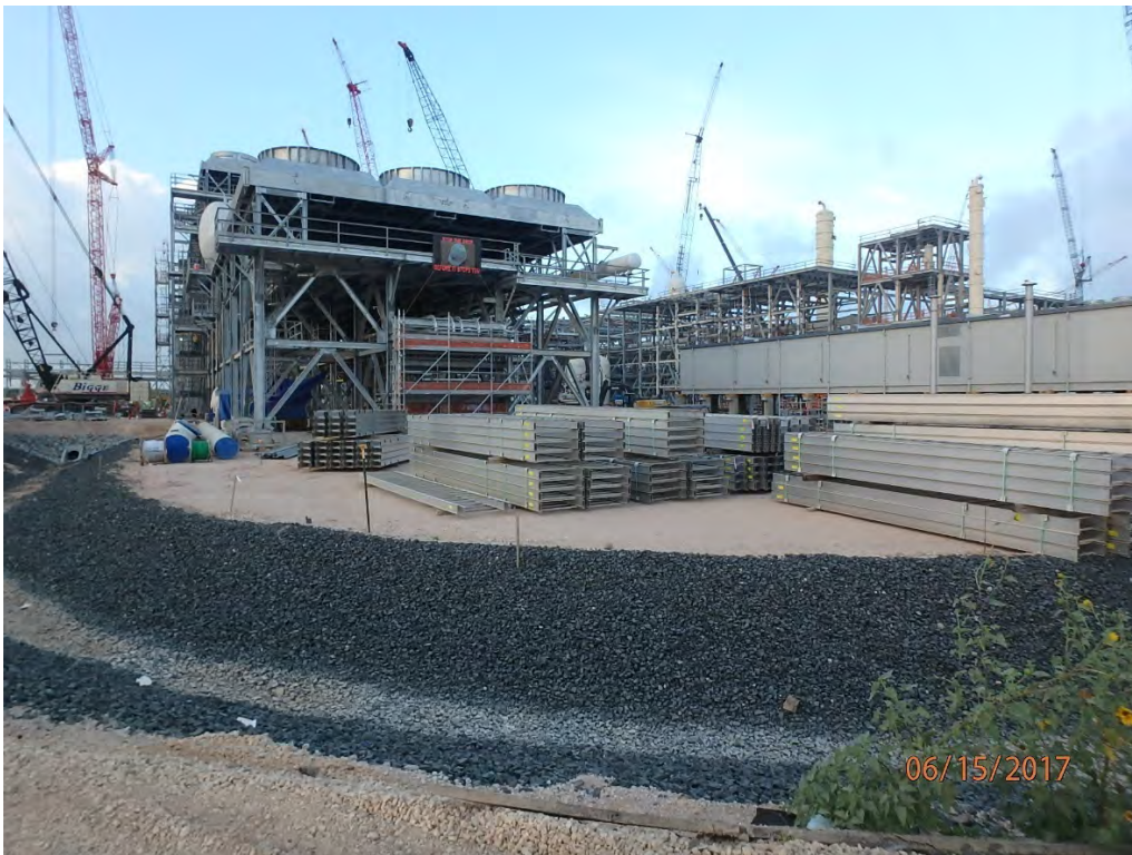
Train 2 – Cable Tray Staging In Preparation for Installation
