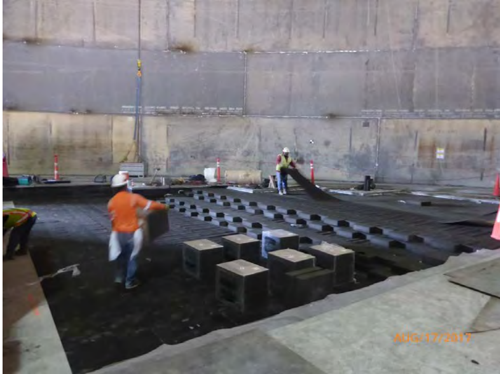
LNG Tank C – Stage 2 Insulation Foam Glass Block
