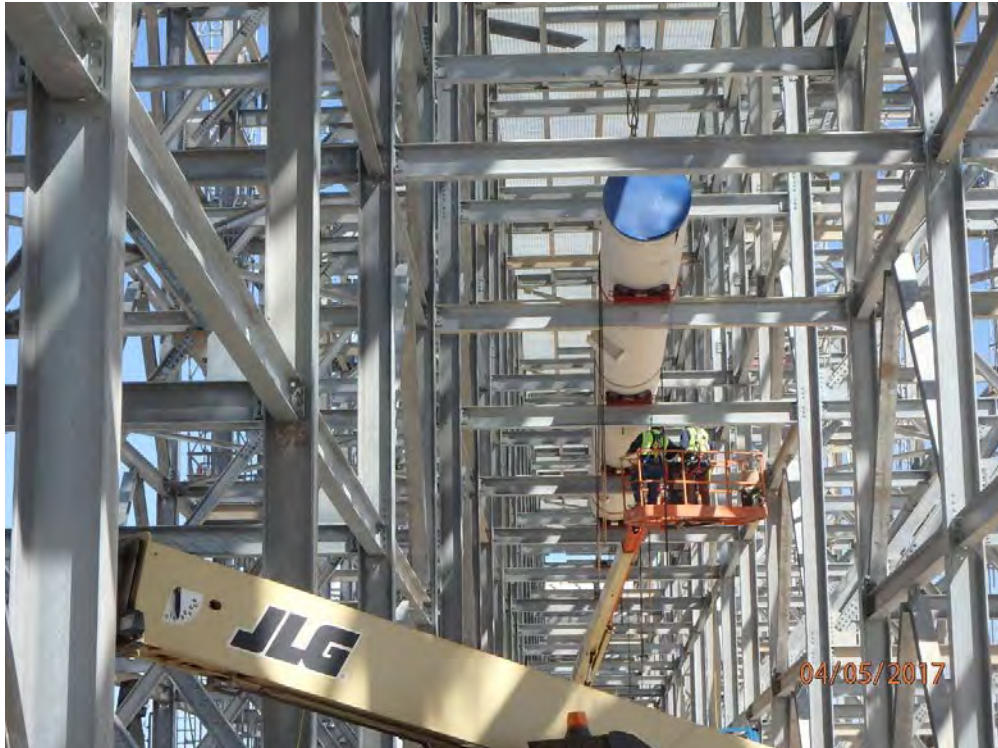
Train 2 – Propane Condenser Pipe Installation
