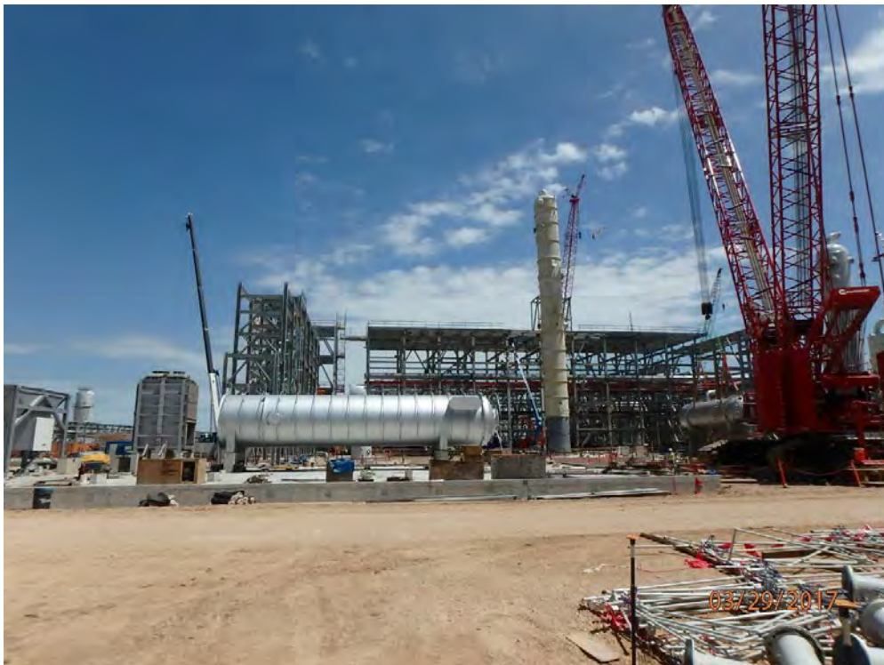
Train 2 – Thermal Oxidizer Installation
