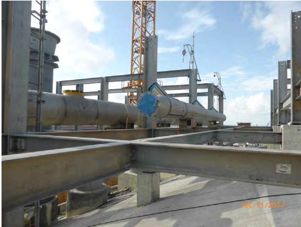
LNG Tank C – Main Pump Platform and Piping Installation
