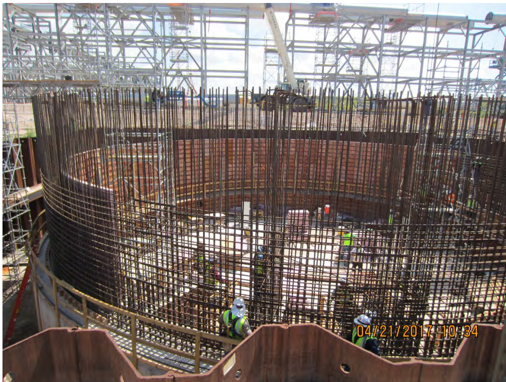
OSBL – Sump Wall Rebar Installation
