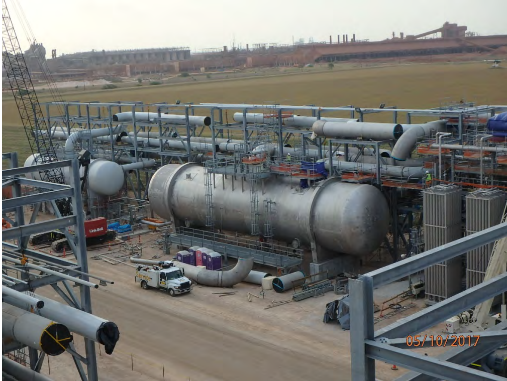
OSBL – Flare Knockout Drum Pipe Installation
