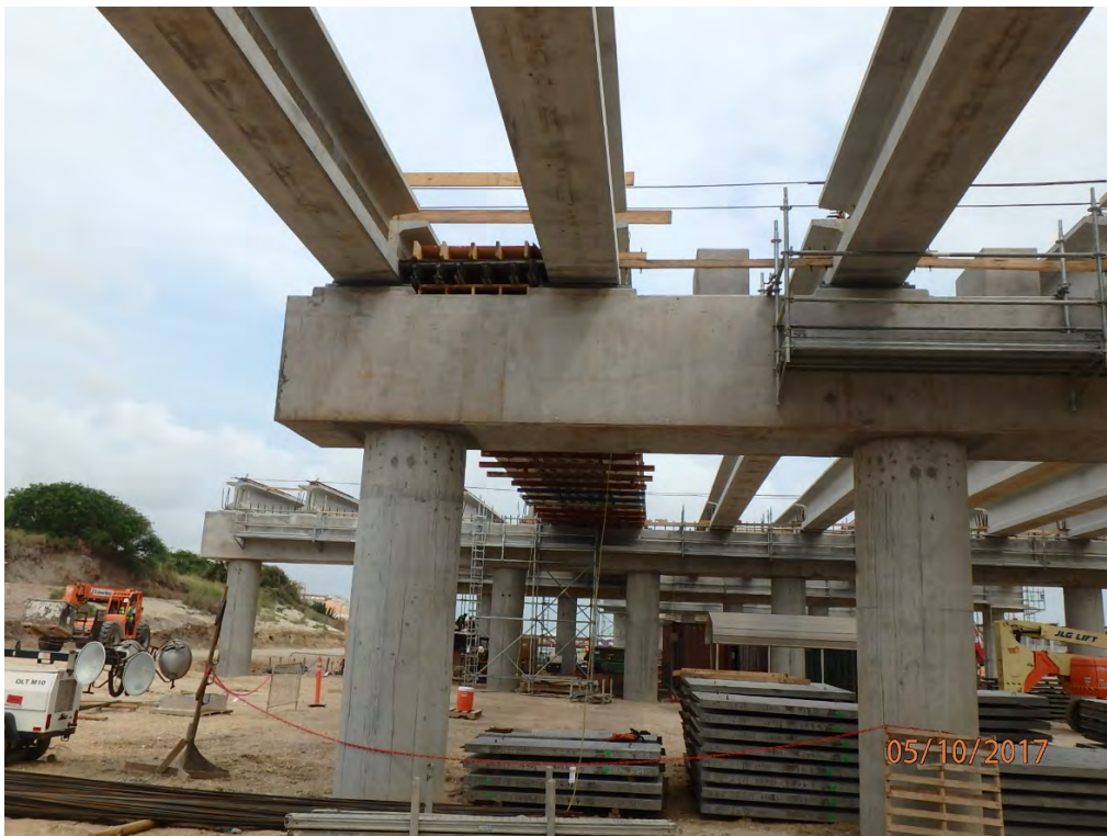
OSBL – East Jetty Diaphragm Formwork Installation
