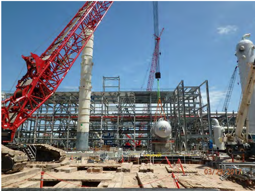
Train 2 – Setting Solvent Flash Drum
