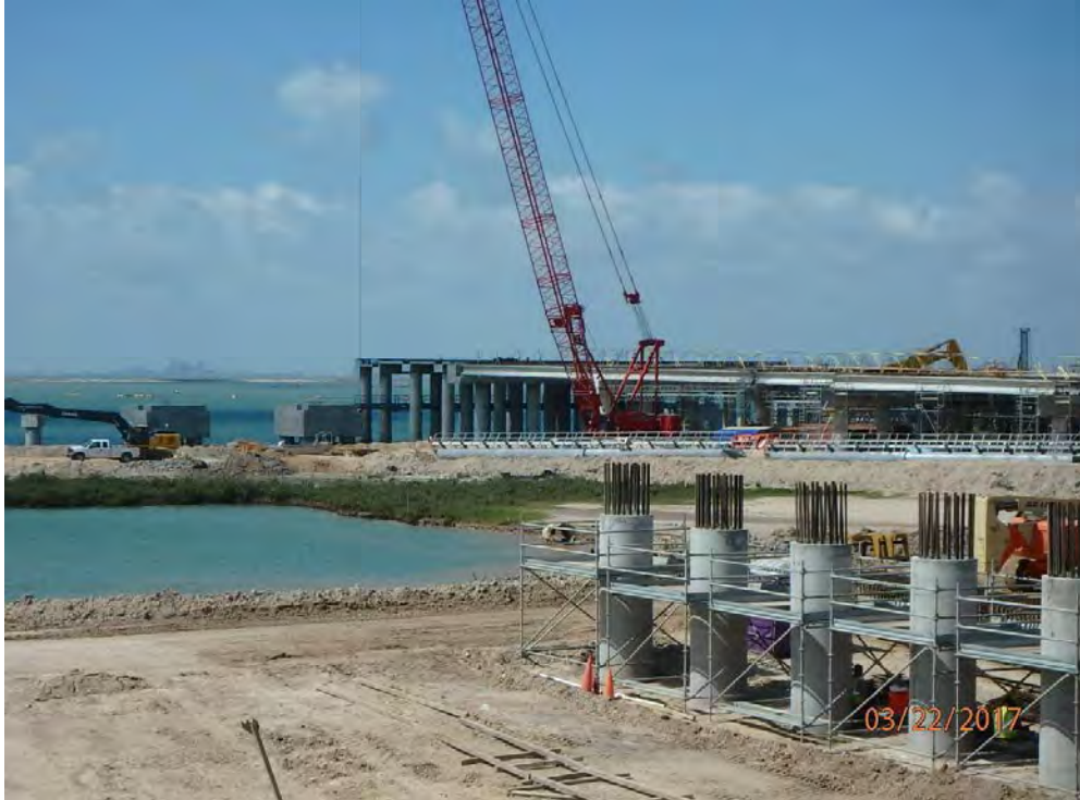
OSBL – East Jetty Columns Installation
