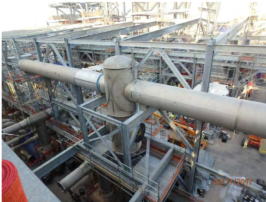
Train 1 – Setting Ethylene Mixing Tee
