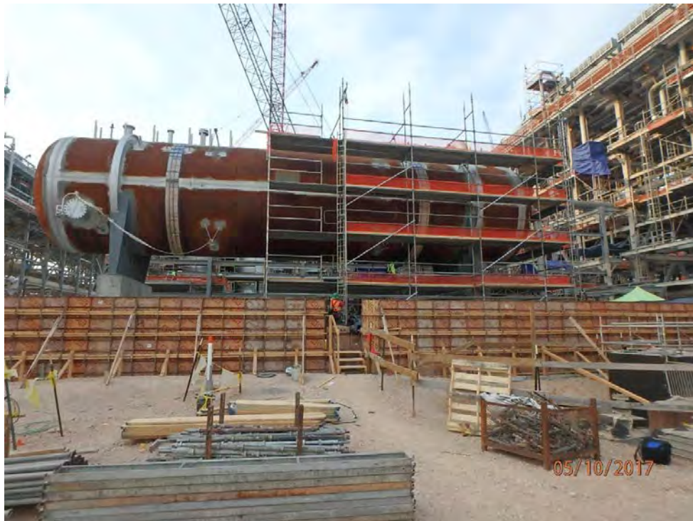
Train 1 – Hot Oil Drum Mechanical Insulation
