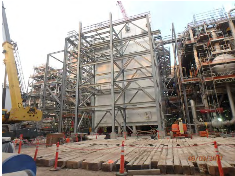
Train 1 – Cold Box Steel Installation
