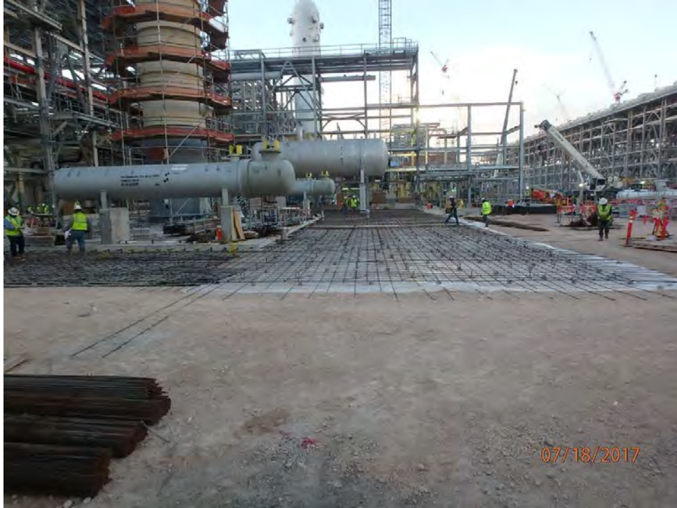
Train 2 – Amine Regen and Acid Gas Removal Area Paving
