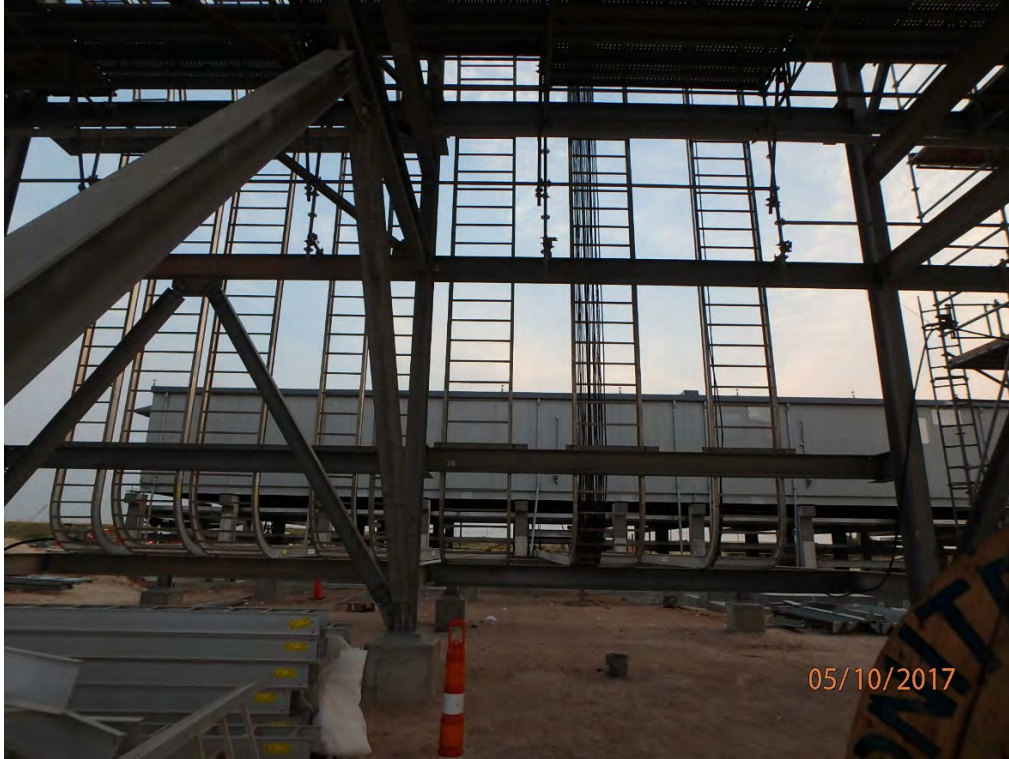
OSBL – Cable Tray Waterfall Installation
