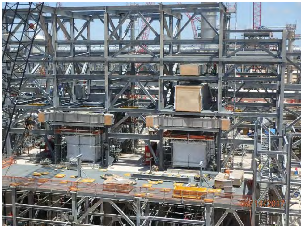
Train 2 – Turbine Ductwork Installation
