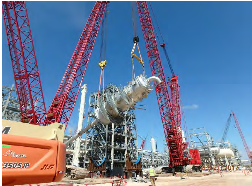
Train 2 – Setting Heavies Removal Column
