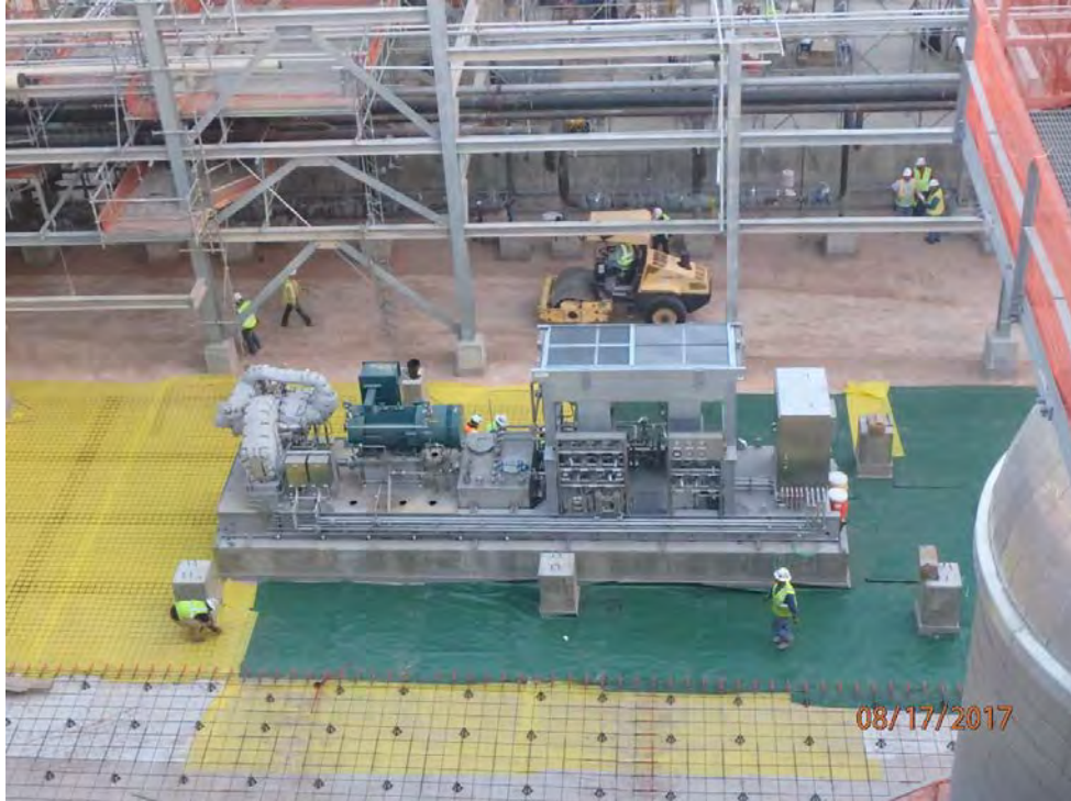
Train 1 – Regen Gas Compressor Setting
