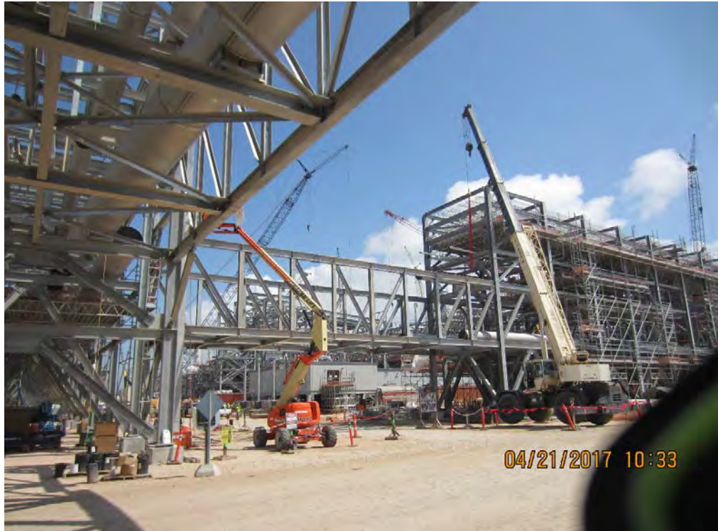
OSBL – Alamo Road Bridge Installation
