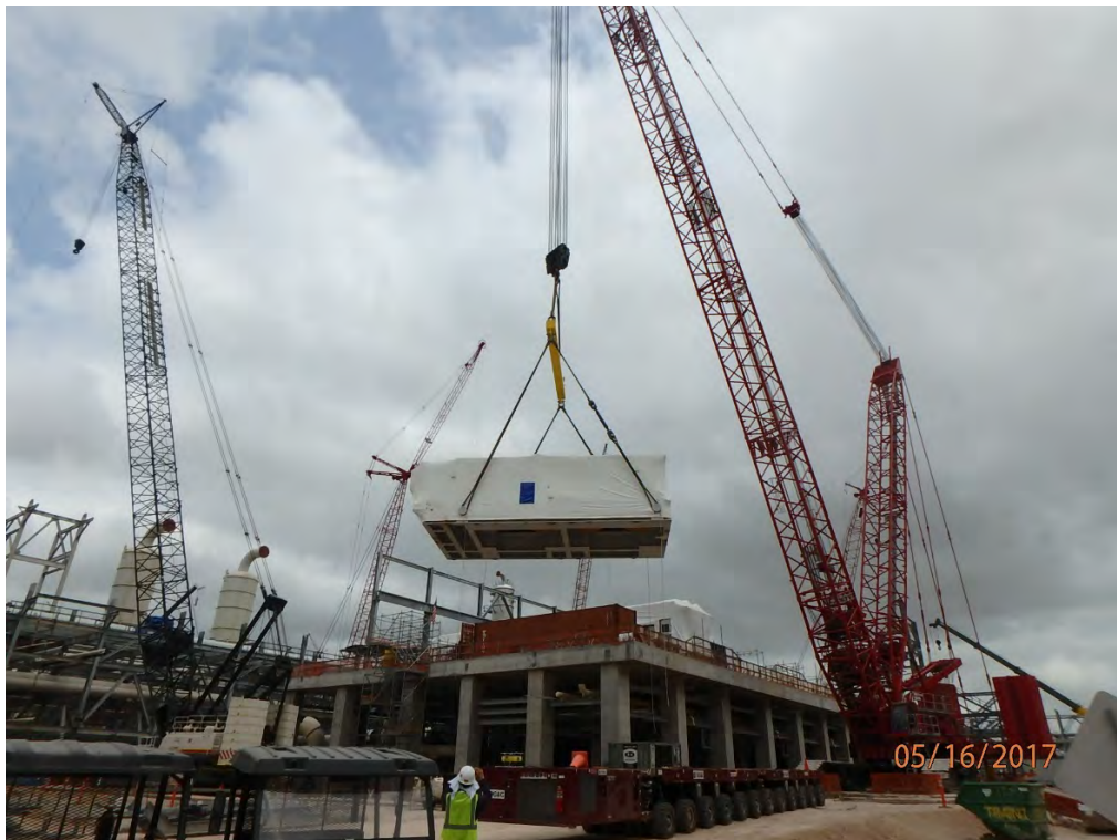
Train 2 – Compressors Setting
