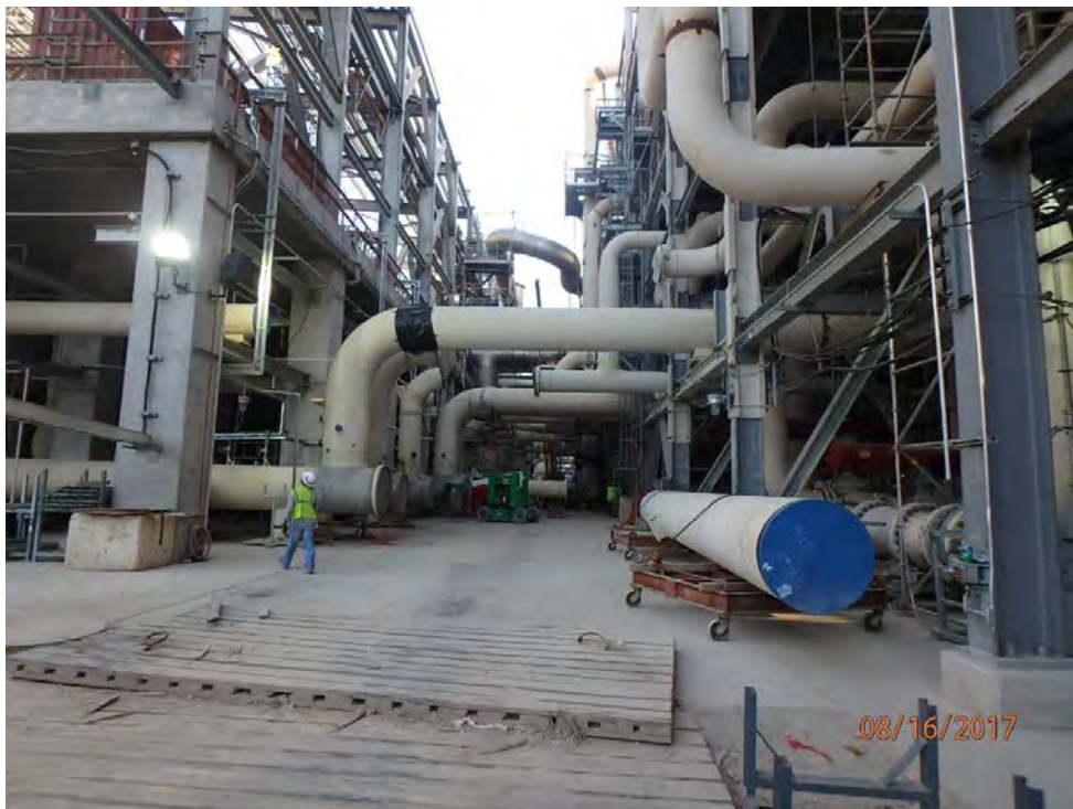
Train 1 – 131A01 Alleyway Pipe Installation
