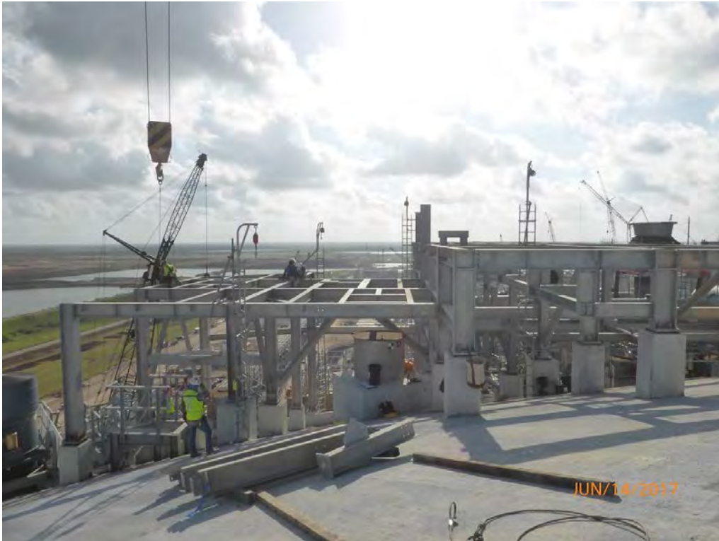
LNG Tank A – Main Pump Platform Installation
