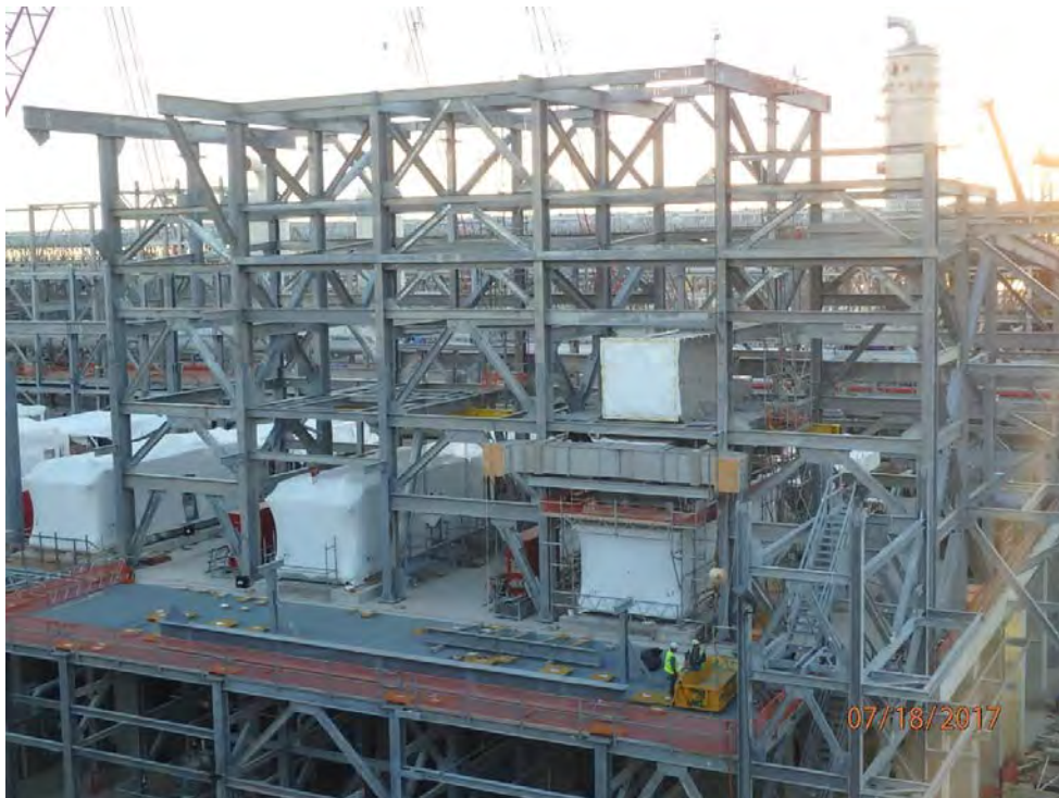
Train 2 – Compressor Area Steel Erection
