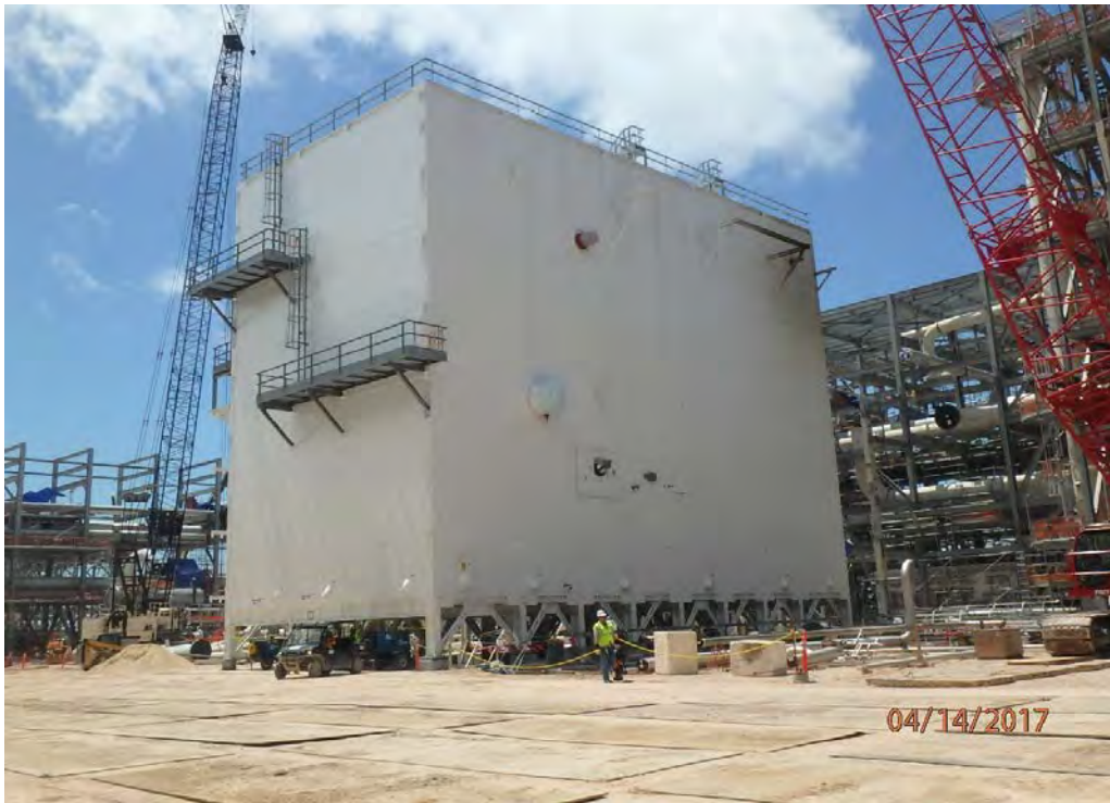
Train 1 – Methane Cold Box on Foundation
