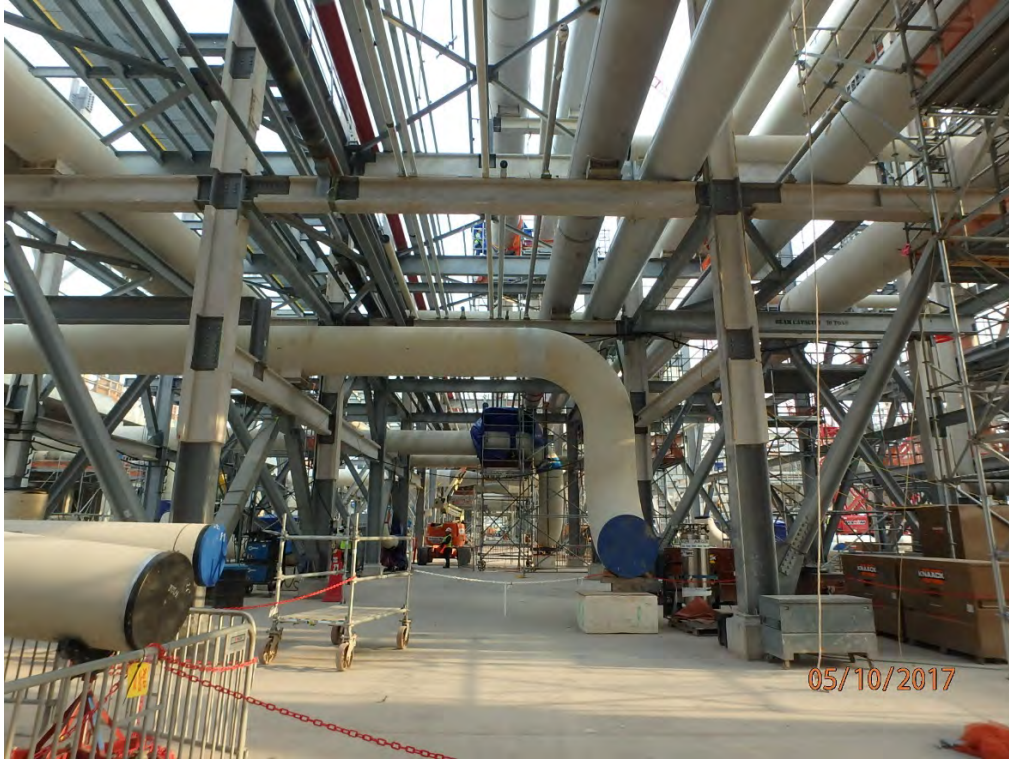
Train 2 – Cryo Rack Pipe Installation
