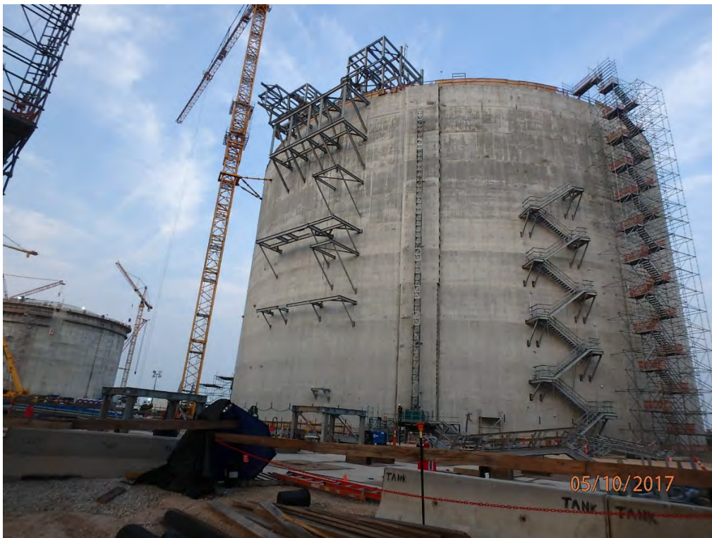
LNG Tank A – Waterfall Support Steel Installation
