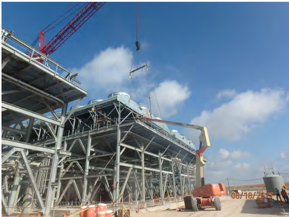
OSBL – Inlet Air Chilling Area Fin Fans Setting
