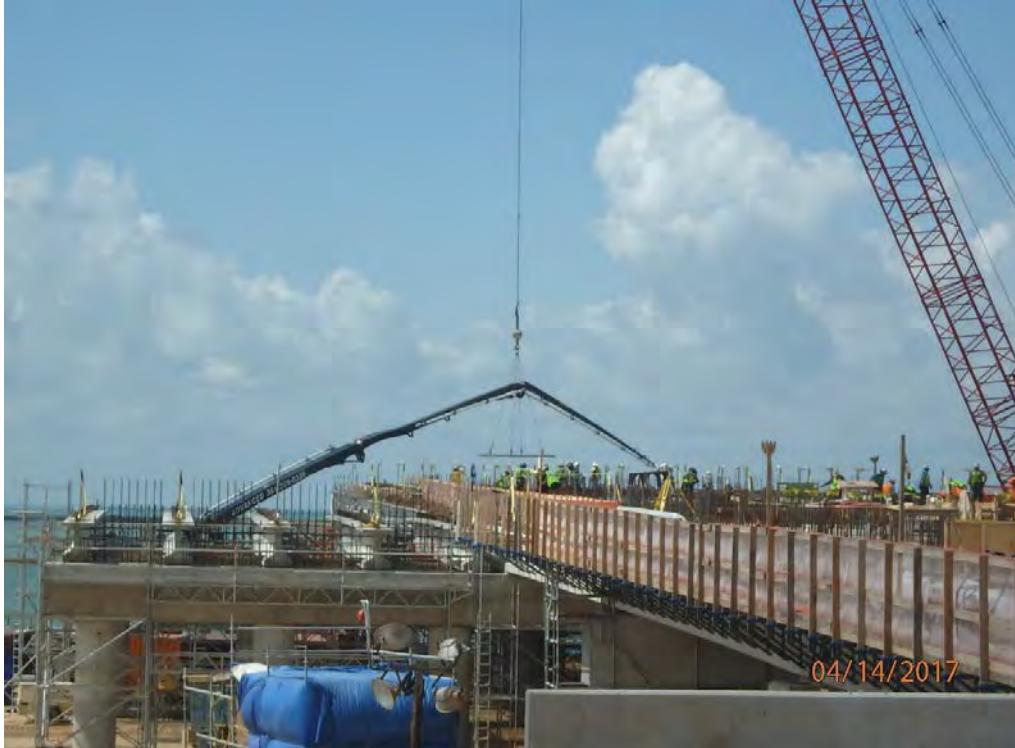
OSBL – West Jetty Concrete Placement
