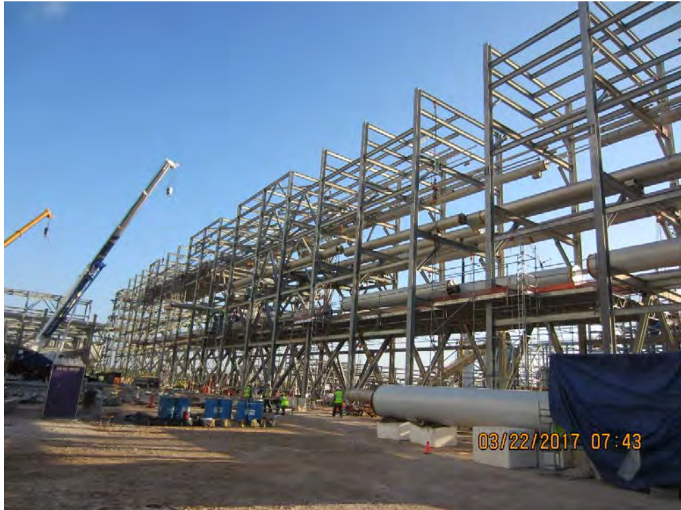
OSBL – AG Pipe Installation
