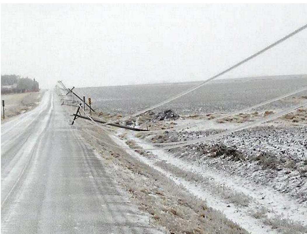
Figure 9.1.15-4: Ice Accumulation and Downed Power Lines South of Luverne, MN (April 10, 2013)
