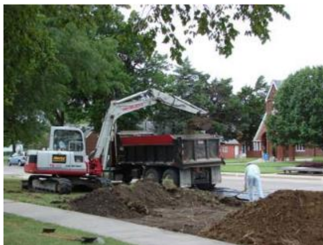
Figure 7.1.15-3: Removal of Contaminated Soil from a Schoolyard in Iola
