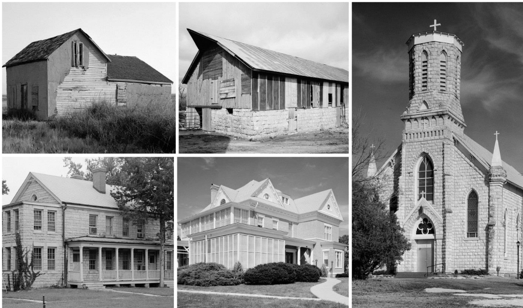
Top Left – Alexander G. Vanduvall House (Nicodemus, KS) – (Historic American Buildings Survey, 1933a) Top Middle – Kandt-Domann Farmstead Barn (Hope, KS) – (Historic American Buildings Survey, 1933b) Bottom Left – Fort Riley, Building Number 174 (Riley, KS) – (Historic American Buildings Survey, 1933c) Bottom Middle – Fort Leavenworth (Leavenworth, KS) – (Historic American Buildings Survey, 1933d) Right – Saint Catherine's Church (Catharine, KS) – (Historic American Buildings Survey, 1933e)
